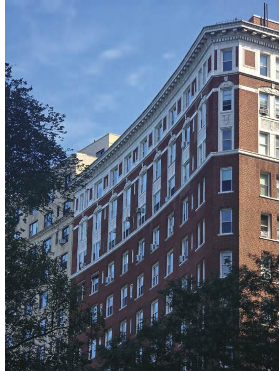
WEST FACADE PHOTO - OVERALL
