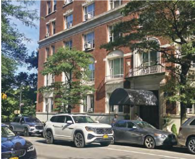
SOUTH FRONT FACADE - CURRENT PHOTO
