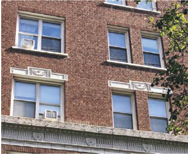
SOUTH FRONT FACADE WINDOW - CURRENT PHOTO
