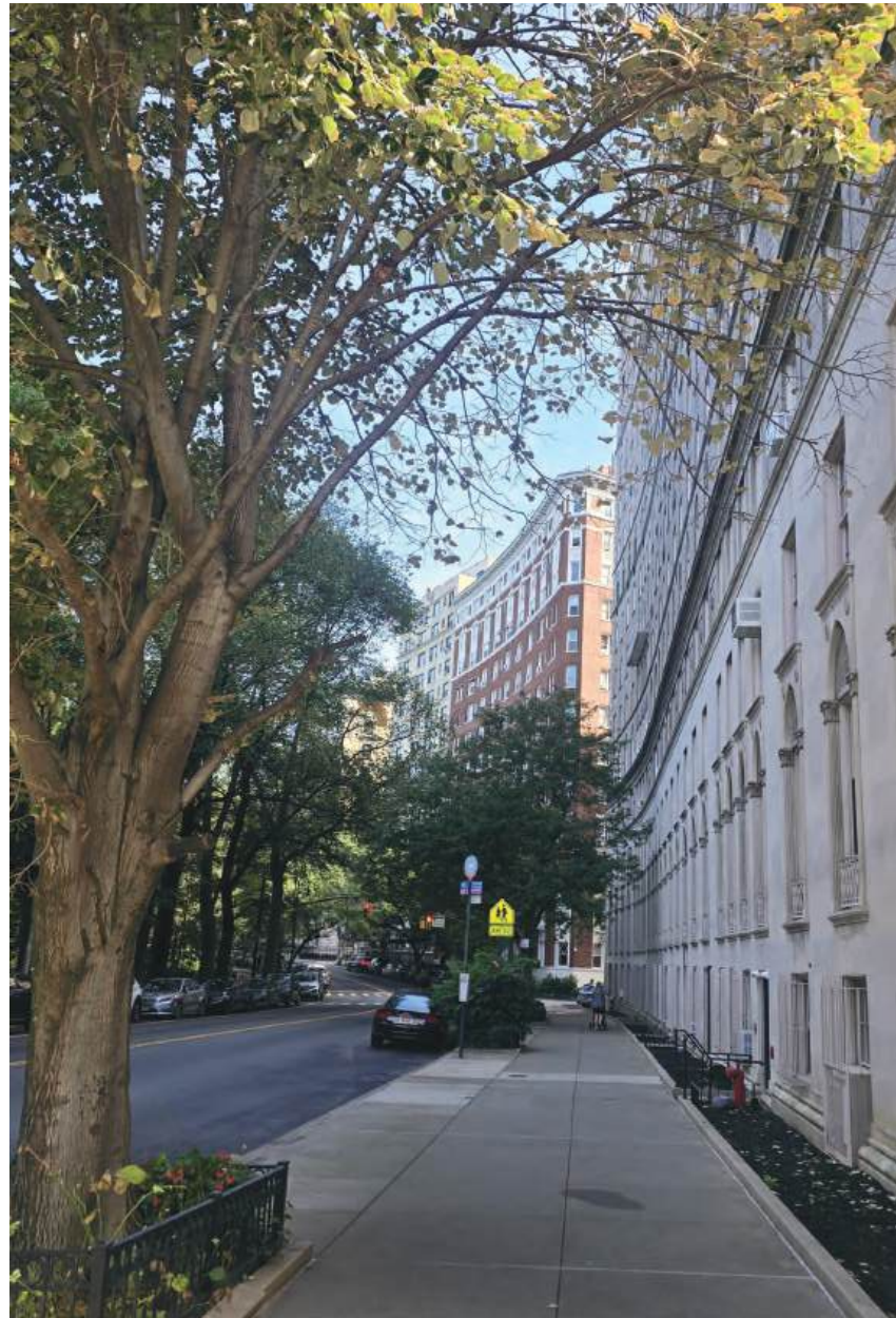
SOUTHWEST CORNER FACADE PHOTO - CURRENT
