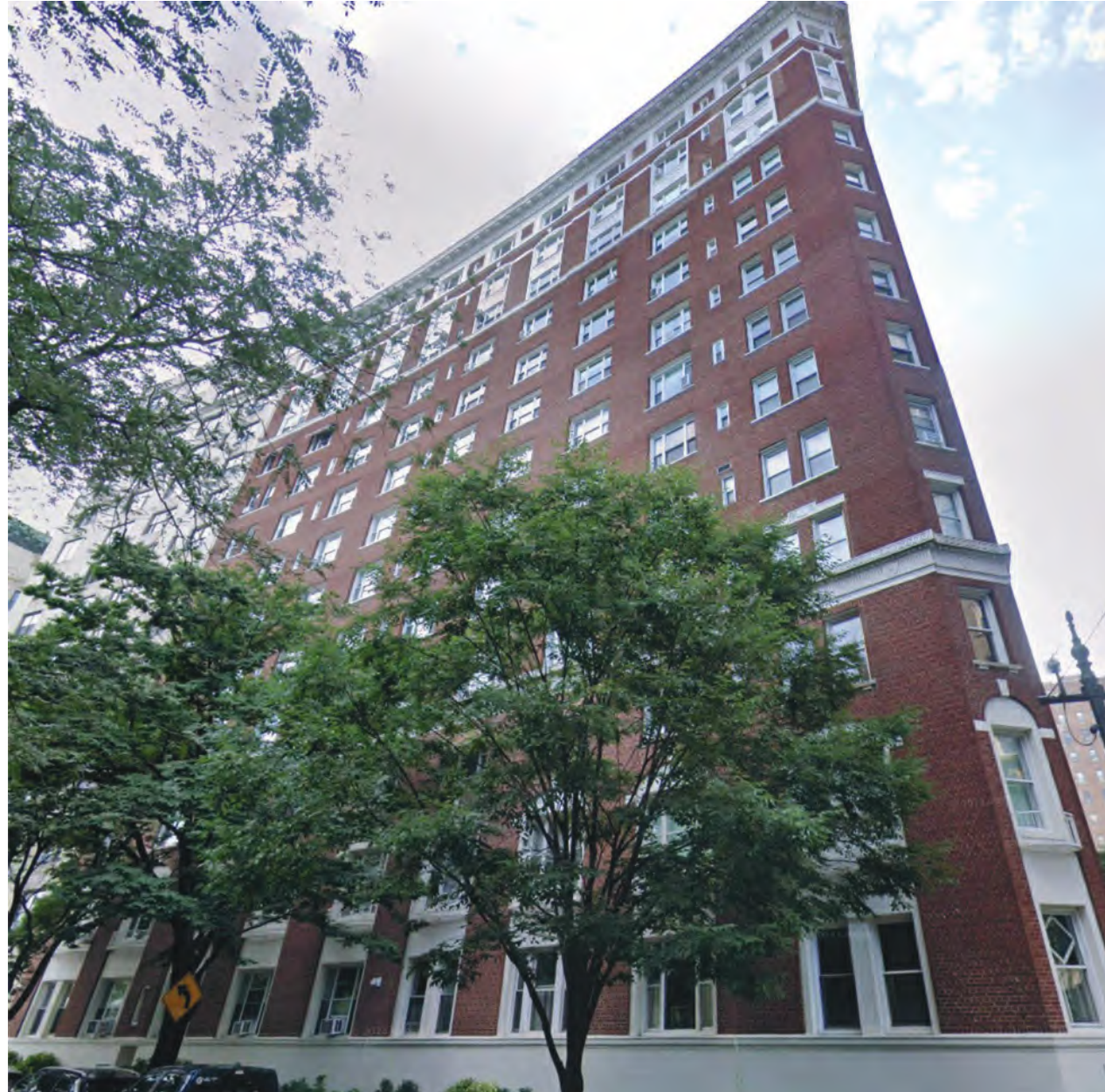
WEST FACADE PHOTO - OVERALL
