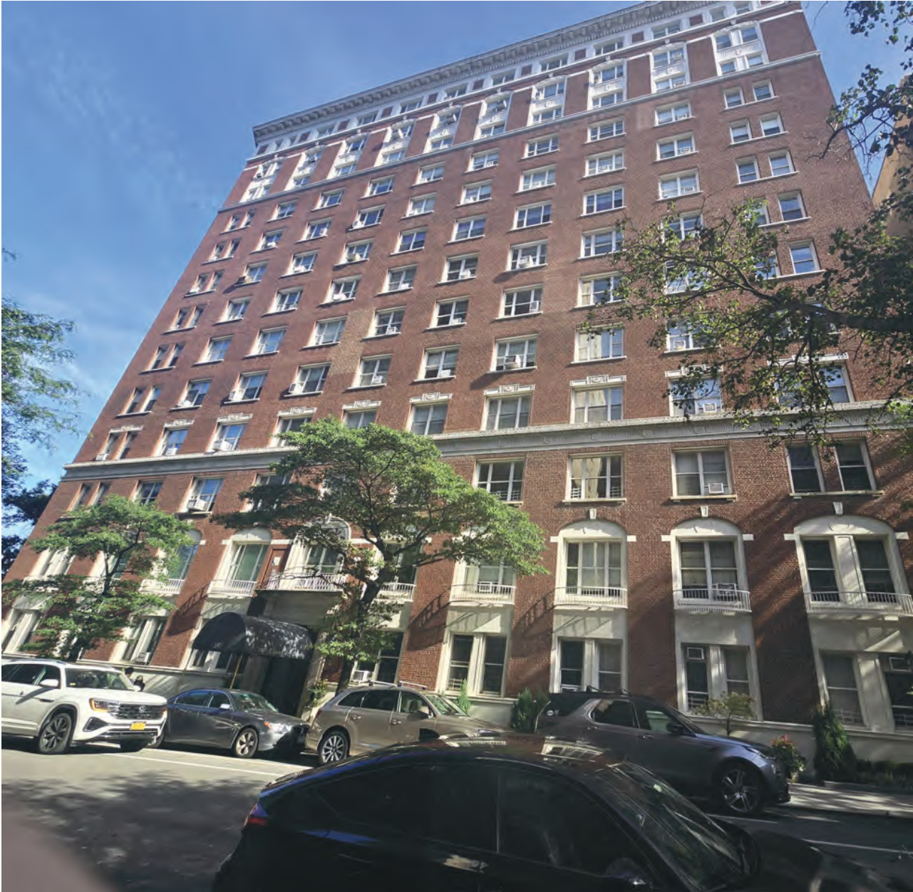
SOUTH FRONT FACADE PHOTO - OVERALL
