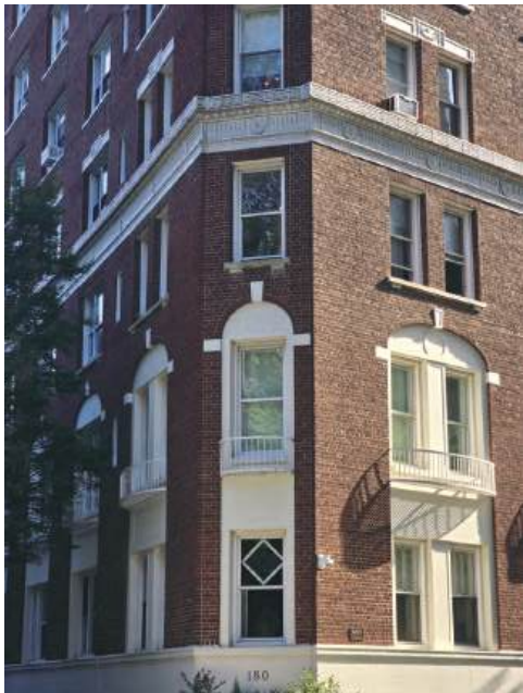
SOUTHWEST CORNER FACADE CURRENT PHOTO - LOWER LEVEL
