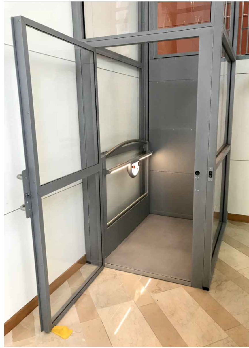
VERTICAL PLATFORM LIFT INTERIOR SAMPLE
