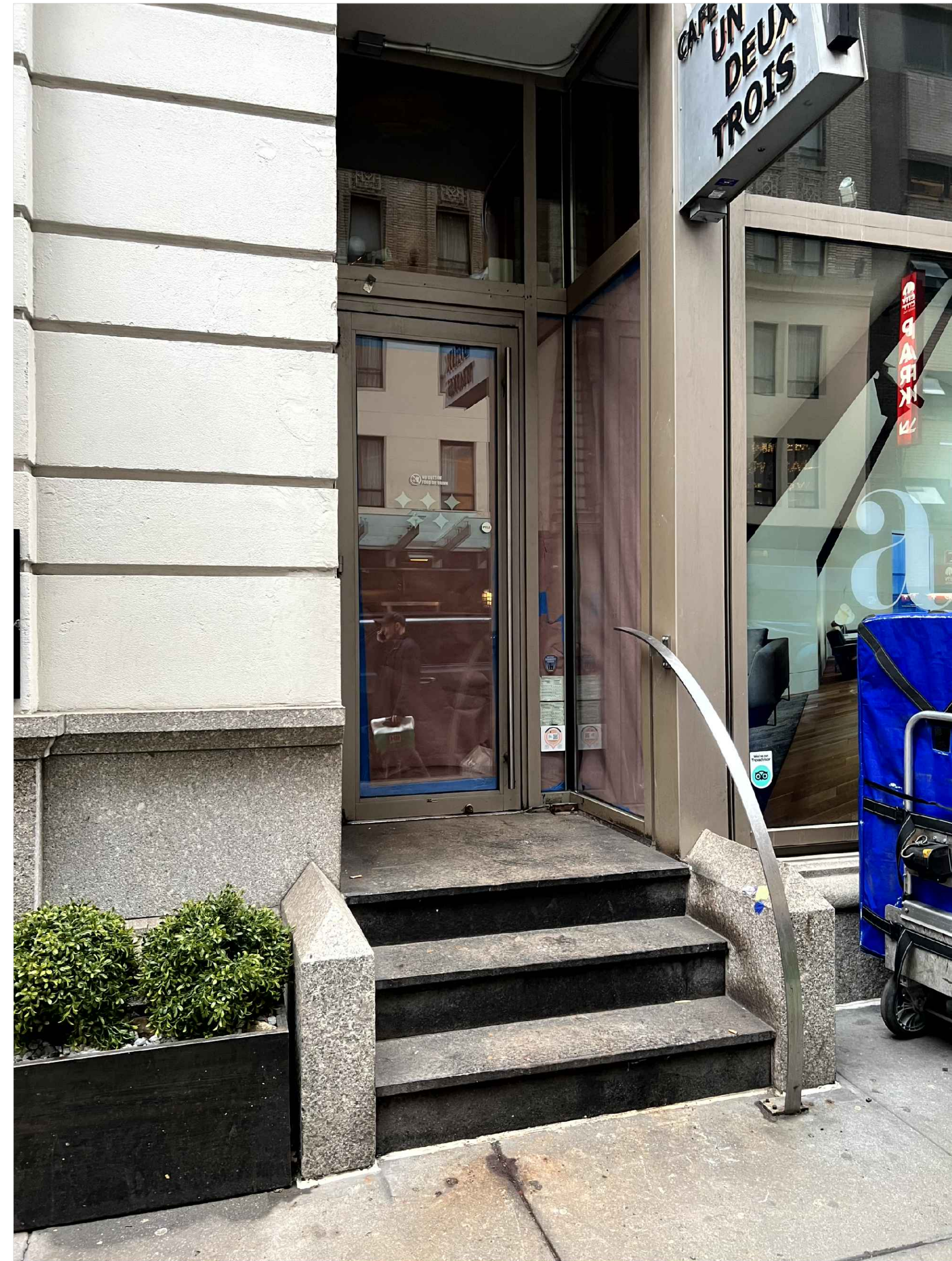
3 EXISTING EAST RESTAURANT ENTRANCE 2026 LOOKING NORTH
