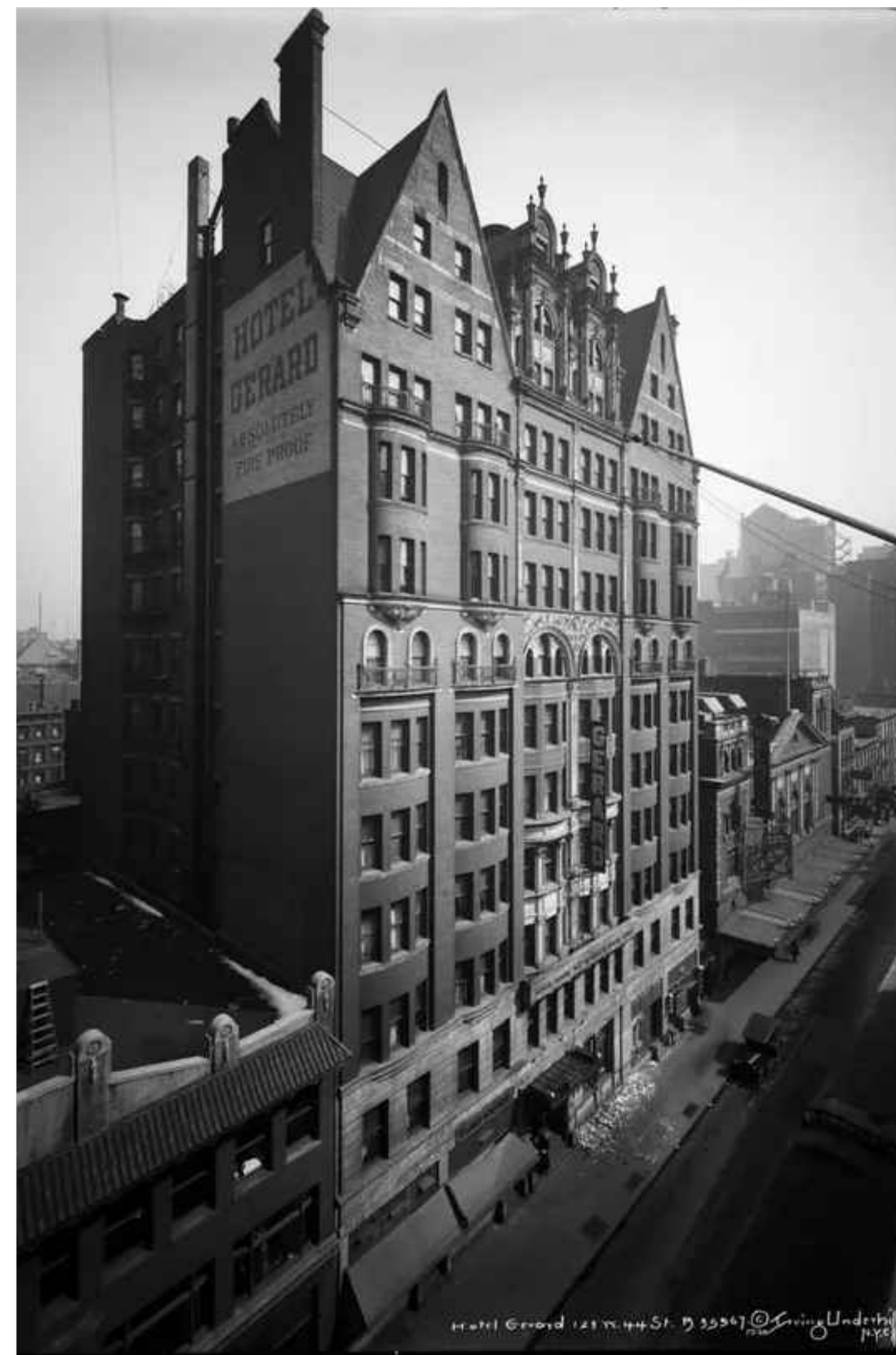
2 SOUTH BUILDING ELEVATION - HISTORIC PHOTO CREDIT: URBAN ARCHIVE | MUSEUM OF THE CITY OF NEW YORK LOOKING NORTHEAST
