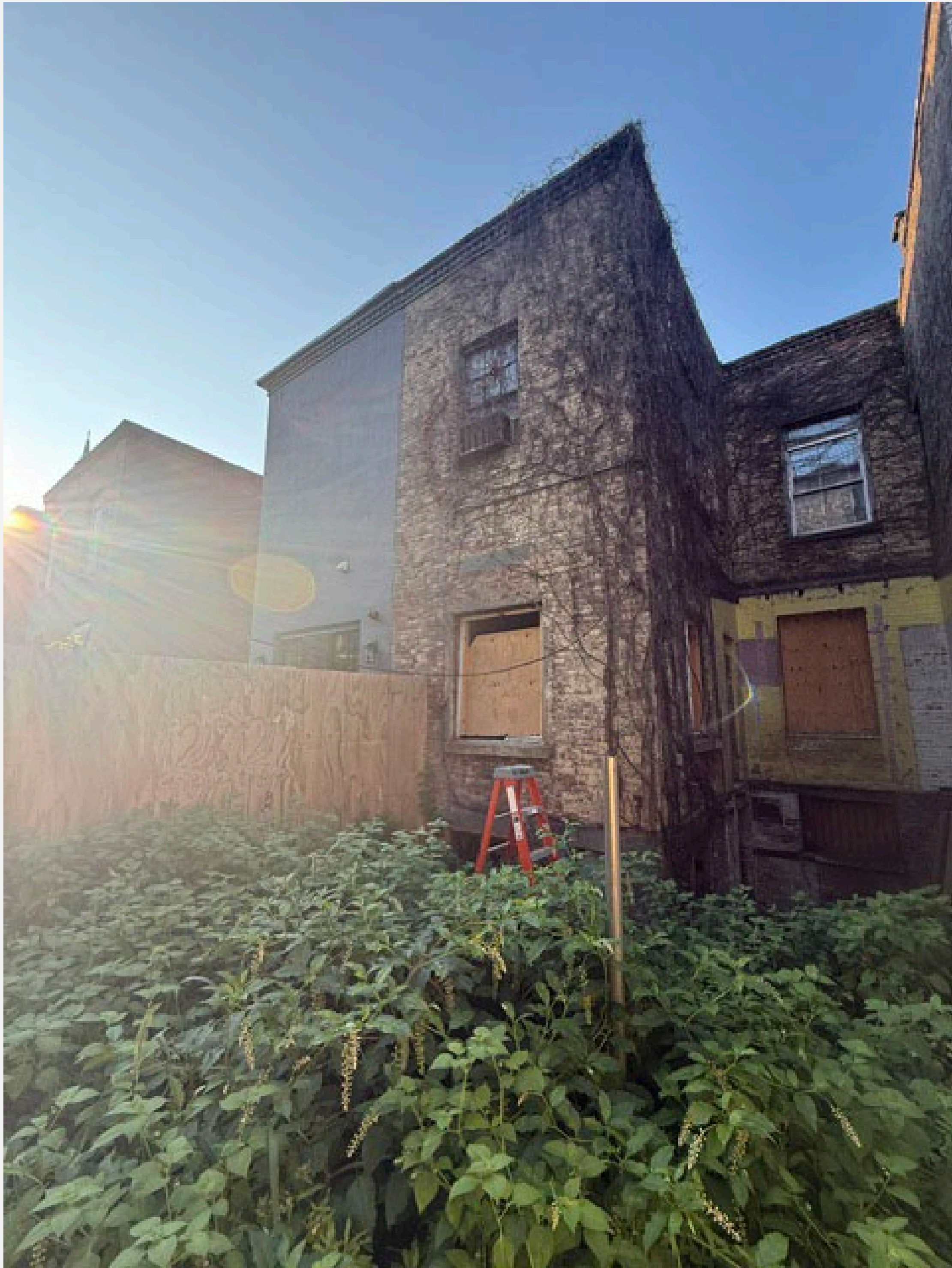
EXISTING REAR FACADE
