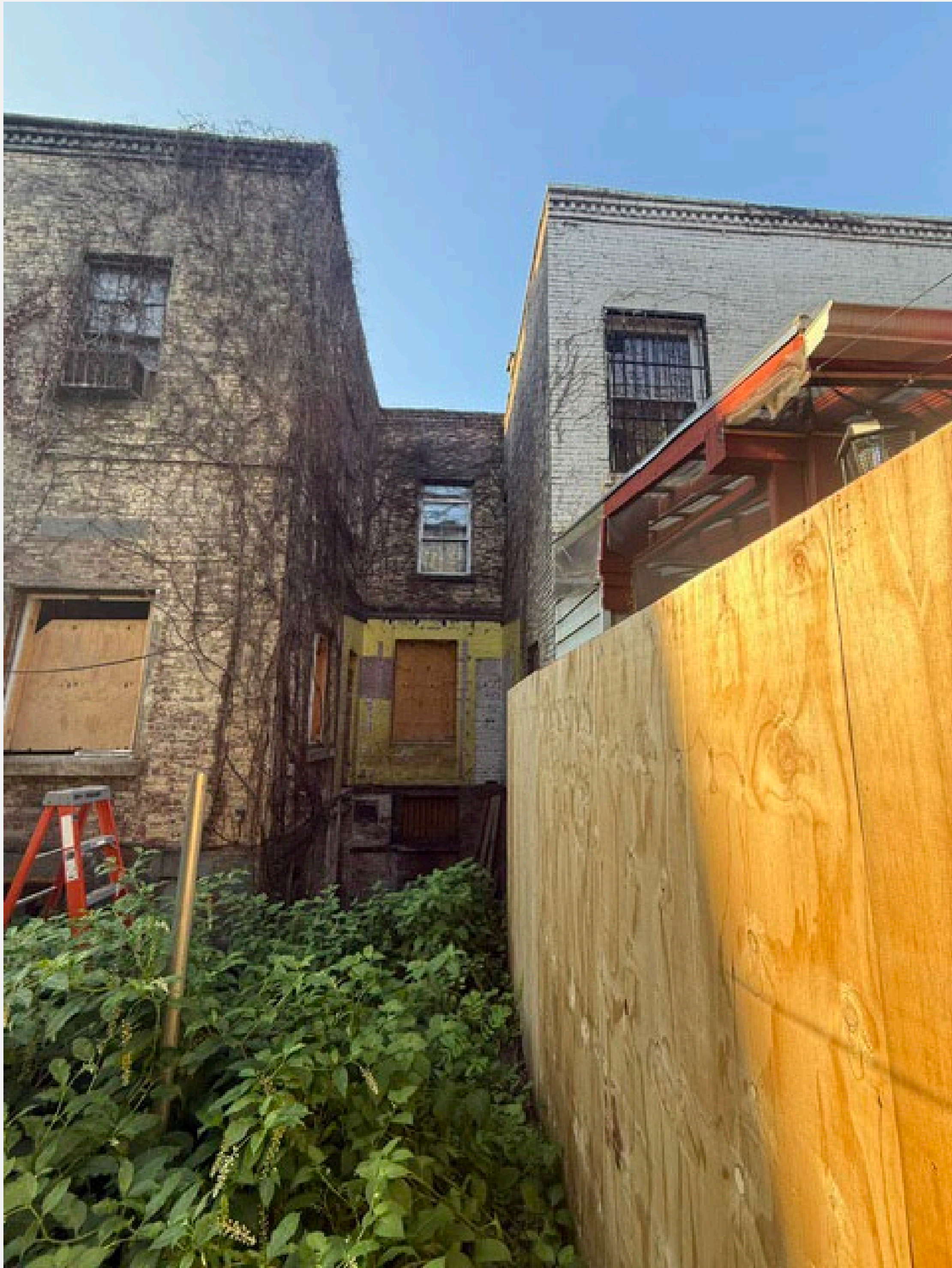
EXISTING REAR FACADE
