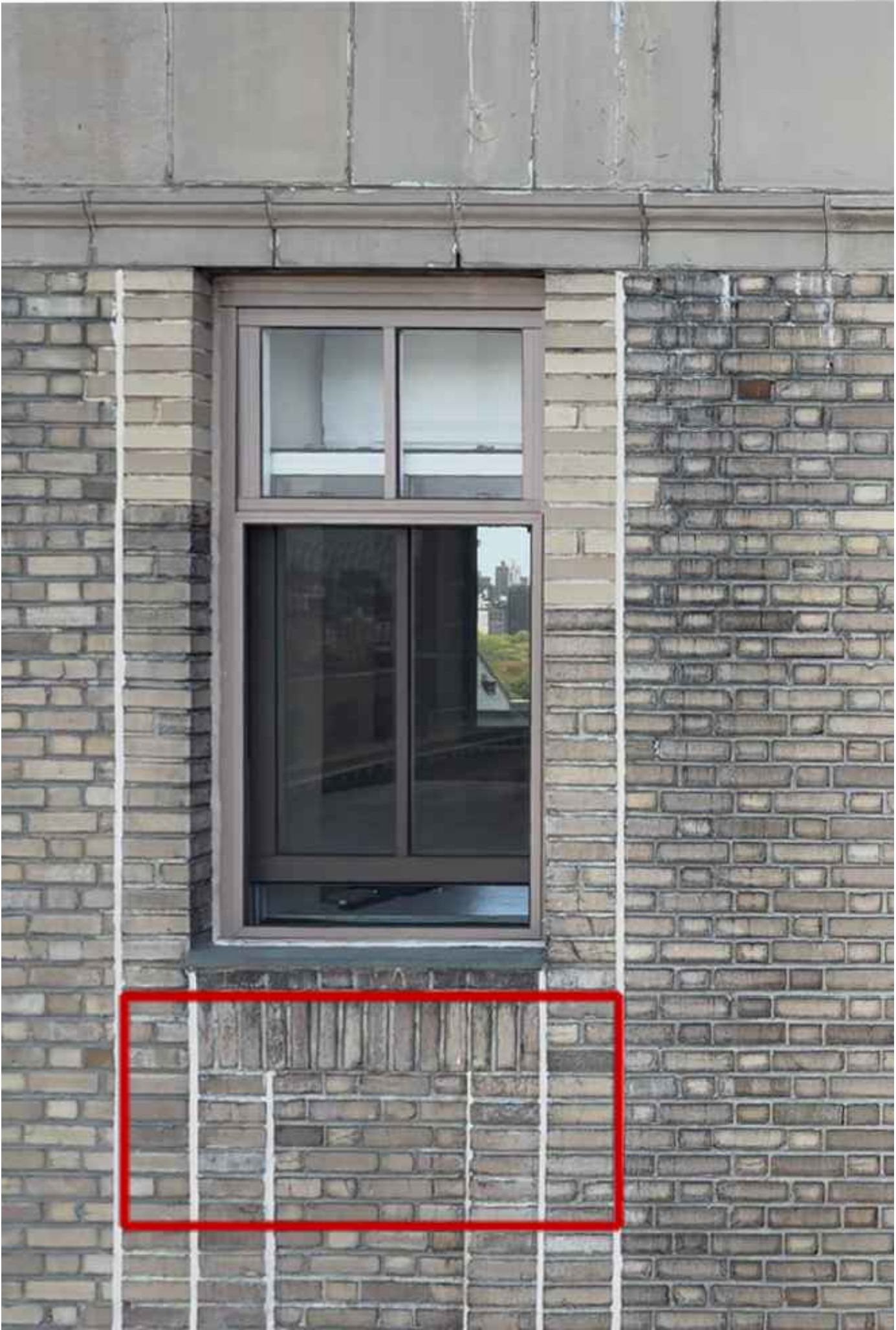
PHOTO 3 LOCATION OF PTAC UNIT
