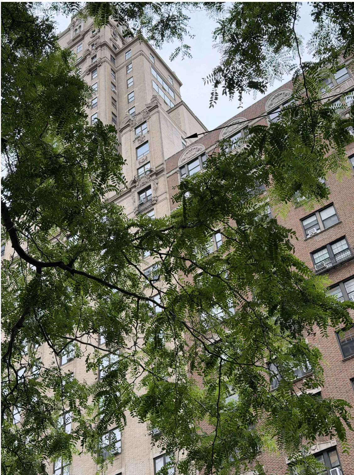
PHOTO TAKEN FROM THE SIDEWALK ACROSS FROM THE BUILDING.
