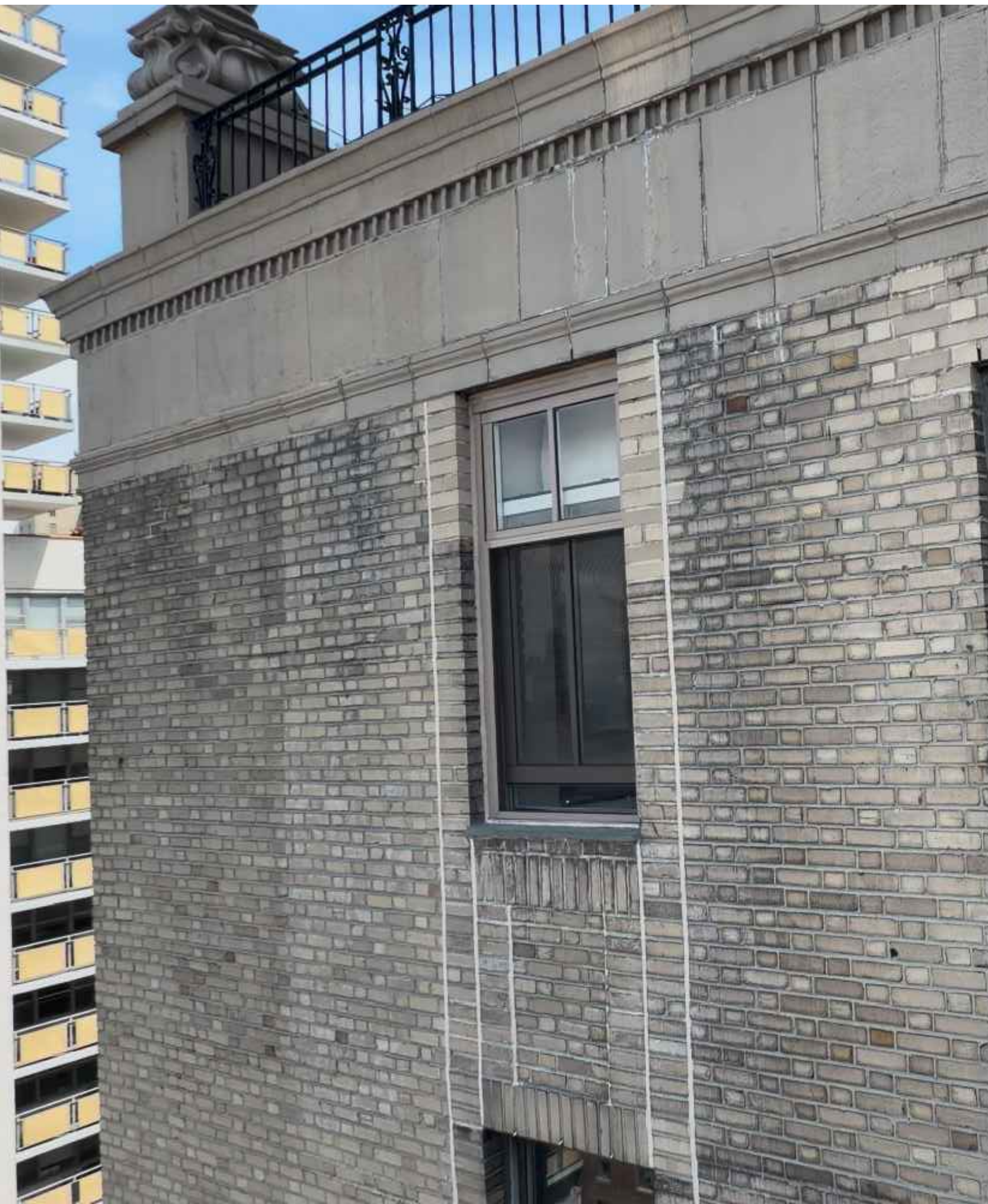
PHOTO 2 CLOSE-UP WINDOW LOCATION
