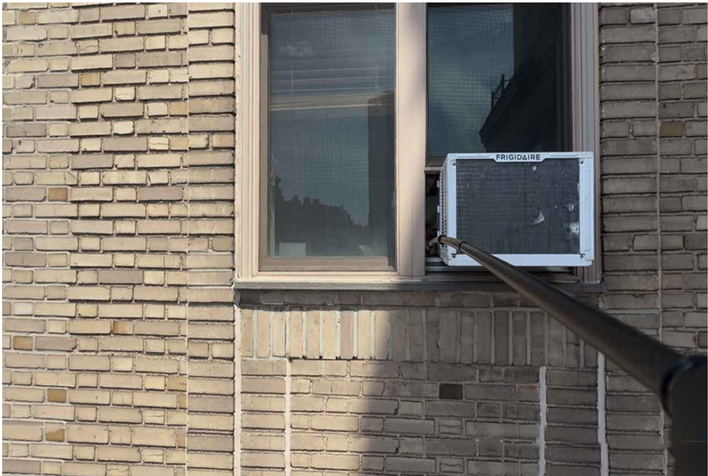
PHOTO 3 WINDOW LOCATION AT SOUTH FACADE
