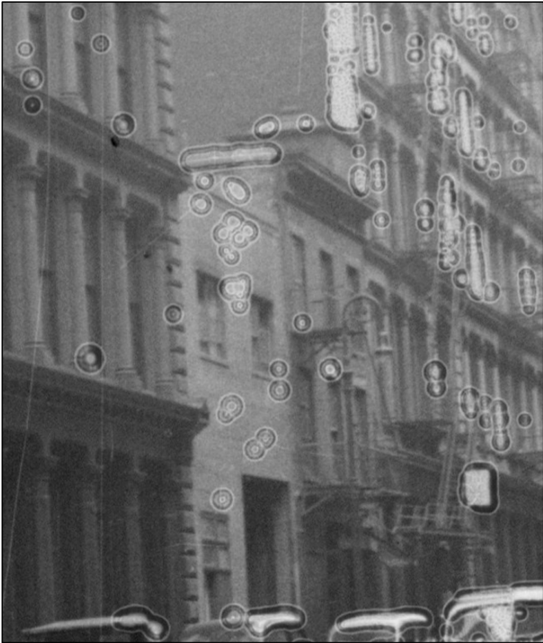
4 - 51 MERCER STREET 1940 TAX PHOTO AFTER FIRE - EXISTING GARAGE
