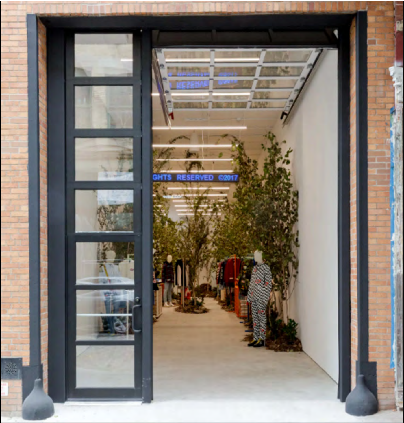
51 MECER STREET WITH THE EXISTING GARAGE DOOR OPENING
