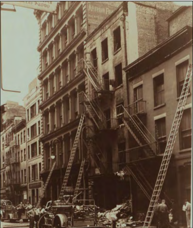
2 - 51 MERCER STREET 1940 TAX PHOTO DURING FIRE
