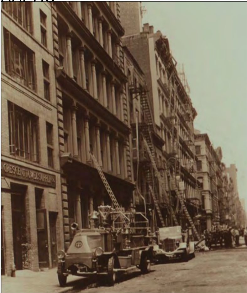
1 - 51 MERCER STREET 1940 TAX PHOTO DURING FIRE
