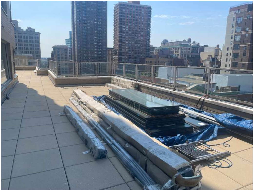
Replacement Glass Panels/Sliding Doors
