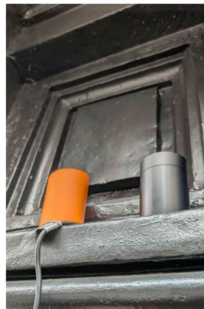
PHOTO 2. MOCKUP OF CYLINDER LIGHT AND REAL LIGHT FIXTURE PLACED AT TOP CORNICE
