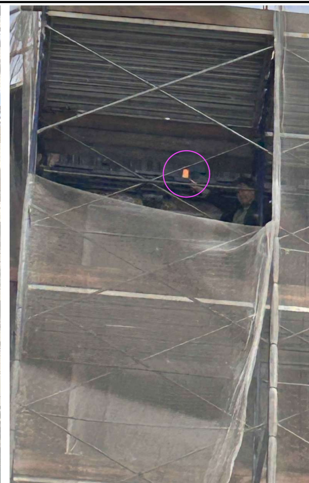
PHOTO 5. POINT A. CLOSE-UP PHOTO: ORANGE CYLINDER MOCKUP VISIBLE, BUT BLACK FIXTURE ISN'T VISIBLE @ TOP CORNICE
