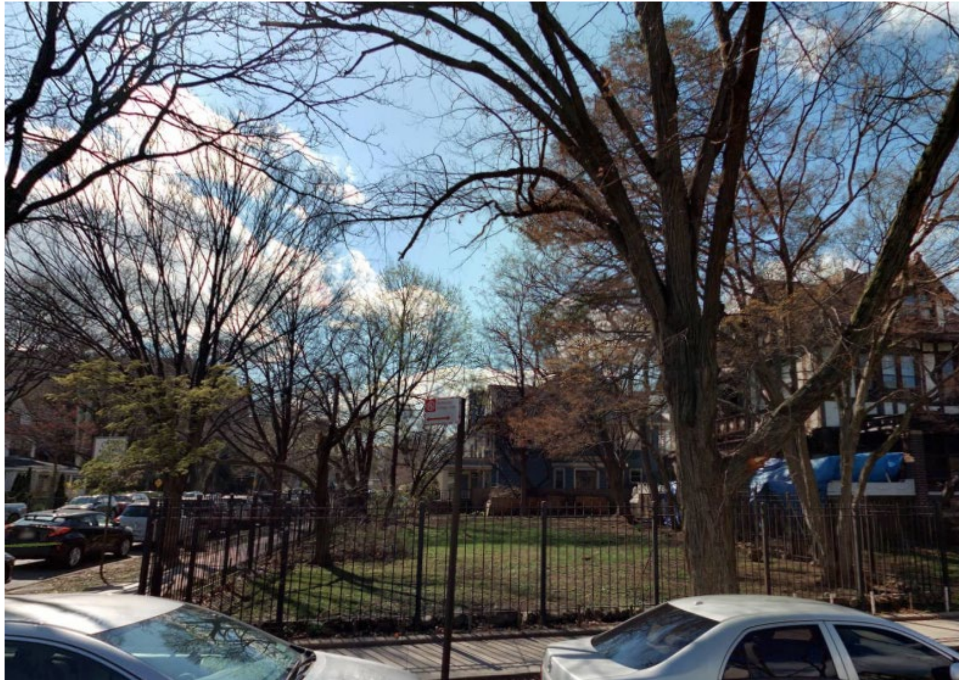
822 East 19 th Street – 6' high metal picket fence, installed prior to designation
