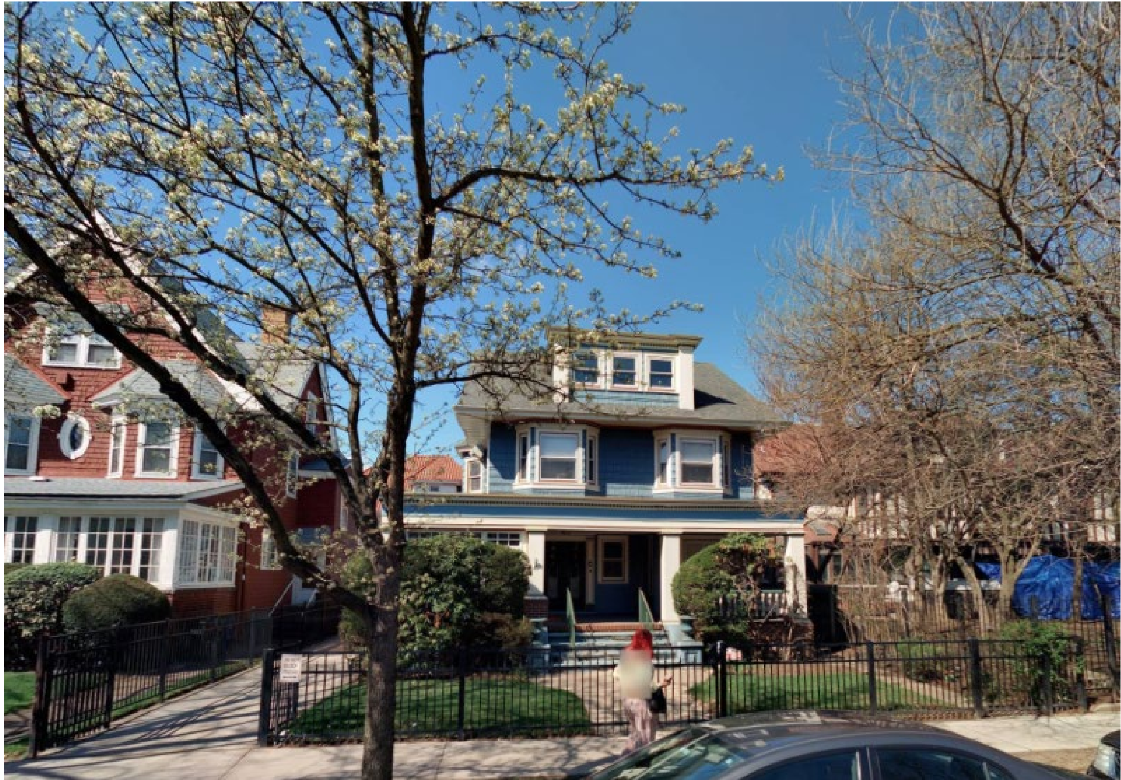
1809 Avenue H – 4' high metal picket fence, installed prior to designation
