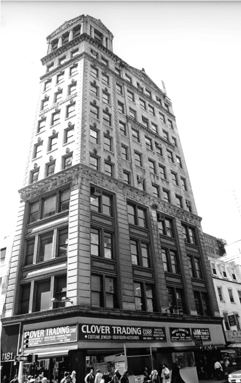
2001, LPC Designation Photo
