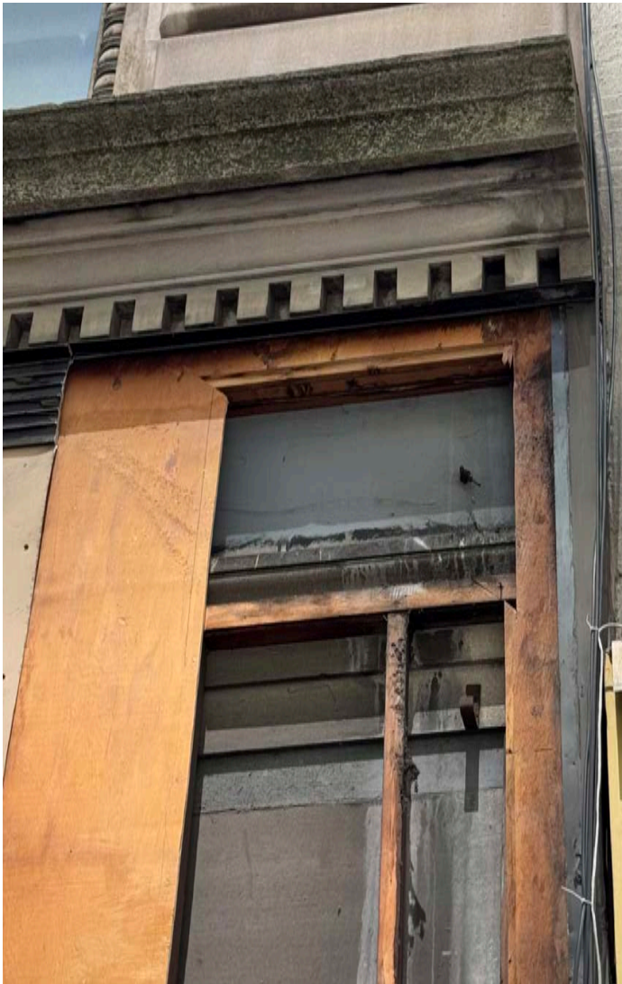
2026, Storefront - Cornice at 28th St
