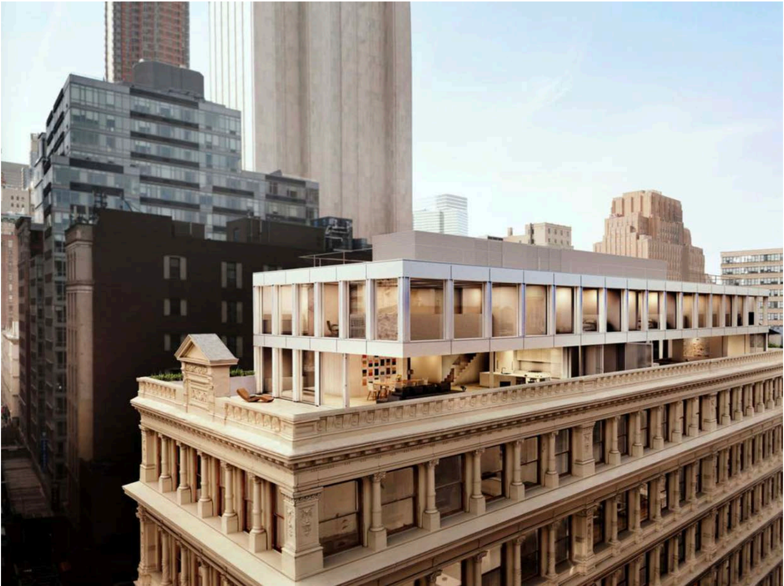
361 Broadway Roofotp addition approved by LPC 06/05/12
