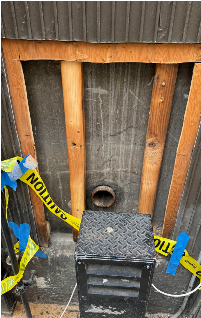
2026, Storefront - Base pier at 28th St
