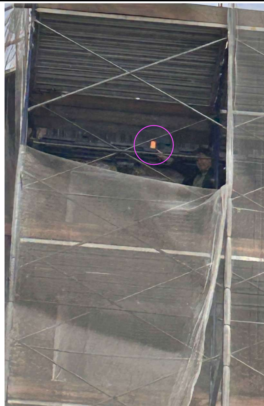
PHOTO 5. POINT B. CLOSE-UP PHOTO: ORANGE CYLINDER MOCKUP VISIBLE, BUT BLACK FIXTURE ISN'T VISIBLE @ TOP CORNICE
