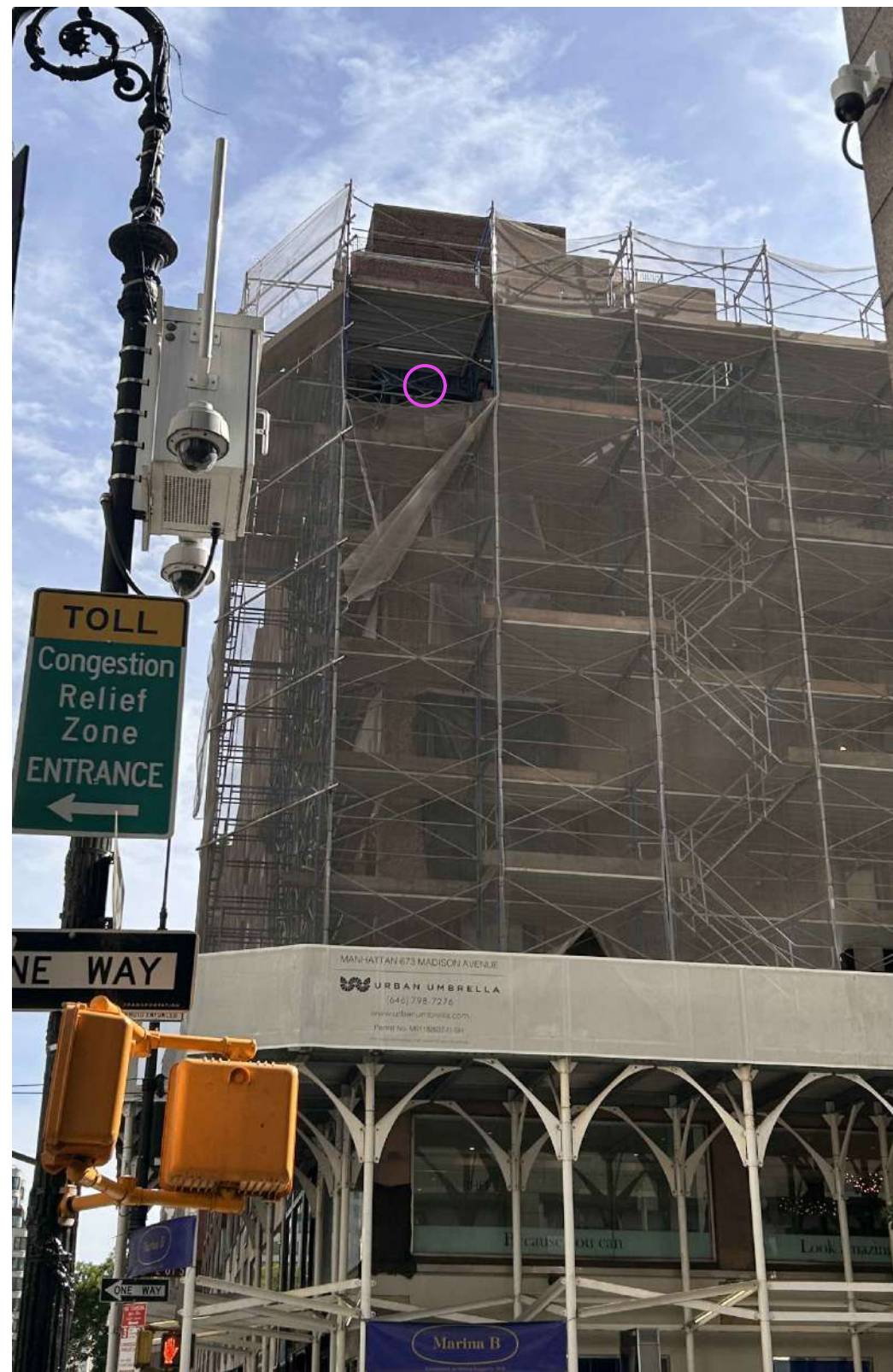
PHOTO 8. POINT D. BLACK FIXTURE ISN'T VISIBLE @ TOP CORNICE
