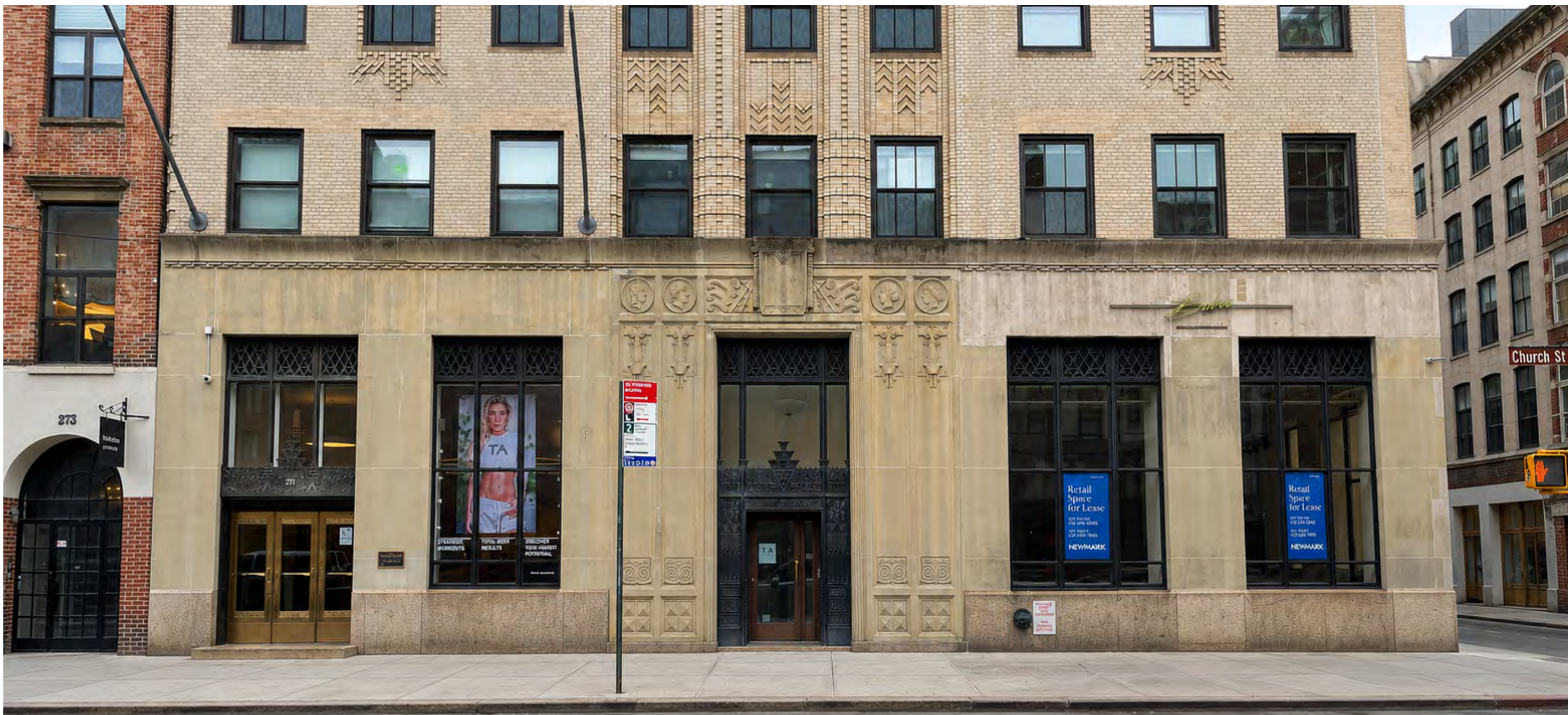
1 EXISTING CONDITION PHOTOS CHURCH STREET FACADE
