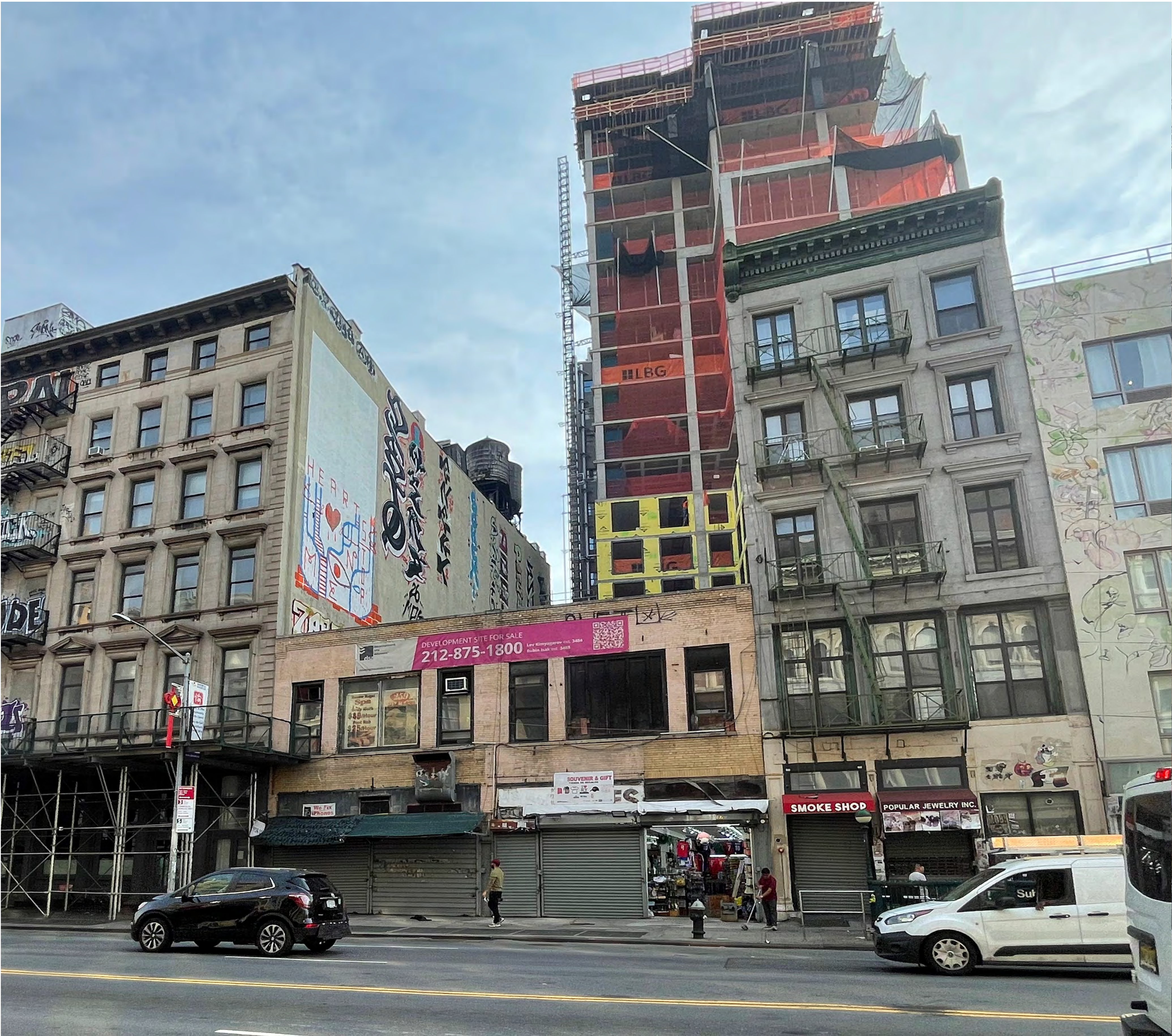
EXISTING SITE CONDITIONS
