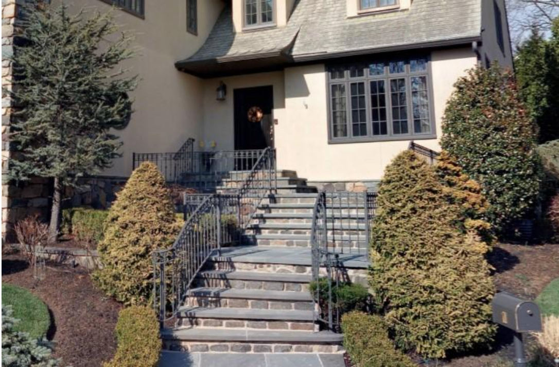
Ironwork at 71 Flagg Court
