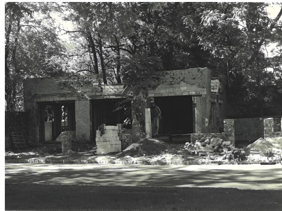
Construction from garage to residence 1989. (LPC Archives)
