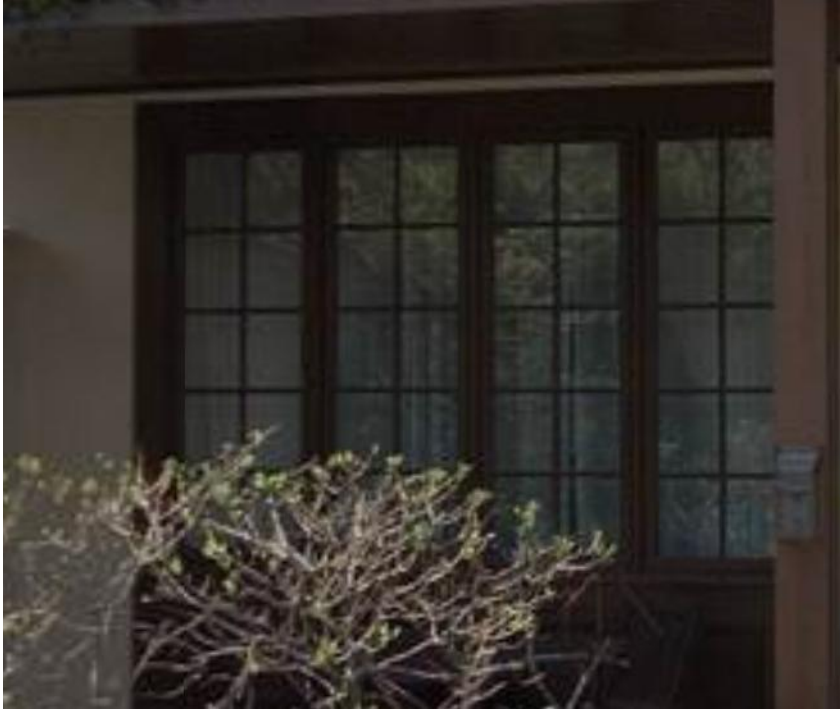
Ten pane windows. (Cyclomedia 2018)
