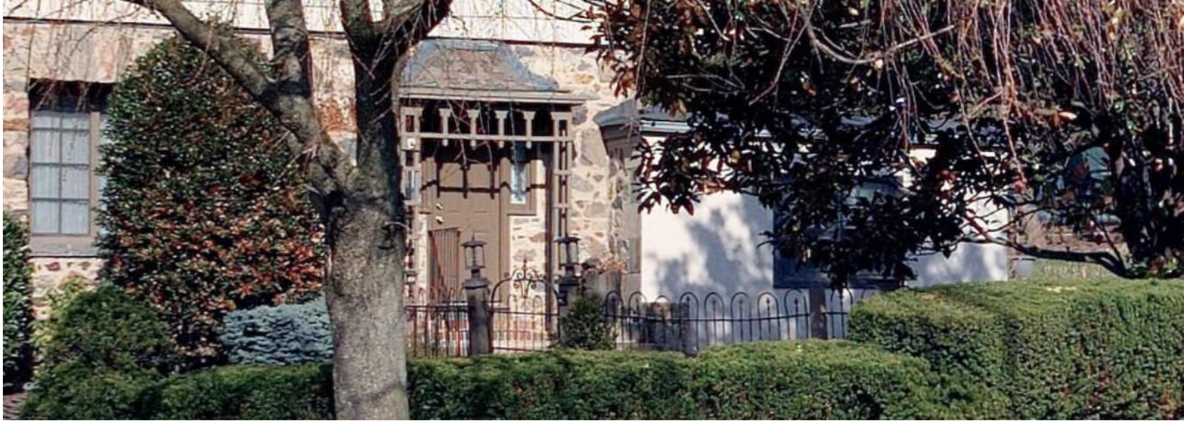
Ironwork at The Gardener's Cottage 45 Flagg Court
