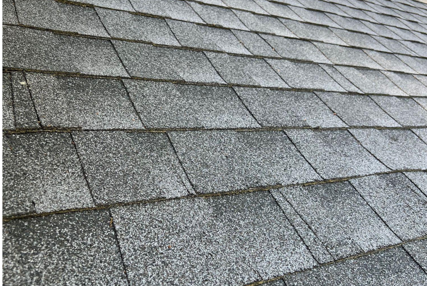
Asphalt shingle upclose.
