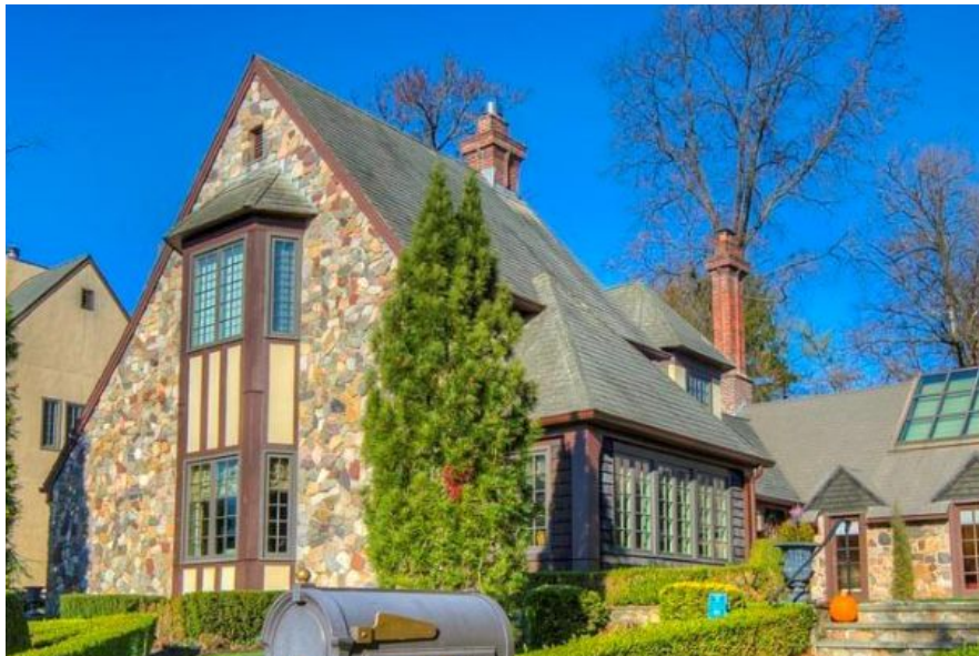
63 Flagg Court. Original Palm House. Historic, modified. Grey asphalt shingle roof, uniform window layout, color, material.
