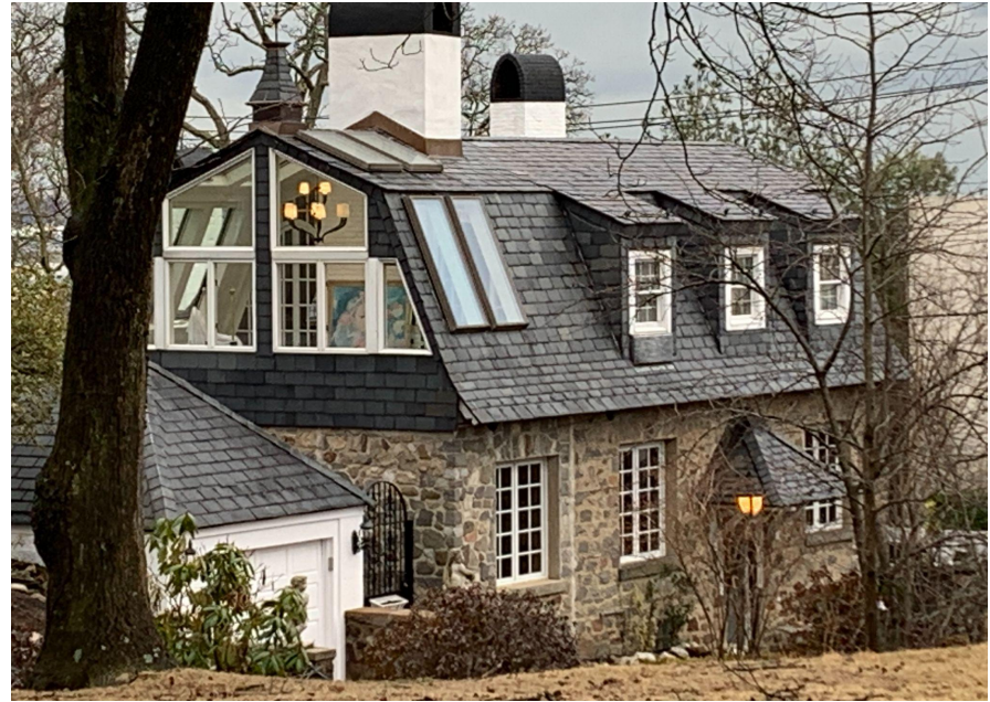
Gatehouse 181 Flagg Place - originally wood shingle, replaced with slate by Flagg
