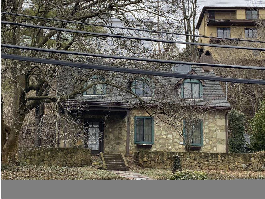
McCall's Demonstration House 1929 Richmond Avenue - originally rolled roofing, then slate, now asphalt shingle
