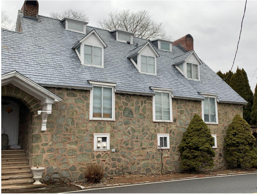
Wallcot 285 Flagg Place - faux slate shingle roofing
