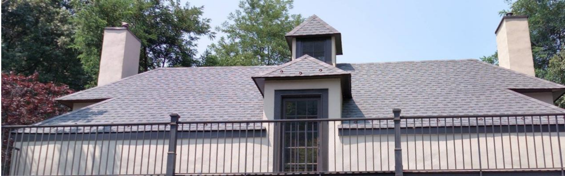
Completed roofing. (Cyclopedia 2025)
