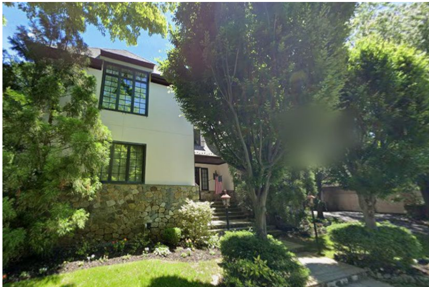
15 Flagg Court. Grey asphalt shingle roof, uniform window layout, color, material. (1980s contemporary construction.)
