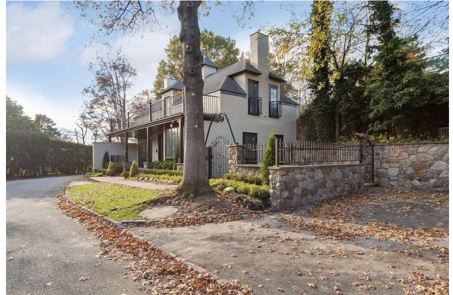
View from Flagg Court. (Facing west)
