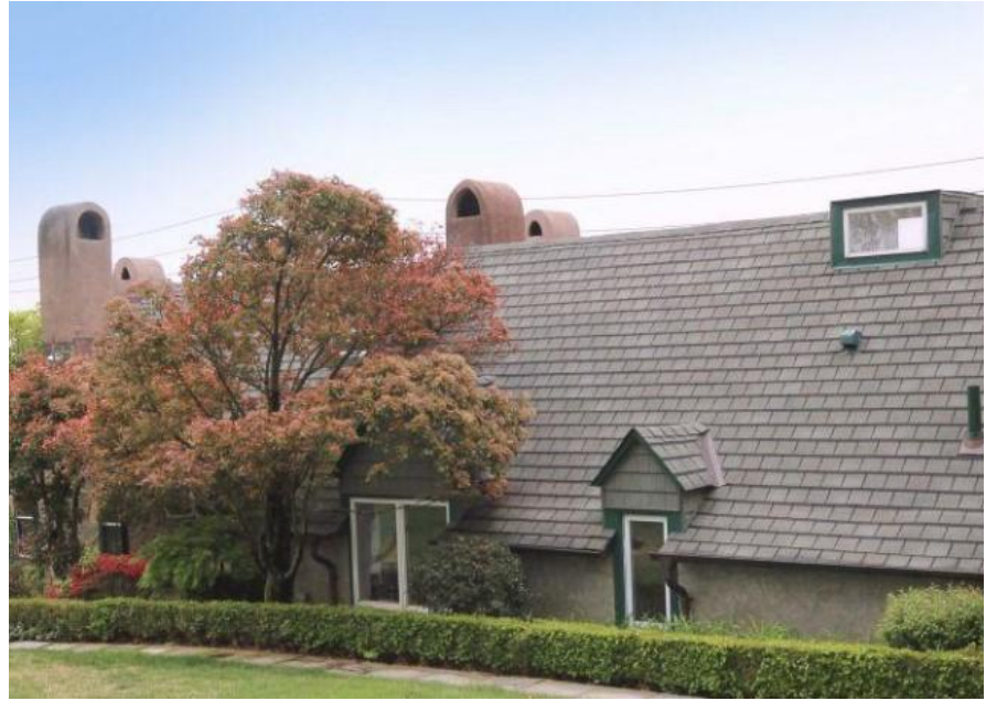
Bowcot 95 Westentry Road - asphalt shingle roofing
