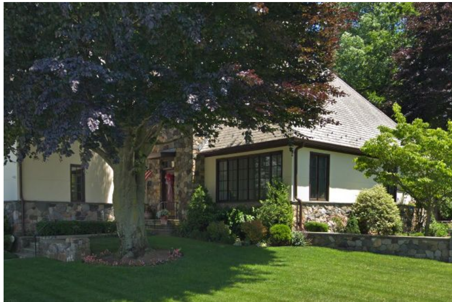
39 Flagg Court. Grey asphalt shingle roof, uniform window layout, color, material. (1980s contemporary construction.)
