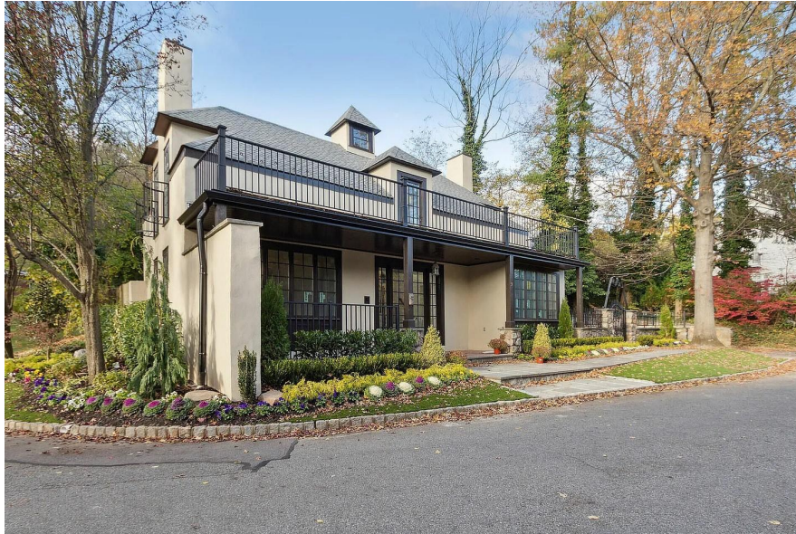
View from Flagg Court. (Facing northeast)
