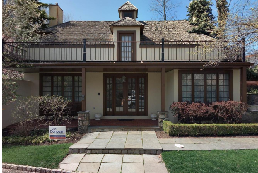
View from Flagg Court facing northwest. (Cyclomedia 2018)
