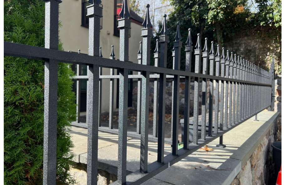
Upclose of ironwork. Aluminum black powder coat.
