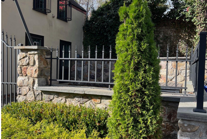
Street view of gate and ironwork facing Charter Oak road.
