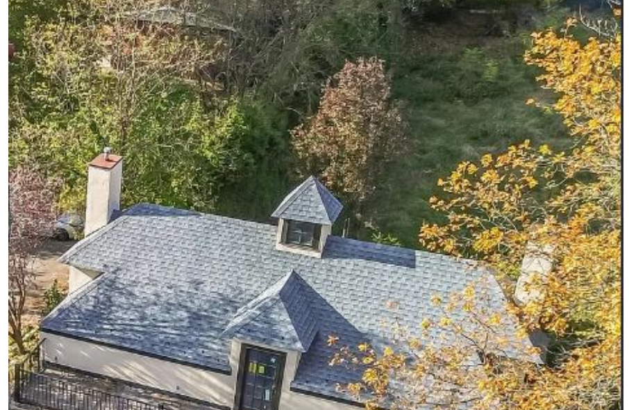
Aerial view of completed roof.
