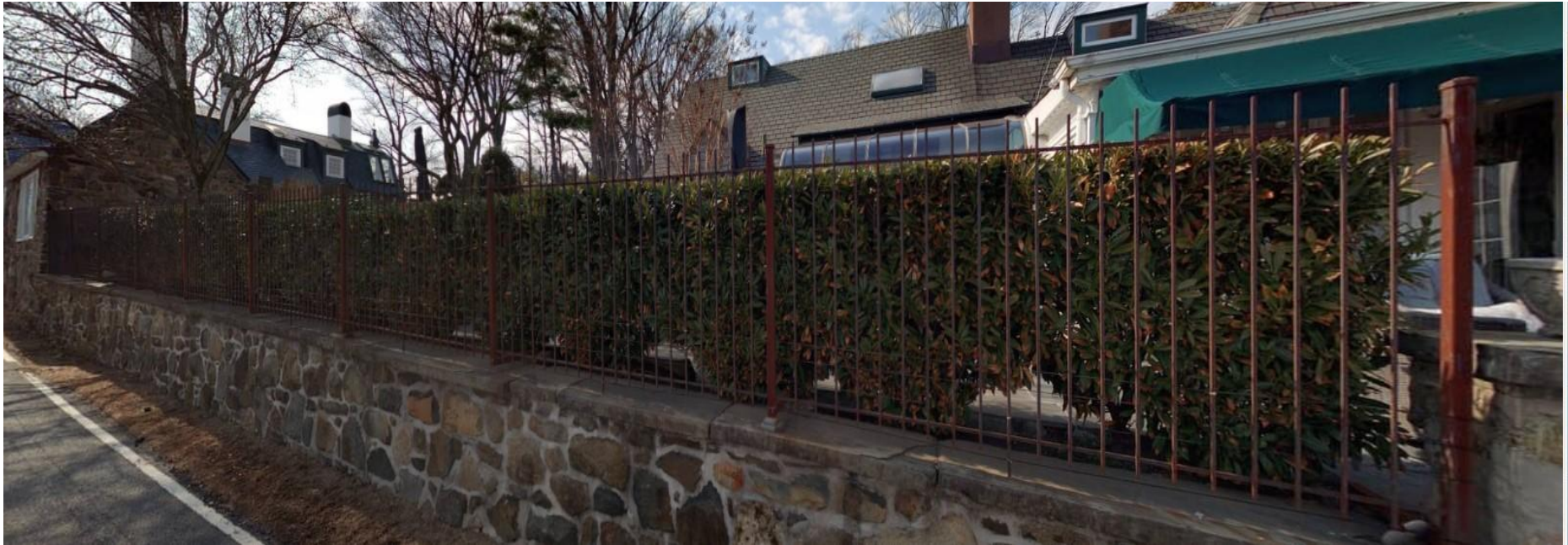
Ironwork connecting the Gatehouse & Bowcot residences
