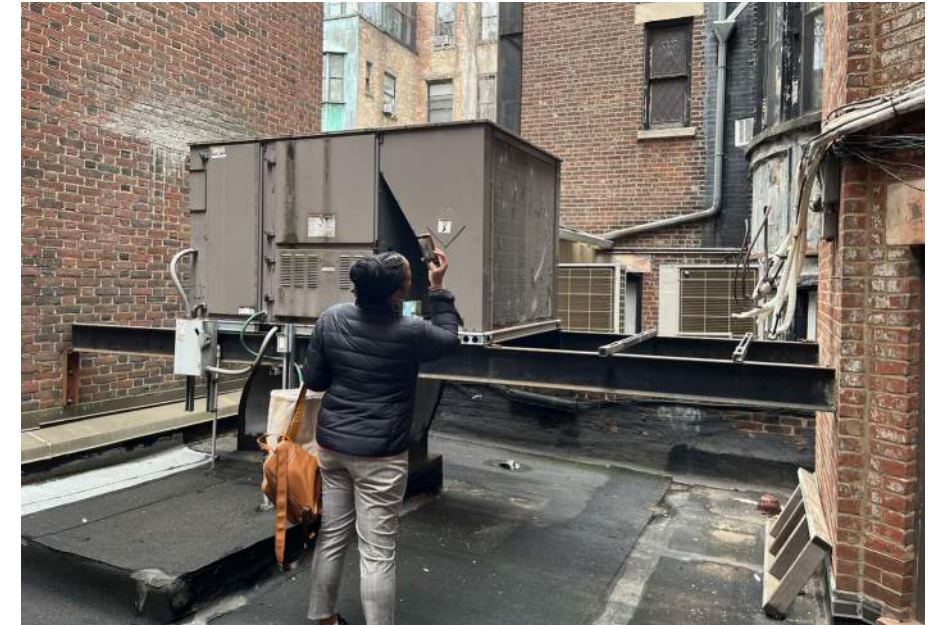
Existing Rear Yard at Rowhouses
