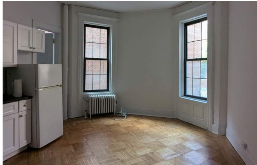
Existing Apartments at Rowhouse
