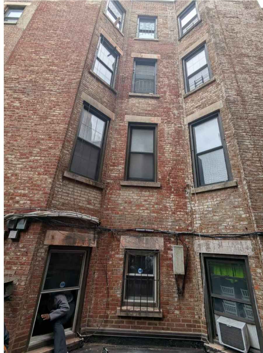
1307 Rowhouse Rear Facade
