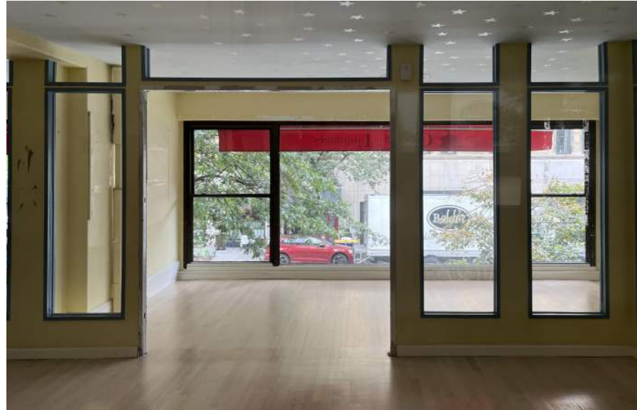
Existing Commercial Space at Rowhouse
