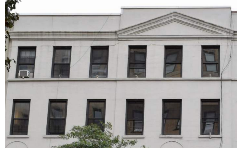
Existing Townhouse Facade
