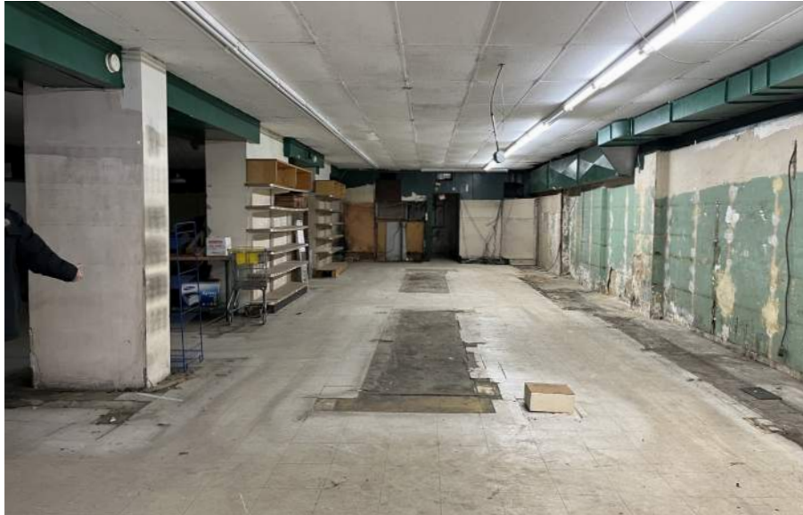
Existing Retail 1st Floor at Rowhouse
