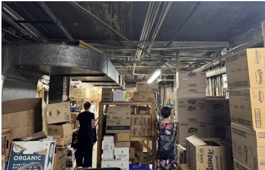
Existing Retail Cellar at Rowhouse
