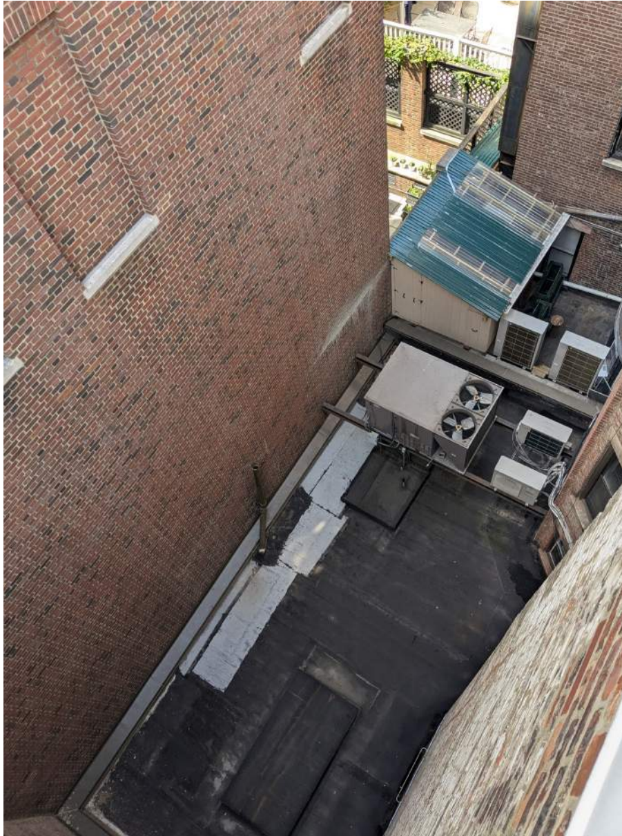
Rowhouse Rear Yard
