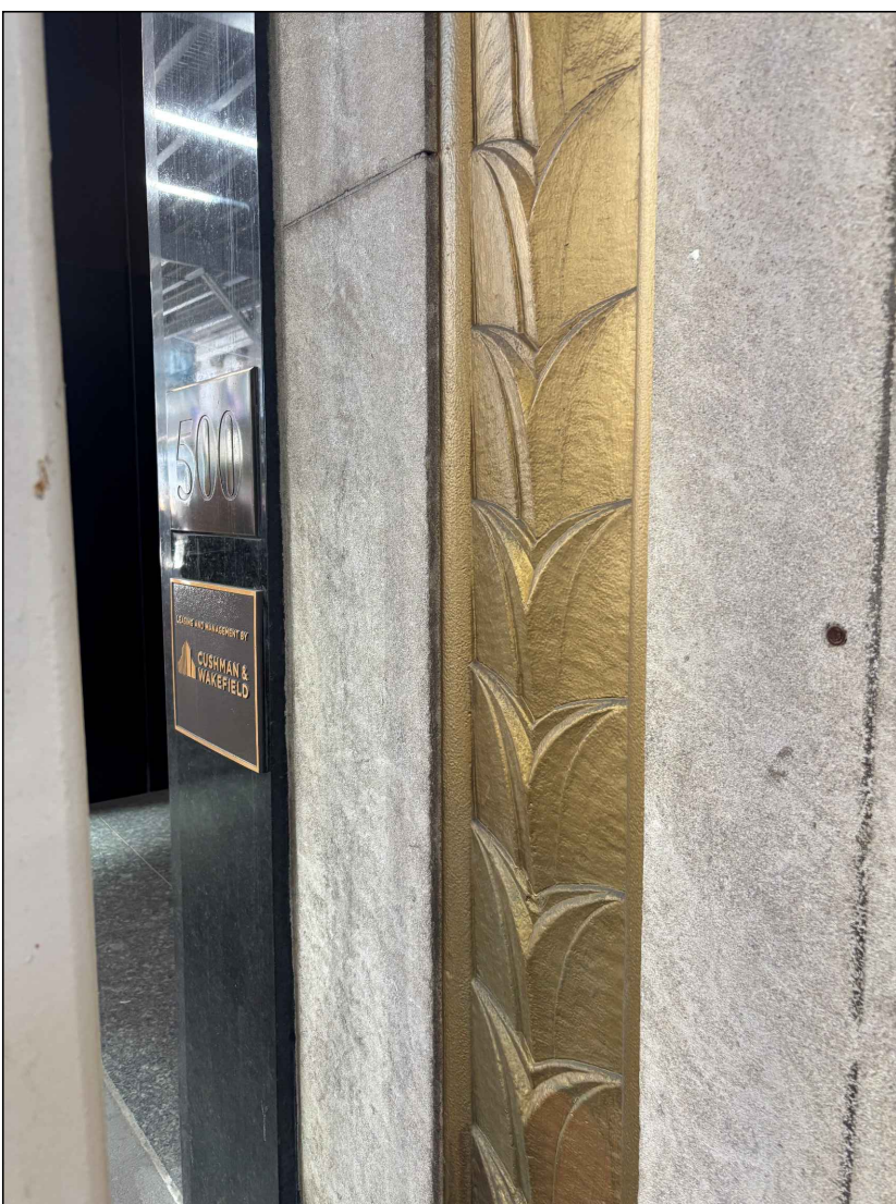
3 CLOSE-UP PHOTO OF EXISTING GOLD ACCENT PAINT AT EAST ELEVATION MAIN ENTRY SCALE: NTS
