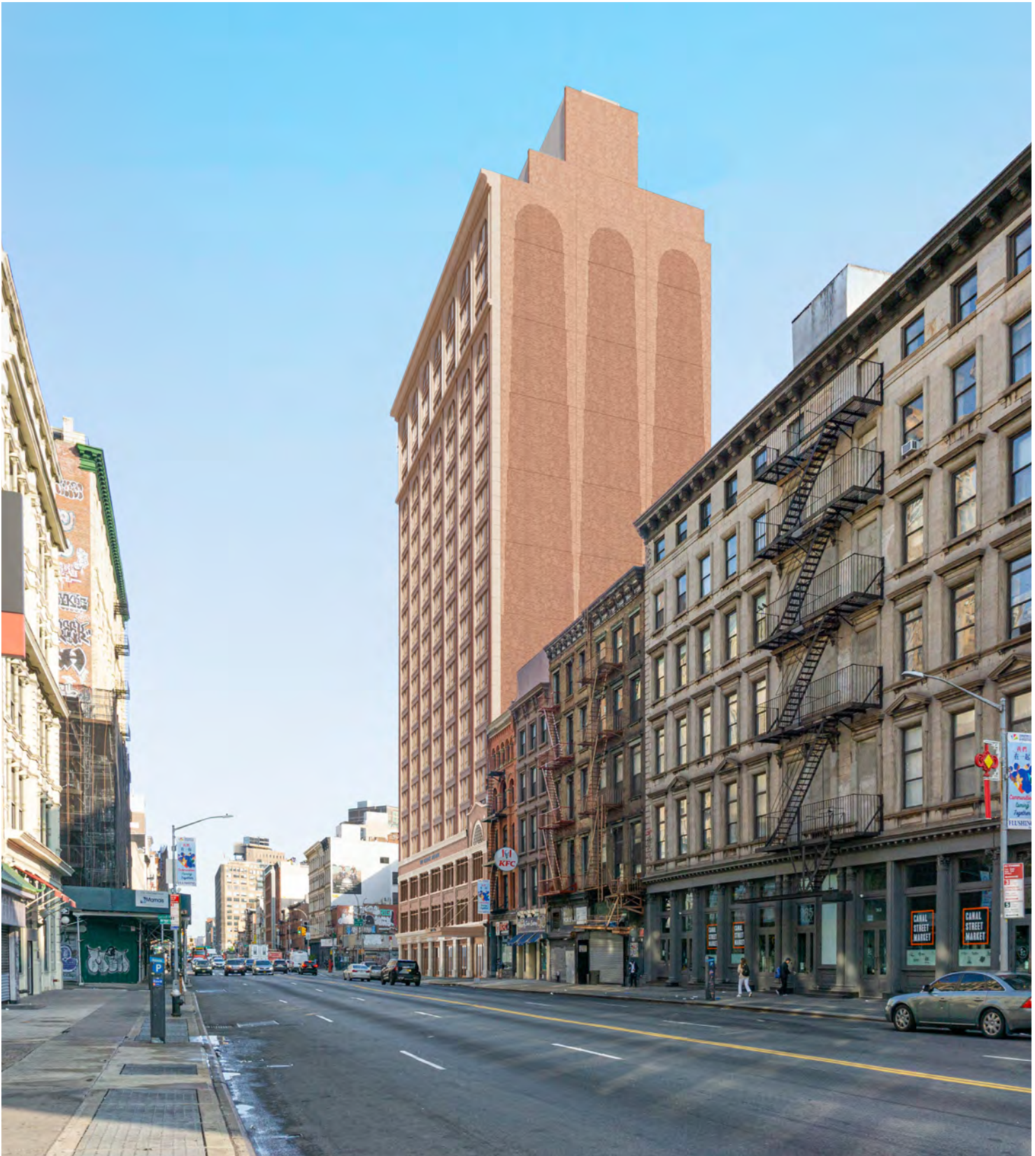
Canal St (Looking West)
