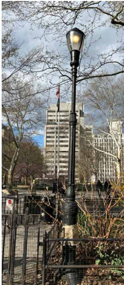
Type 1 E pole with 2085 Luminaire, 12' Ht.
