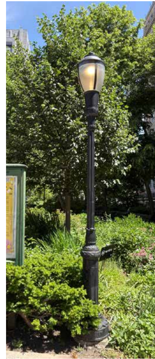
Type 4 B pole with 2085 Luminaire, 8' Ht.
