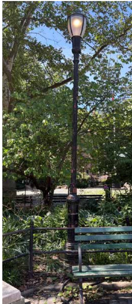
Type 2 B pole with 2085 Luminaire, 12' Ht.
