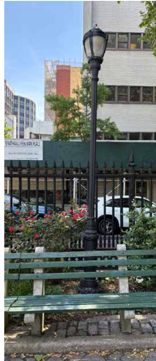
Type 3 B pole with Riverside Luminaire, 12' Ht.
