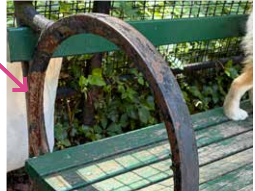
Corrosion on metal
