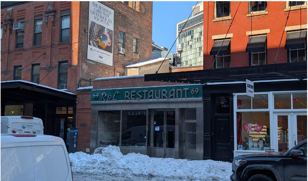
3 | VIEW FROM ACROSS GANSEVOORT STREET
