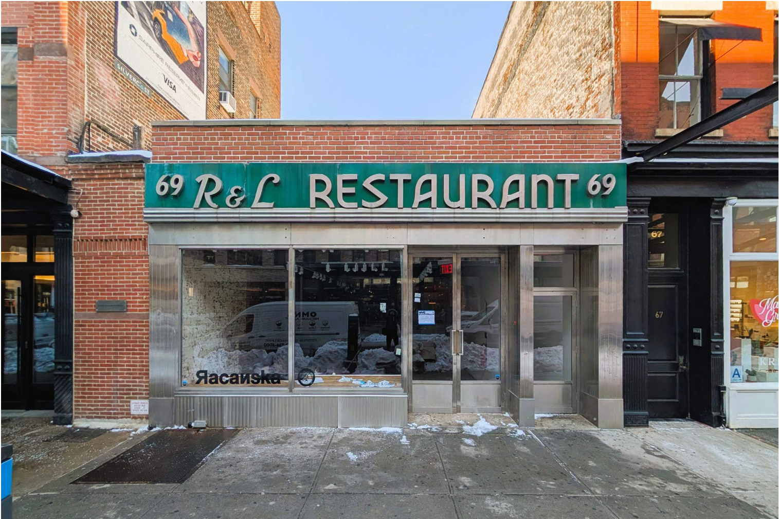
EXISTING SOUTH FACADE
