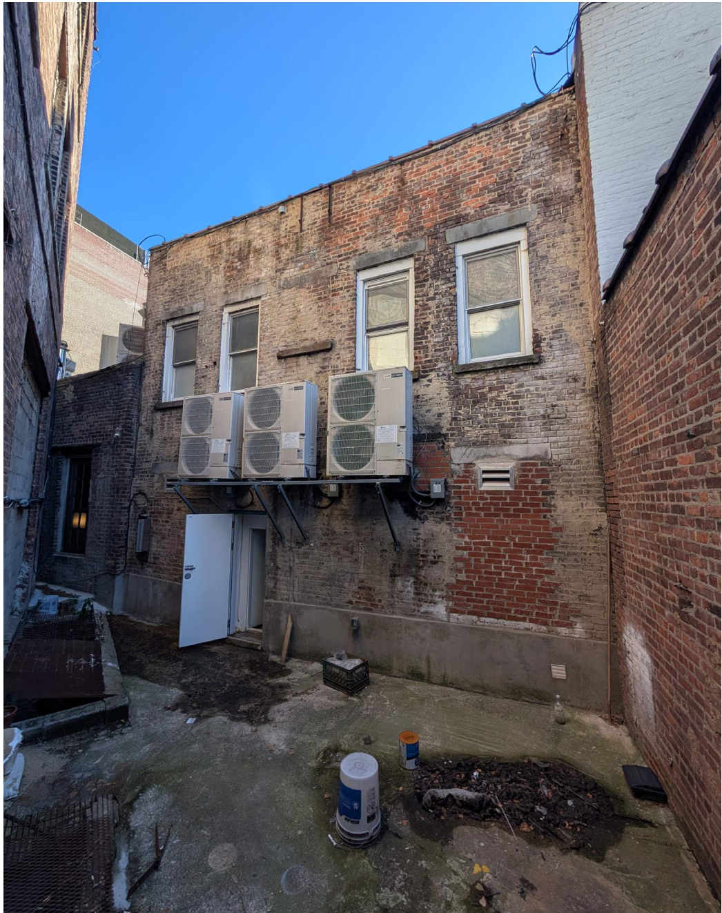
1 | NORTH ELEVATION - REAR FACADE
