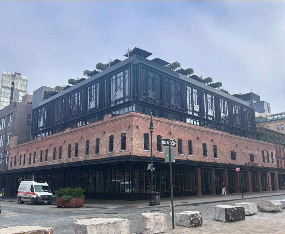
19 9TH AVENUE LPC COFA 16-4882 | PERMIT ISSUED 11/24/2014 CONTRASTING MODERN INTERVENTION
