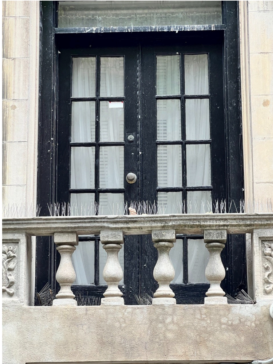
Exterior view of current balcony door
