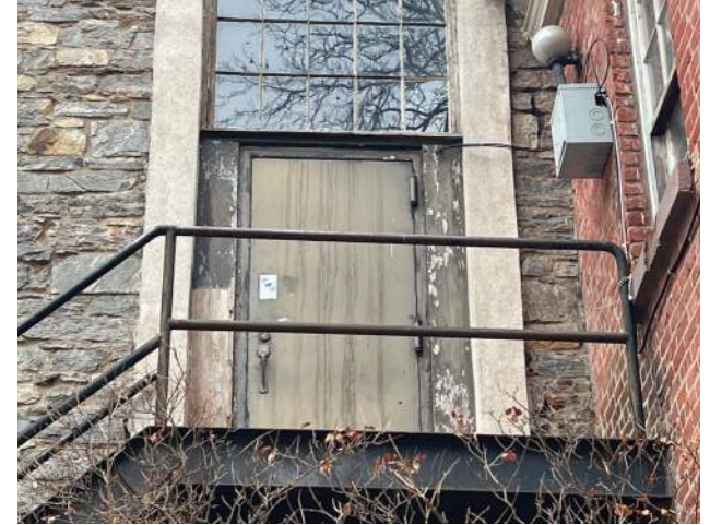
The Parish Hall emergency exit door from the second floor is out of place as a flat metal panel in a window wall. Its plywood frame has failed.
