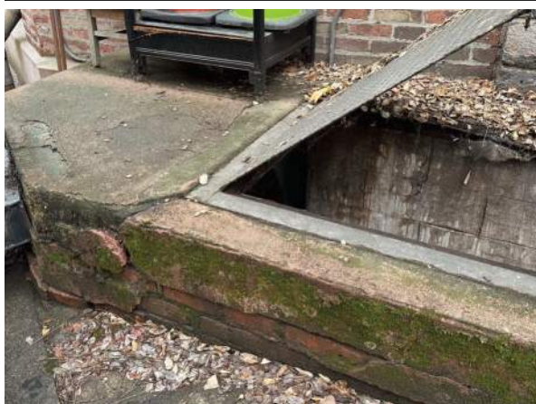
A17-1 - REPLACE AREAWAY VAULT DOORS AND CURB
