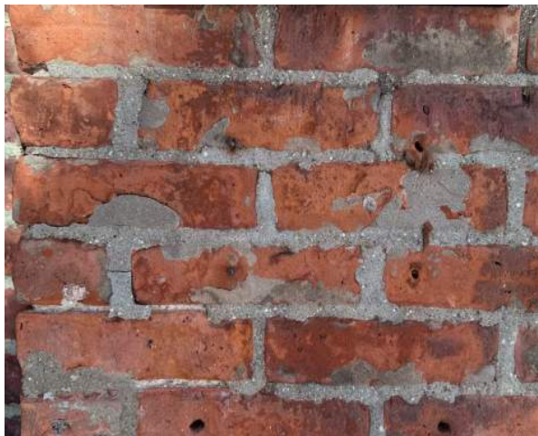
A30 - REPOINT PARISH HALL MORTAR JOINTS
