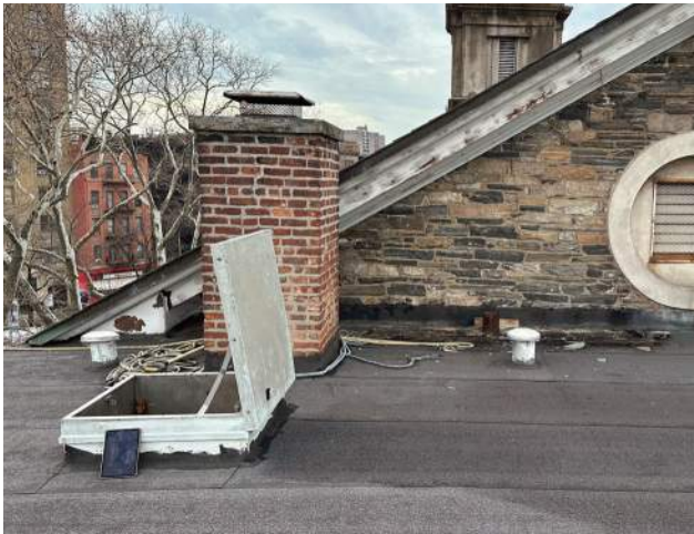
A hatch opens from the 2FL ballet studio balcony onto the low-slope roof.
