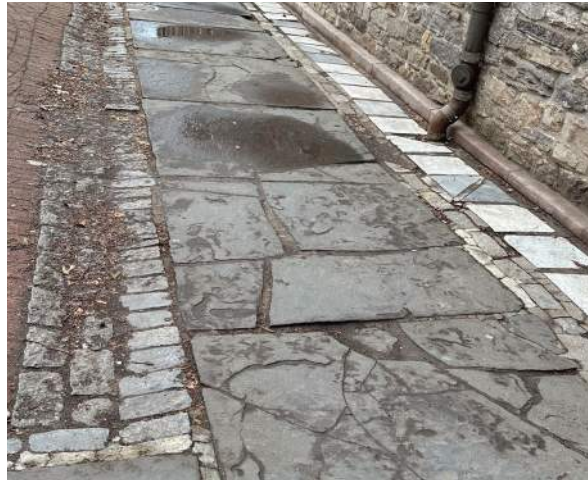
A53 - REPAIR SITE PAVING TO PARISH HALL
