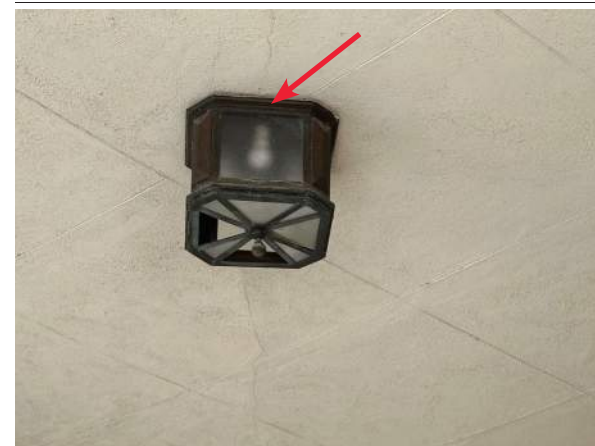
A11-2 - REPAIR CRACKS AT PORTICO CEILING STUCCO
