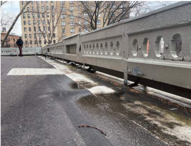
The roof membrane appears to have been in place before the parapet and base flashings were repaired, before 2017, but is in sound condition.
