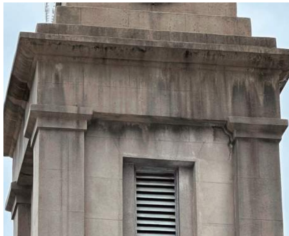
A31 - CLEAN MASONRY FACADES
