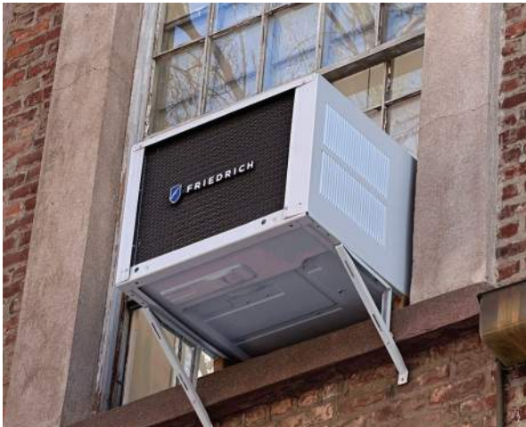
A04 - PROVIDE WEATHER SEALS AT A/Cs
