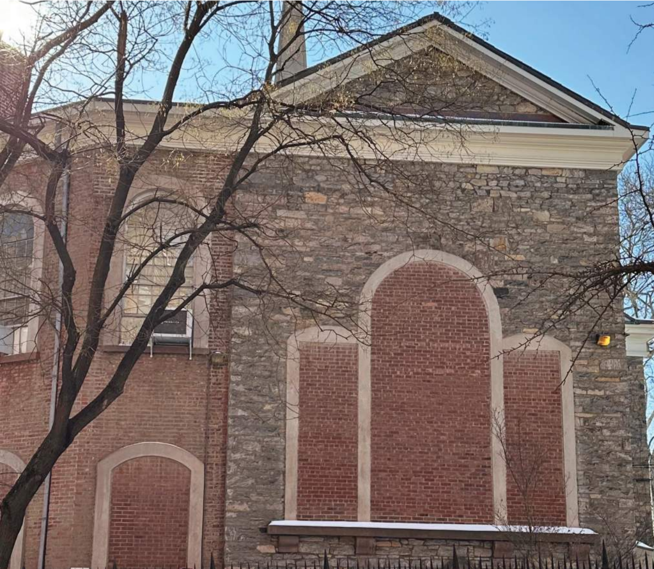
The east facade showcases the gable end of the stone wall and brick walls that are in good condition. Wood windows on both buildings are replacements.
