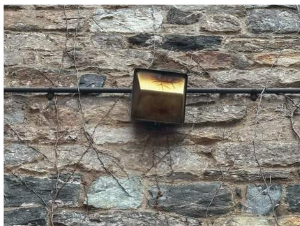
A54 - REMOVE NON-FUNCTIONING LIGHTING AND CONDUIT
