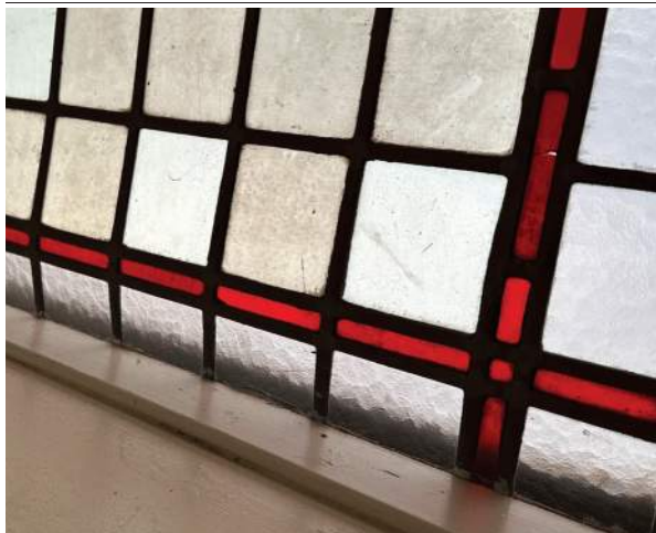
A33 - REPAIR STAINED GLASS WINDOWS
