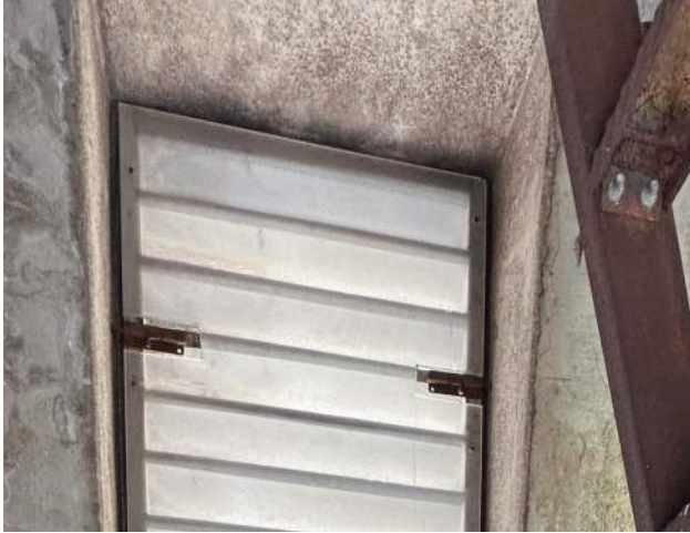
Bell Tower louvers are typically slatted wood screens held in place by throw bolts. They do not resist weather.
