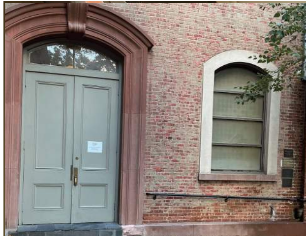
Parish Hall entry doors are solid wood, operate soundly, and have functional hardware.
