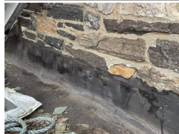
A15-1 - REPLACE PARISH HALL ROOFING MEMBRANE AT FLAT ROOF
