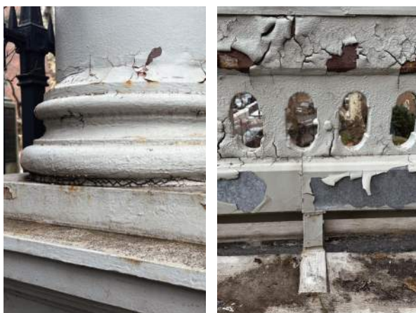
A12-1 - REPAIR AND REFINISH CAST IRON PORTICO
