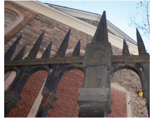
A20 - REFINISH METAL PORTION OF SITE FENCE
