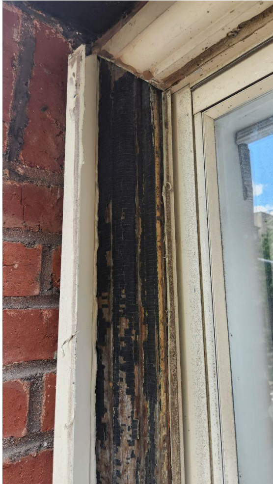
EXISTING WINDOW PROBES - BLACK WINDOW FINISH BASED ON PROBE, PENDING ANALYSIS RESULT
