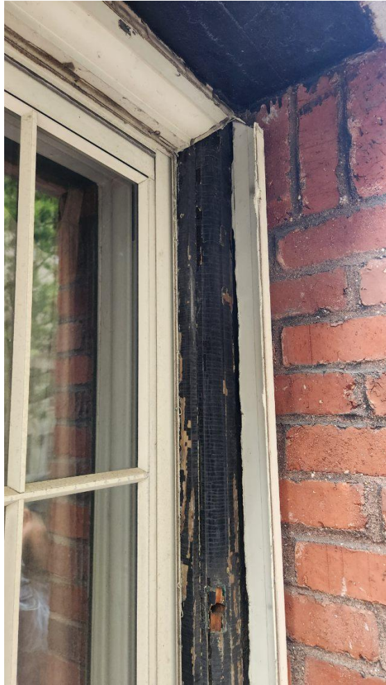
EXISTING WINDOW PROBES - BLACK WINDOW FINISH BASED ON PROBE, PENDING ANALYSIS RESULT
