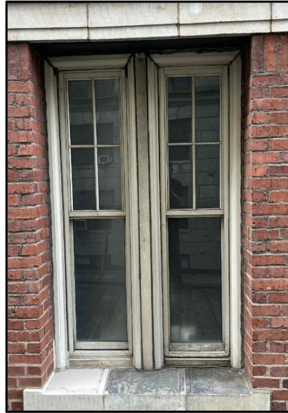
NORTH ELEVATION – EXISTING CONDITION TYPE 'C'
