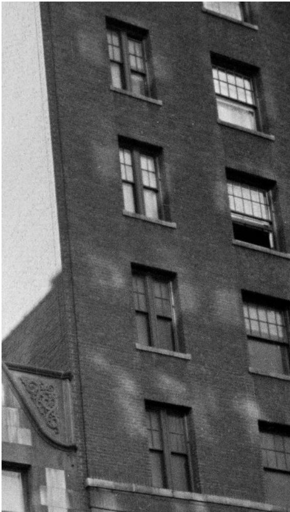
HISTORIC WINDOW TYPE "C" CLOSE UP
