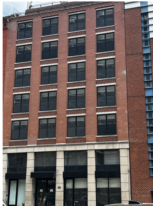
CURRENT WEST PRIMARY FAÇADE
