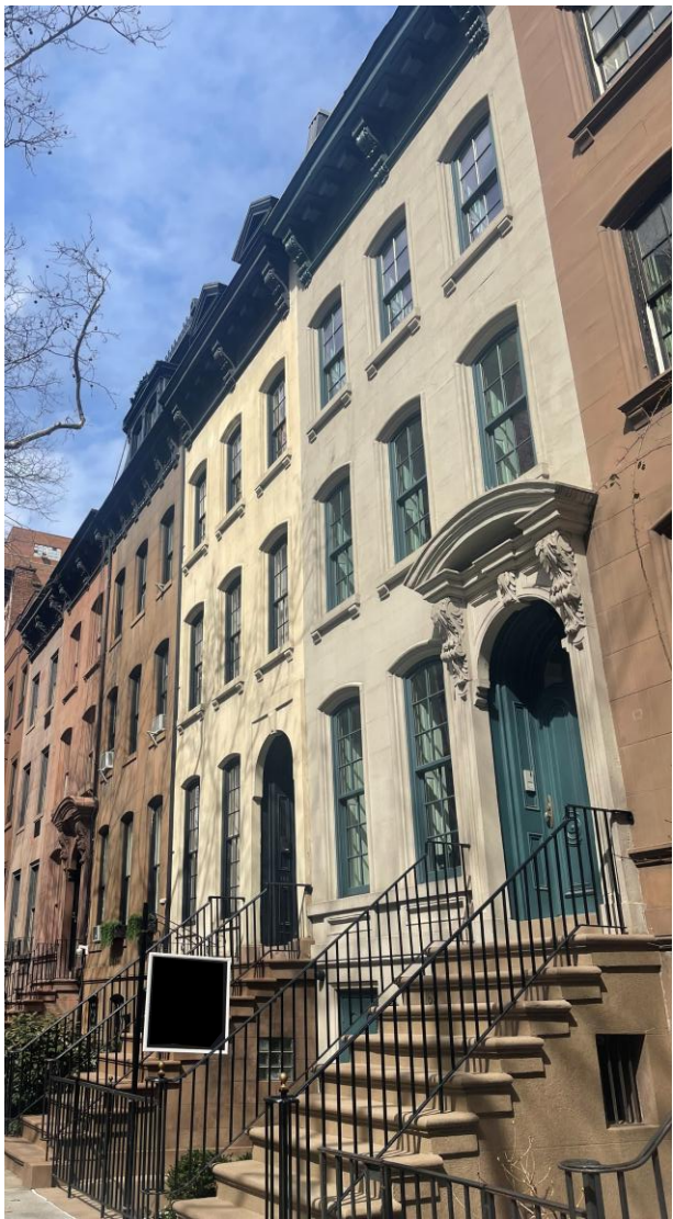
AS BUILT – SOUTH STREET FAÇADE
