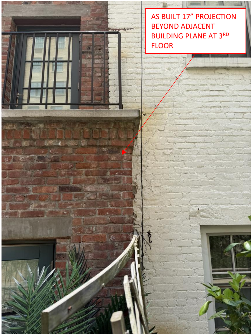
AS BUILT – 17” PROJECTION BEYOND ADJACENT BUILDING PLANE
