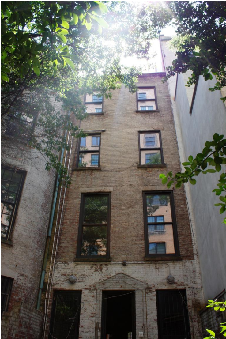
PRE CONSTRUCTION – REAR YARD NORTH ELEVATION
