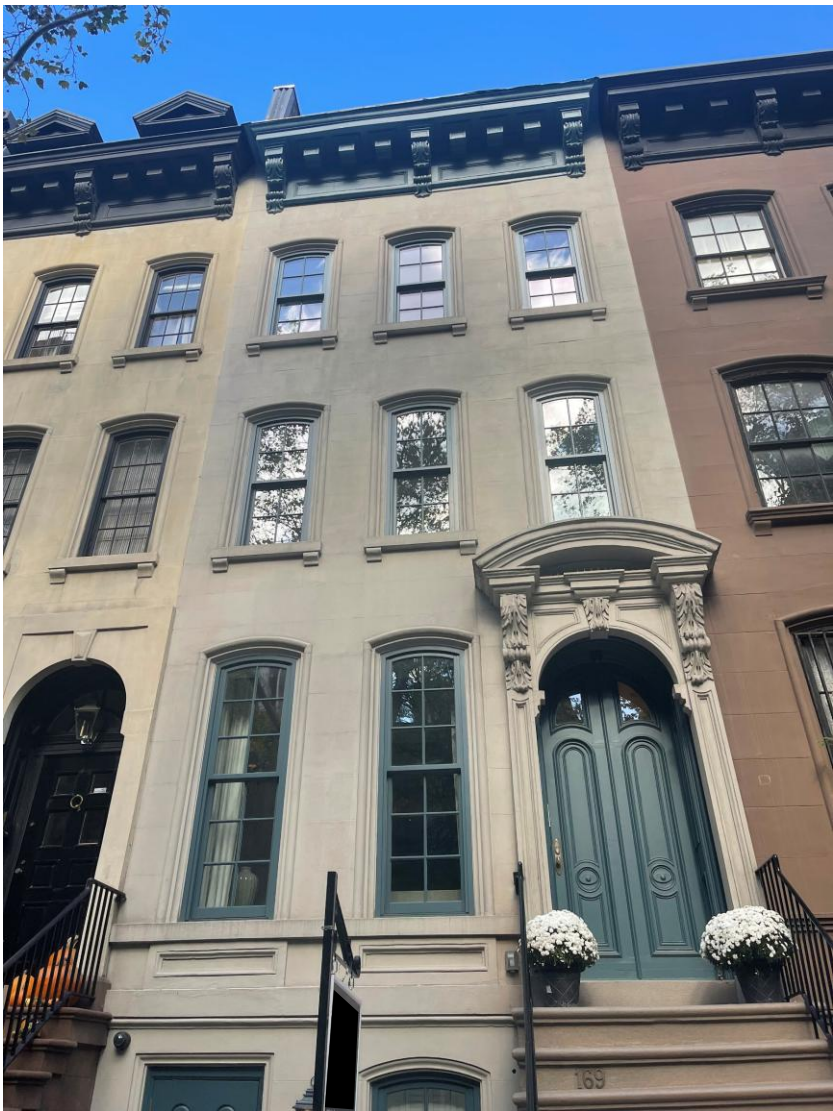
AS BUILT – SOUTH STREET FAÇADE
