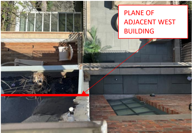
AS BUILT – LOOKING DOWN FROM UPPER ROOF
