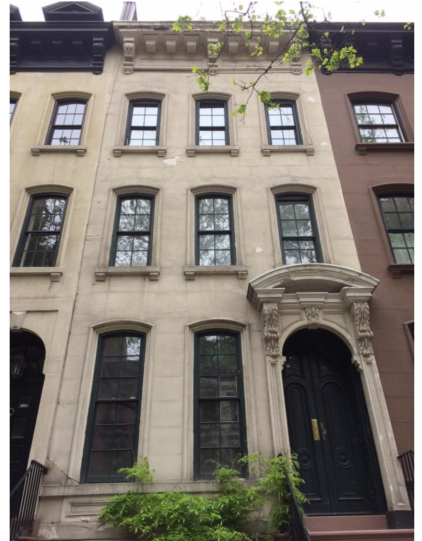
PRE CONSTRUCTION – SOUTH STREET FAÇADE
