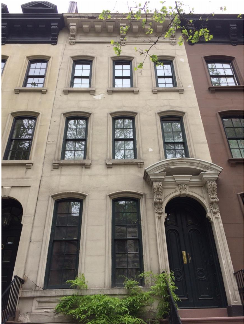
PRE CONSTRUCTION – SOUTH STREET FAÇADE
