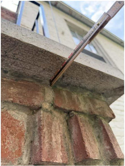
AS BUILT – 3” COPING OVERHANG
