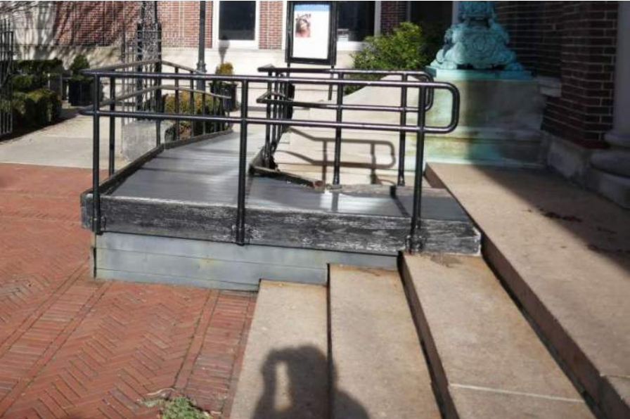
EXISTING RAMP & RAILING
