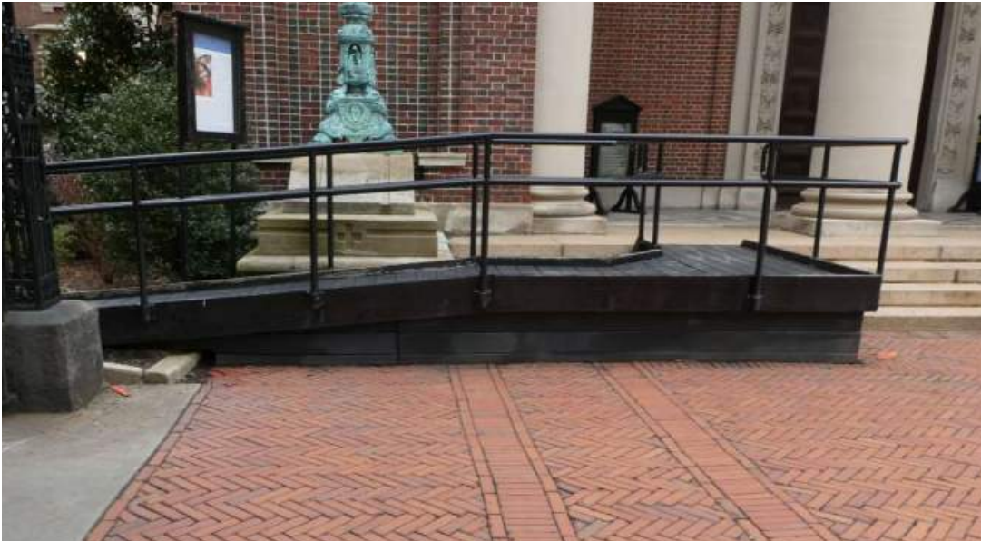
EXISTING RAMP & RAILING
