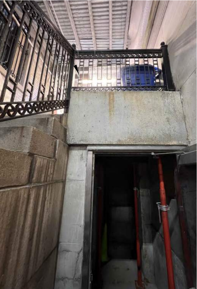
EXISTING STAIR & GUARDRAIL
