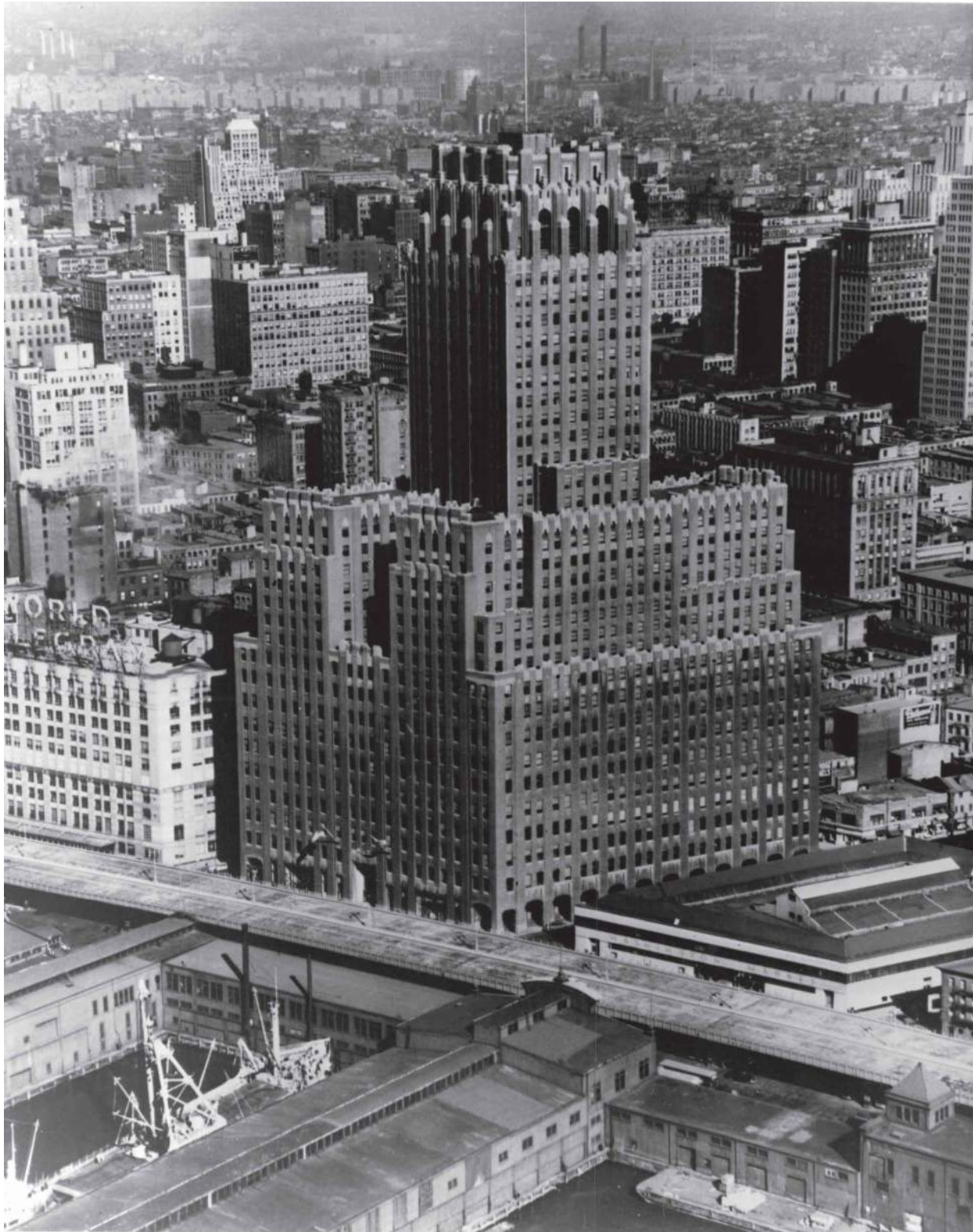
THE BARCLAY-VESEY BUILDING, VIEW FROM SOUTHWEST CORNER, C.1960?
