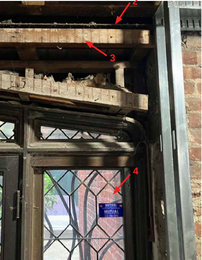
PHOTO OF EXISTING LINTEL FROM INTERIOR
