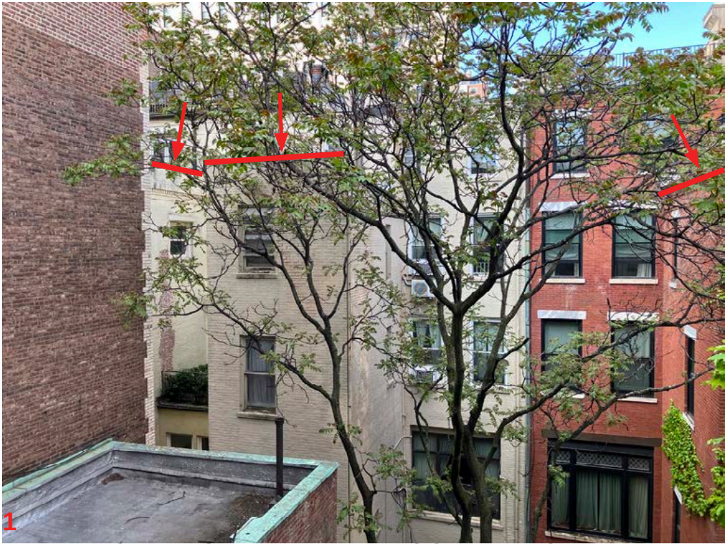
VIEW FROM EXIST REAR 4TH FLOOR WINDOW
