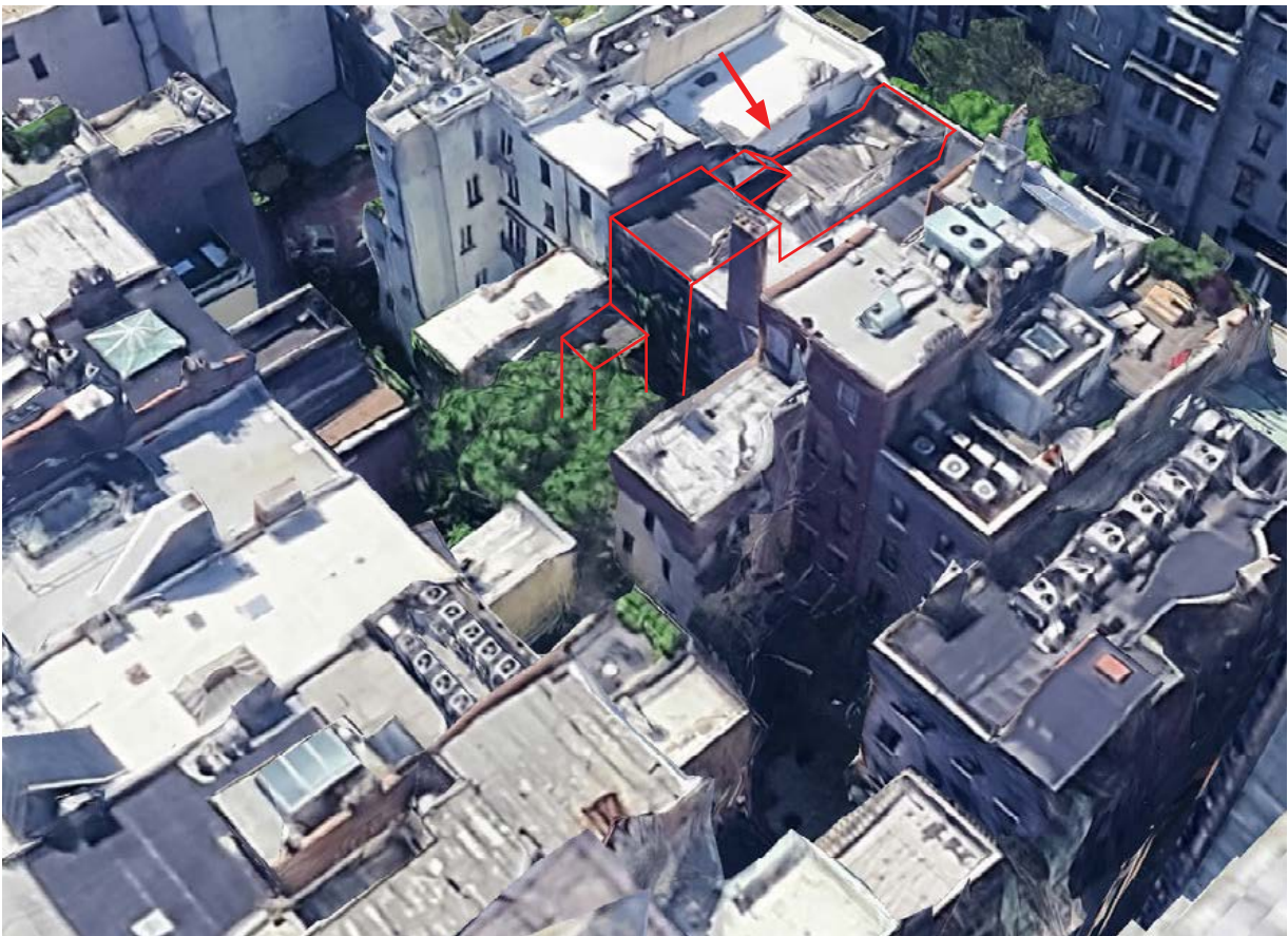
GOOGLE EARTH VIEW (FROM REAR)
