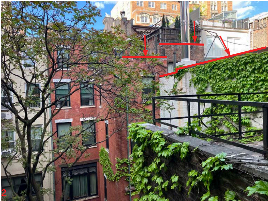
VIEW FROM EXIST REAR 4TH FLOOR WINDOW
