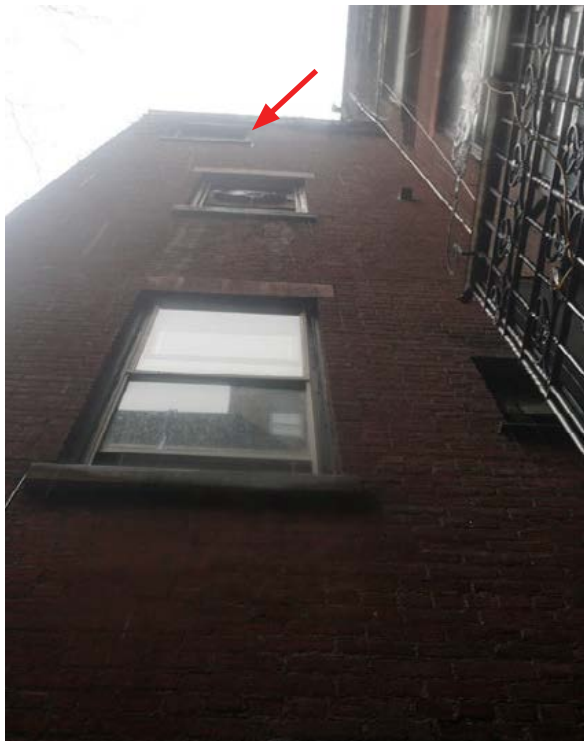
PHOTO OF EXISTING WINDOW FROM EXTERIOR
