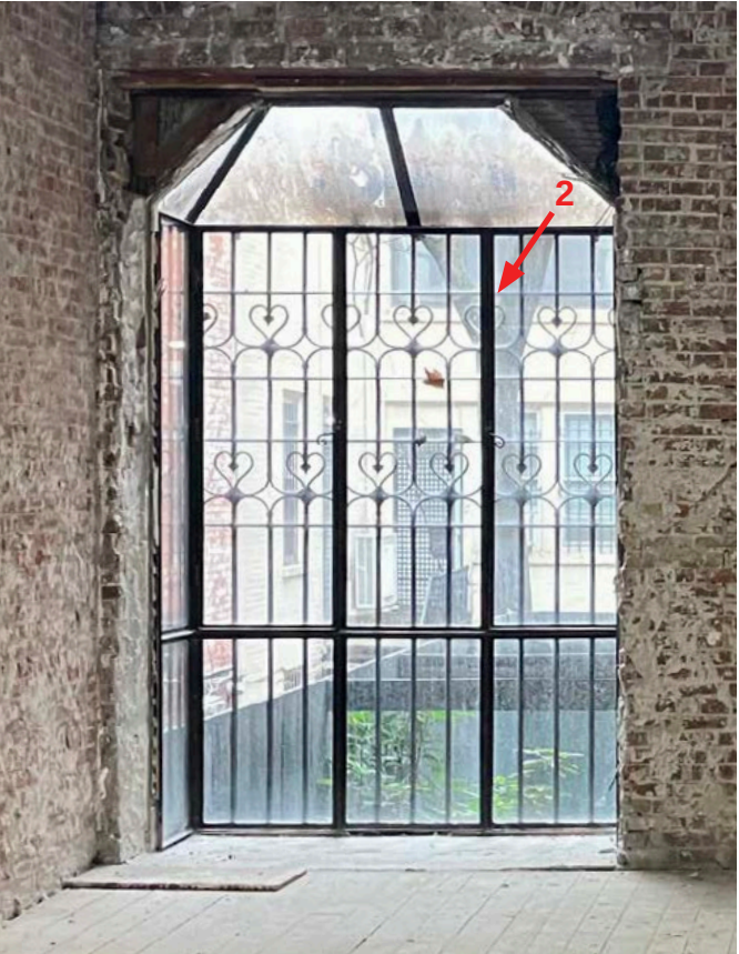
PHOTO OF EXISTING FROM INTERIOR
