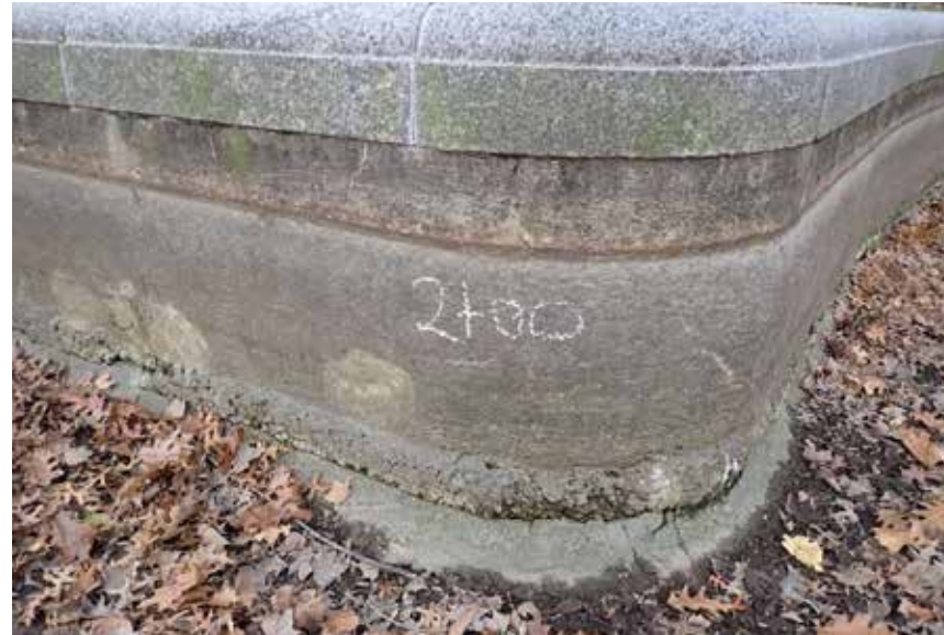
Early 20th Century Concrete Walls
