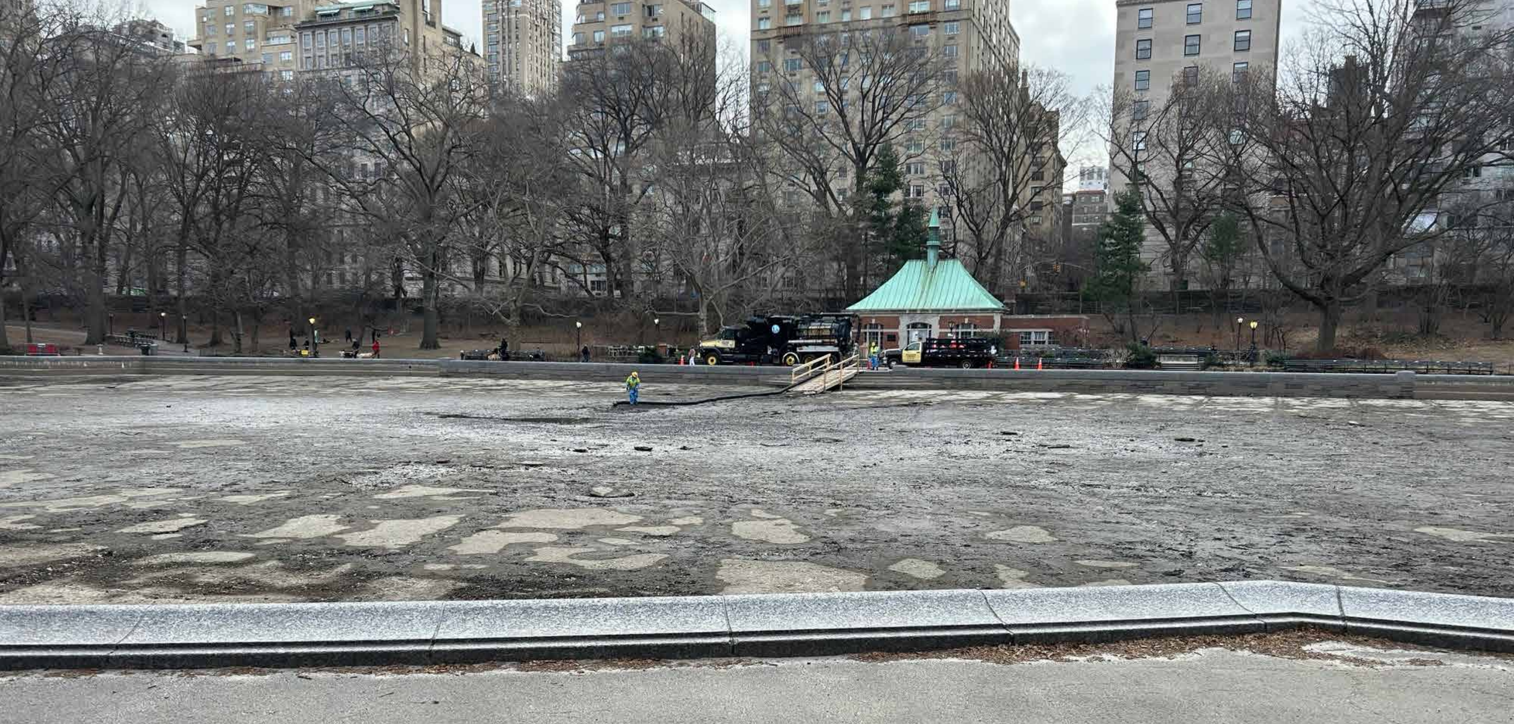
Conservatory Water Basin Floor, Existing Condition (Winter 2024)
