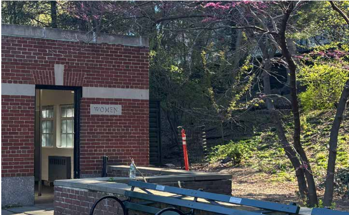
EXISTING CONDITION - INTERIOR OF WOMEN'S RESTROOM EXPOSED, VISIBLE FENCING AT BACK
