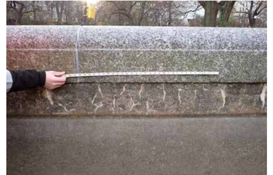
CPC Replacement Concrete Walls
