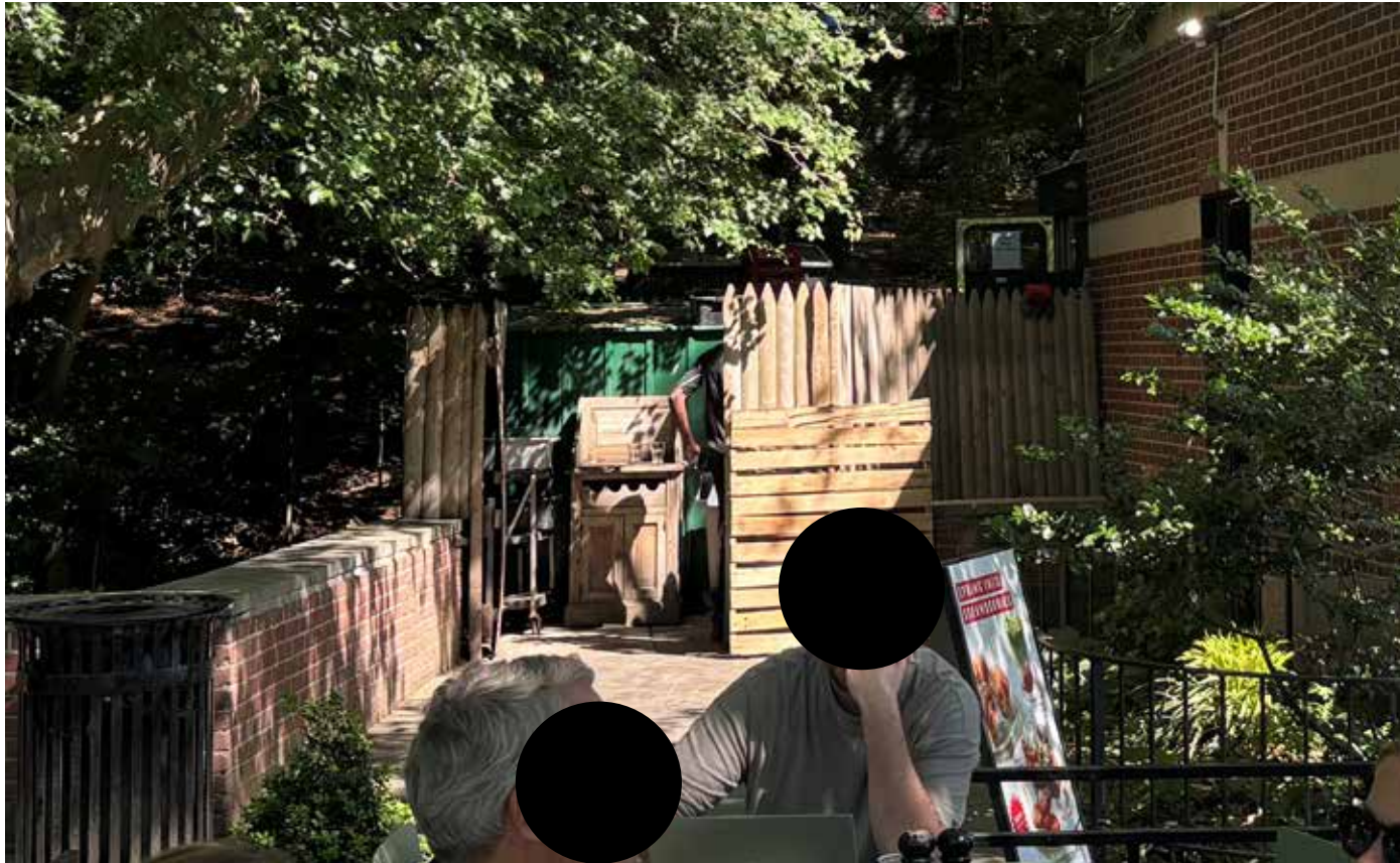
EXISTING CONDITION - WOOD PICKET FENCE, EXPOSED STORAGE CONTAINERS AND EQUIPMENT
