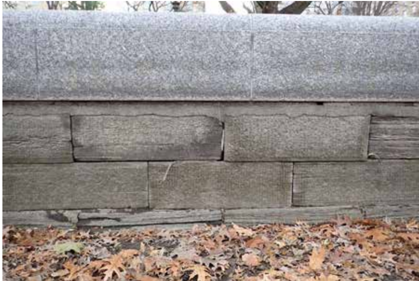
Masonry Block Walls
