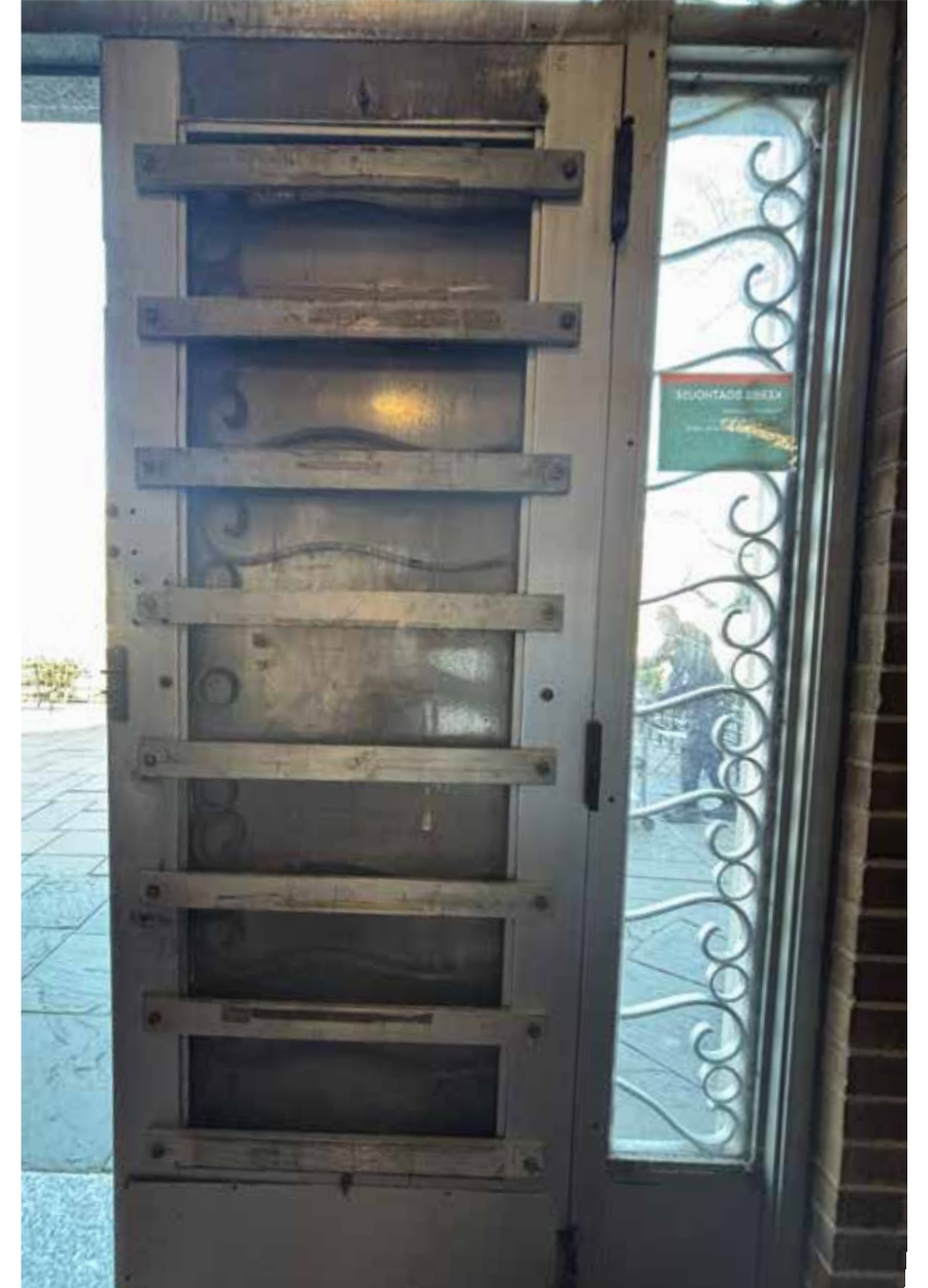
Hidden historic detail elements to be salvaged, reused and used as amold to recast missing detail elements
