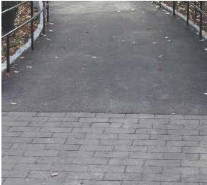
Landing at Accessible Path Rectangular Asphalt Block Paver
