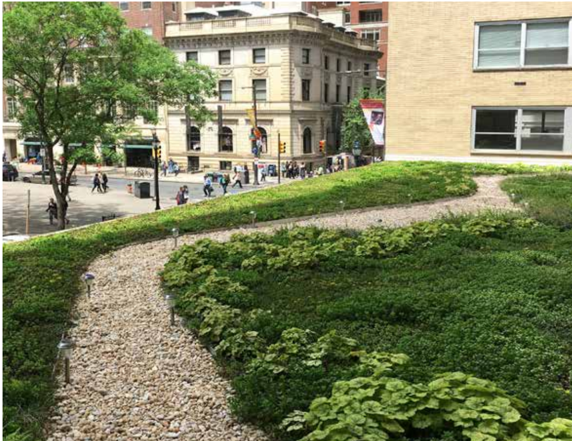
Precedent Image | Rittenhouse Claridge Lobby roof retrofit, Philadelphia, PA Low lying planting profile, sedum and shade loving perennials
