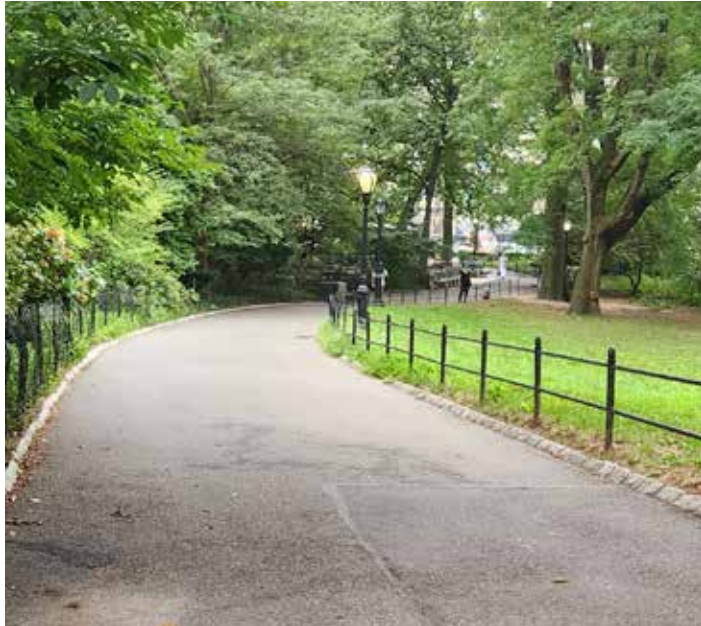
Asphalt Paving with Sloping Granite Block Curb
