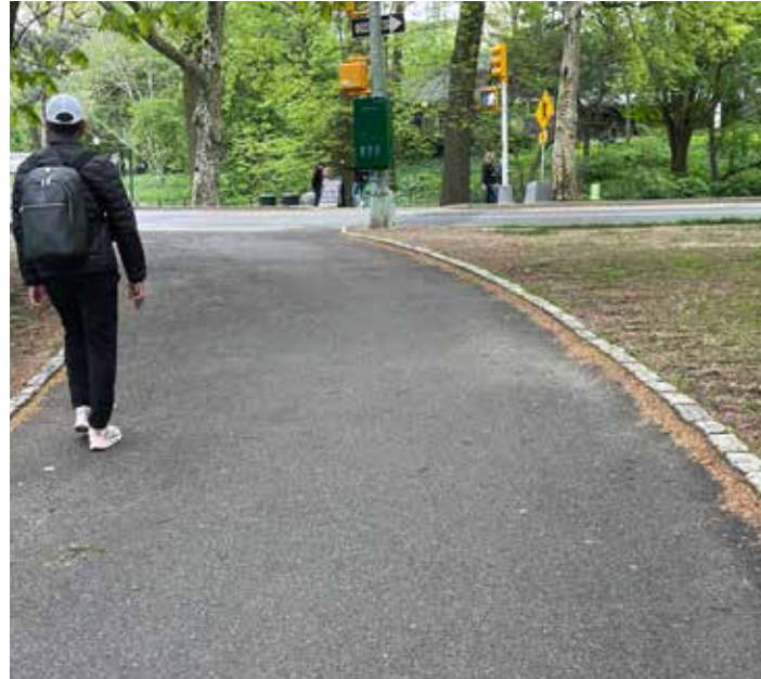
Asphalt Paving with Vertical Granite Block Curb
