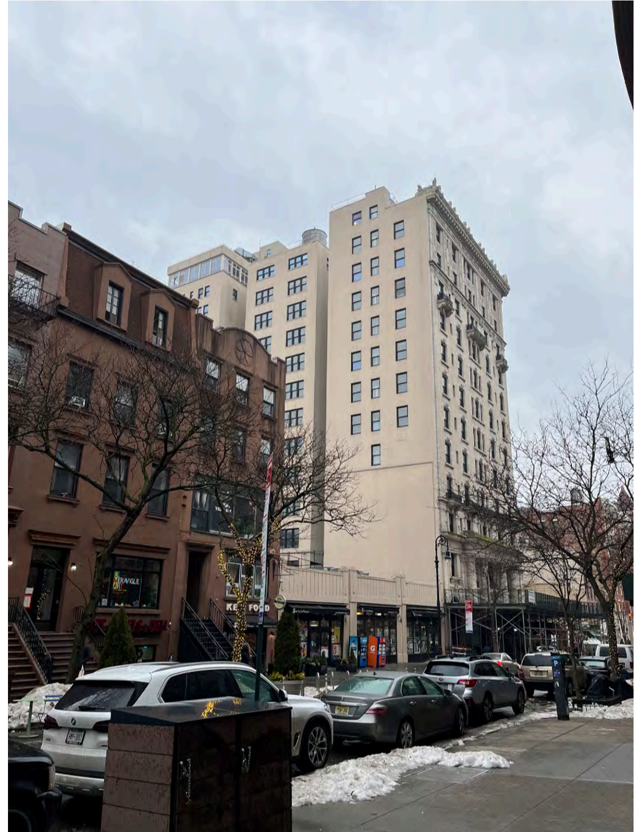
View to rear facade from east on Montague Street
