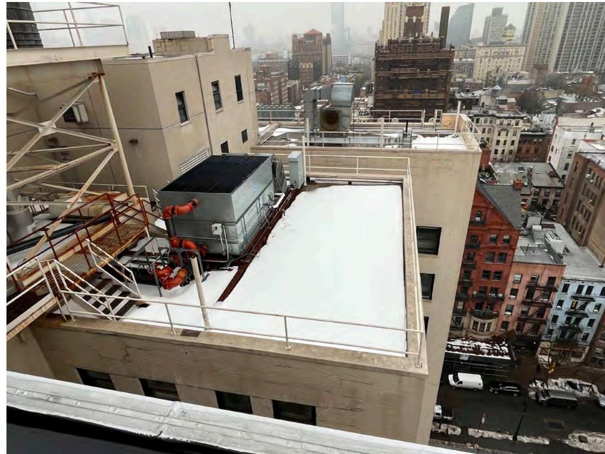
View to north from roof
