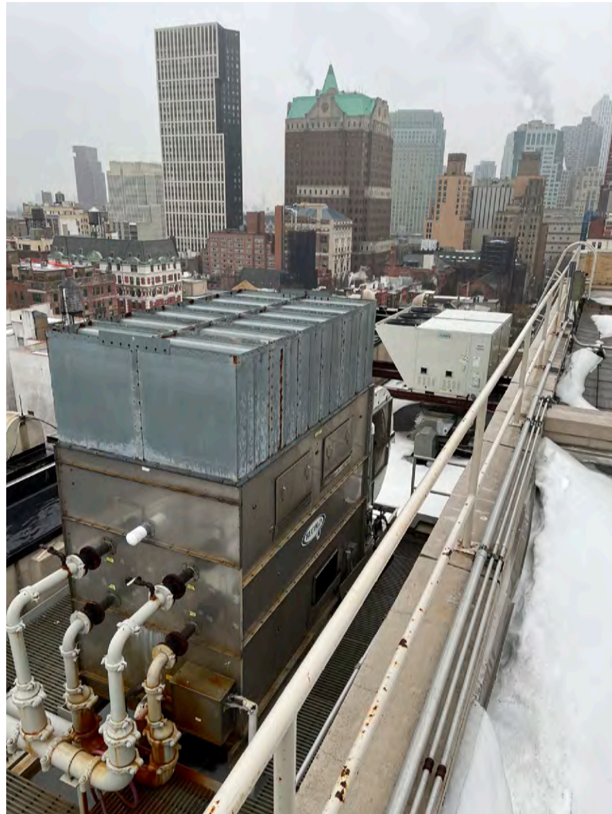
View to east from 14th floor addition terrace
