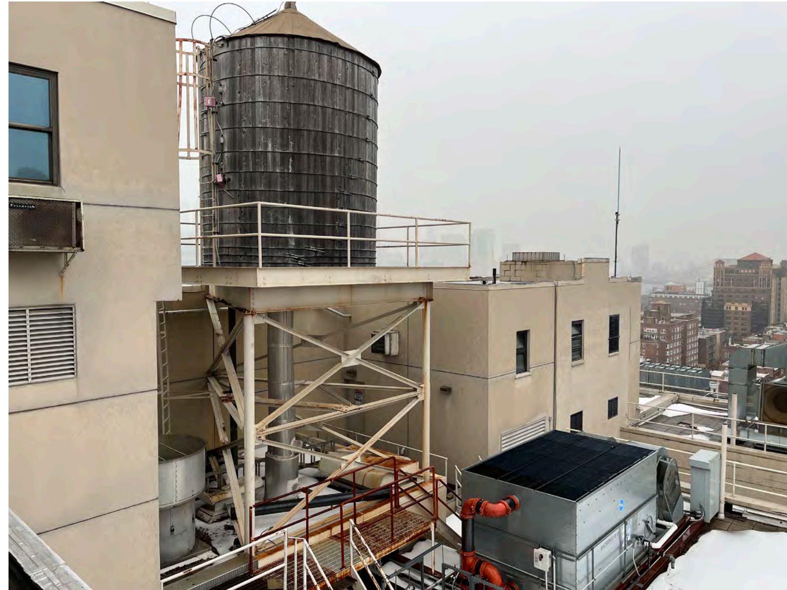
View to north from roof
