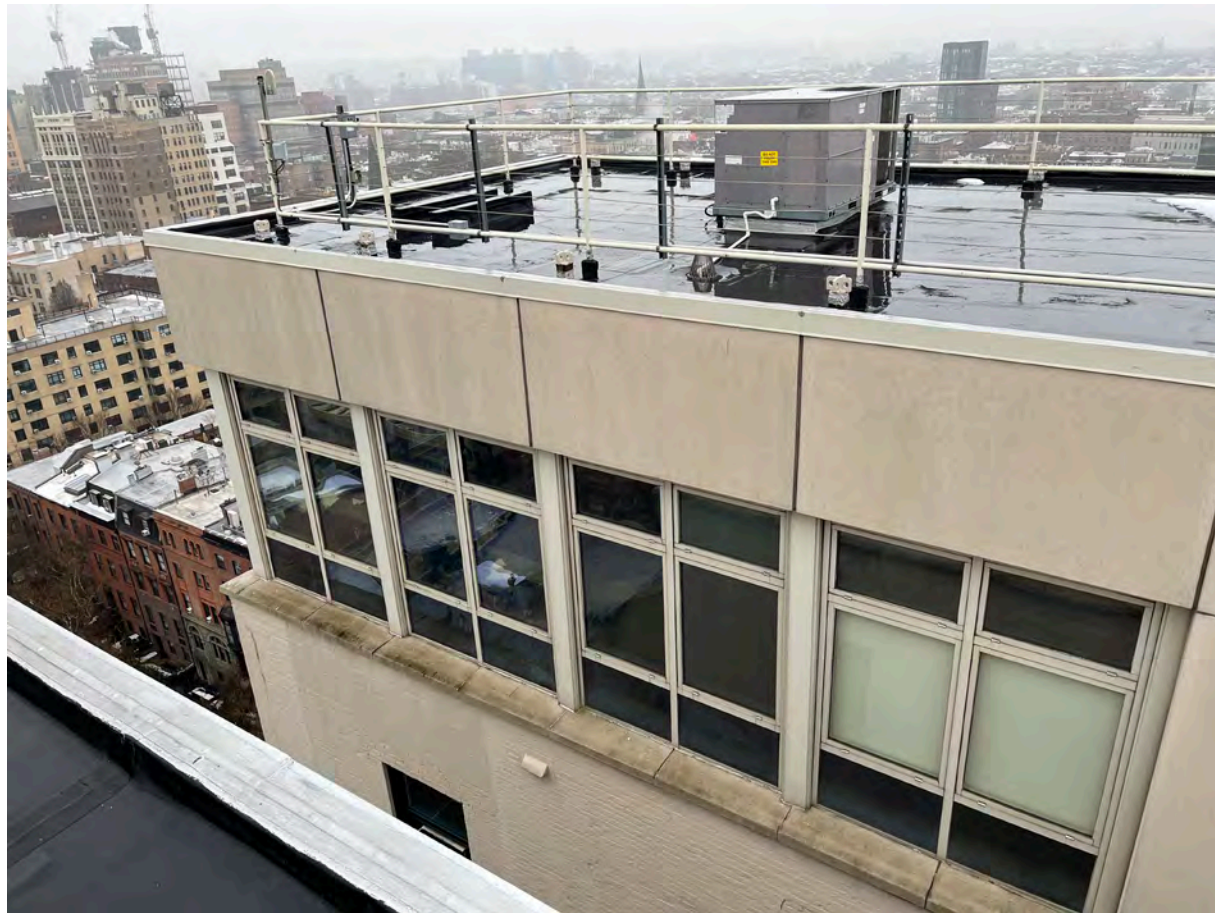
View to southeast from roof
