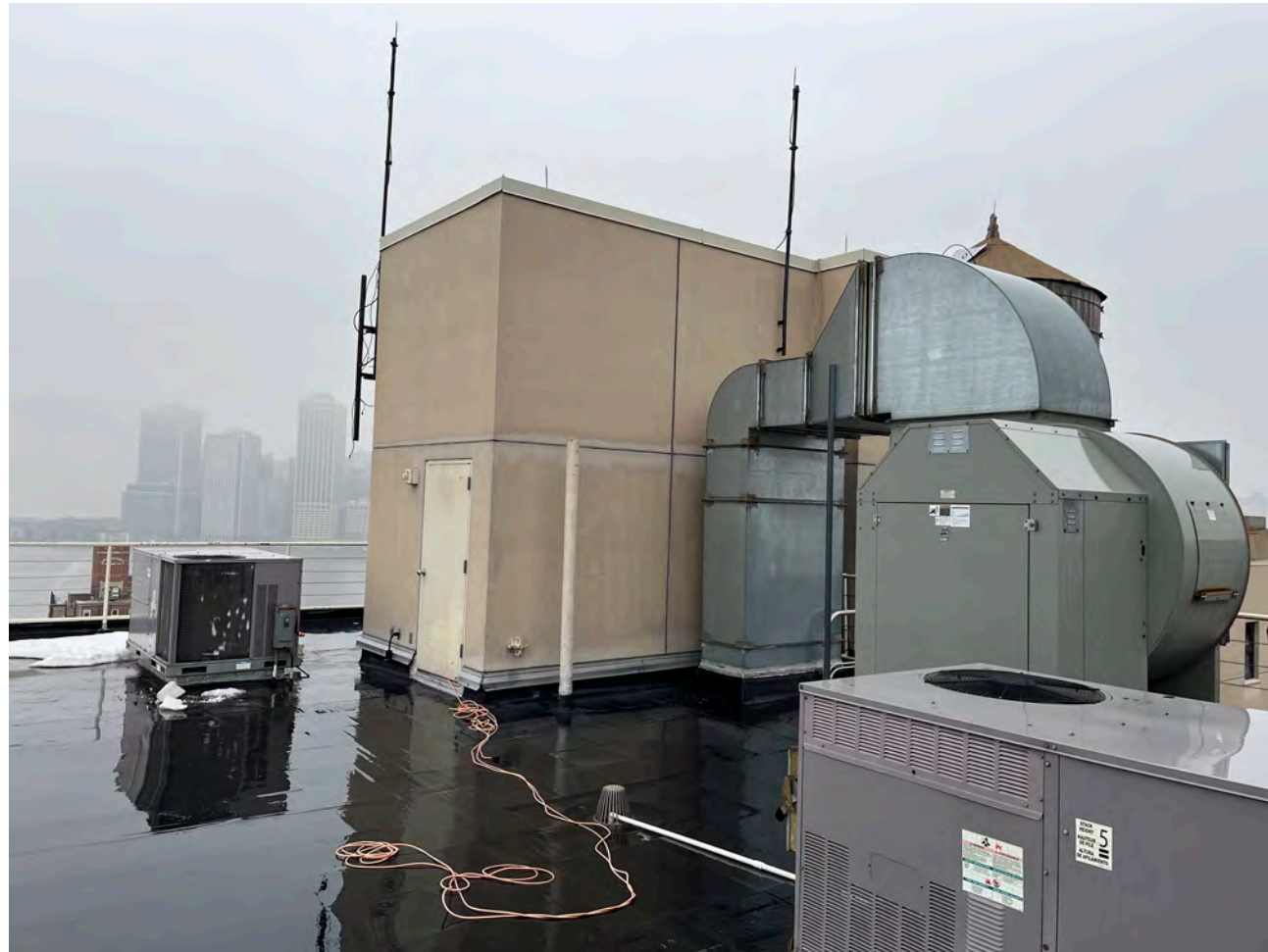
View to west at roof
