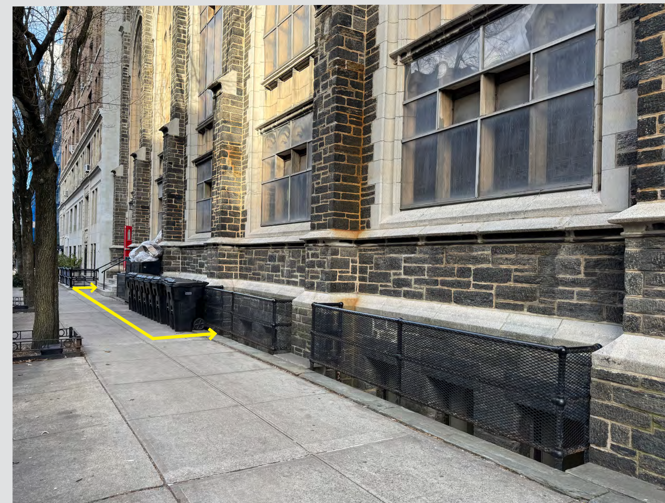
③ W.114TH ST. VIEW TOWARD THE WEST; RAMP IS PROPOSED TO BE LOCATED ALONG THE 2ND AND 3RD WINDOW BAY, WITH THE LANDING AT THE DOOR;
