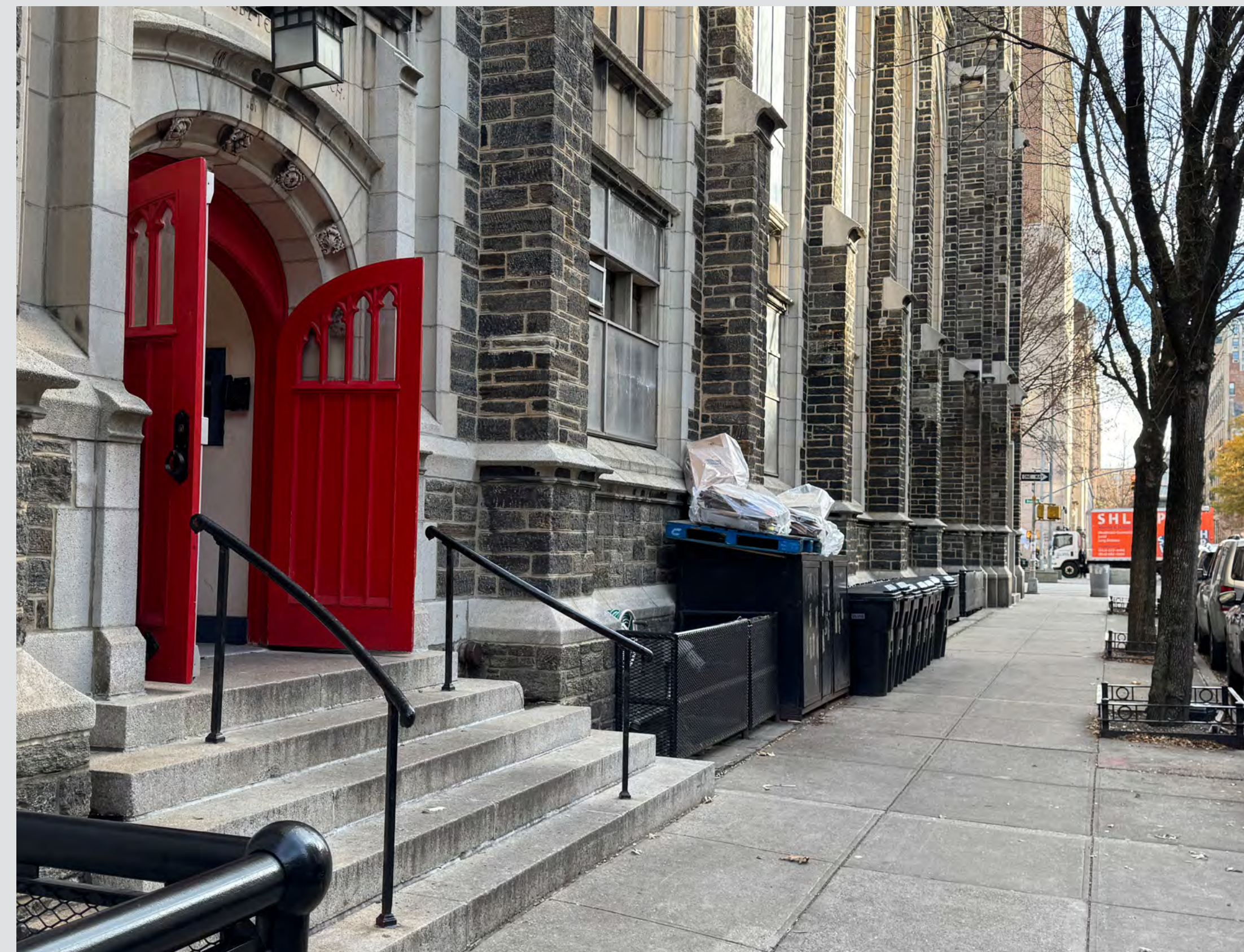
② ACCESSIBLE RAMP IS PROPOSED TO BE LOCATED ALONG THE 2ND AND 3RD WINDOW BAYS, WITH THE LANDING AT THE DOOR; THIS REQUIRES MODIFICATION OF THE EXISTING STAIRS.
