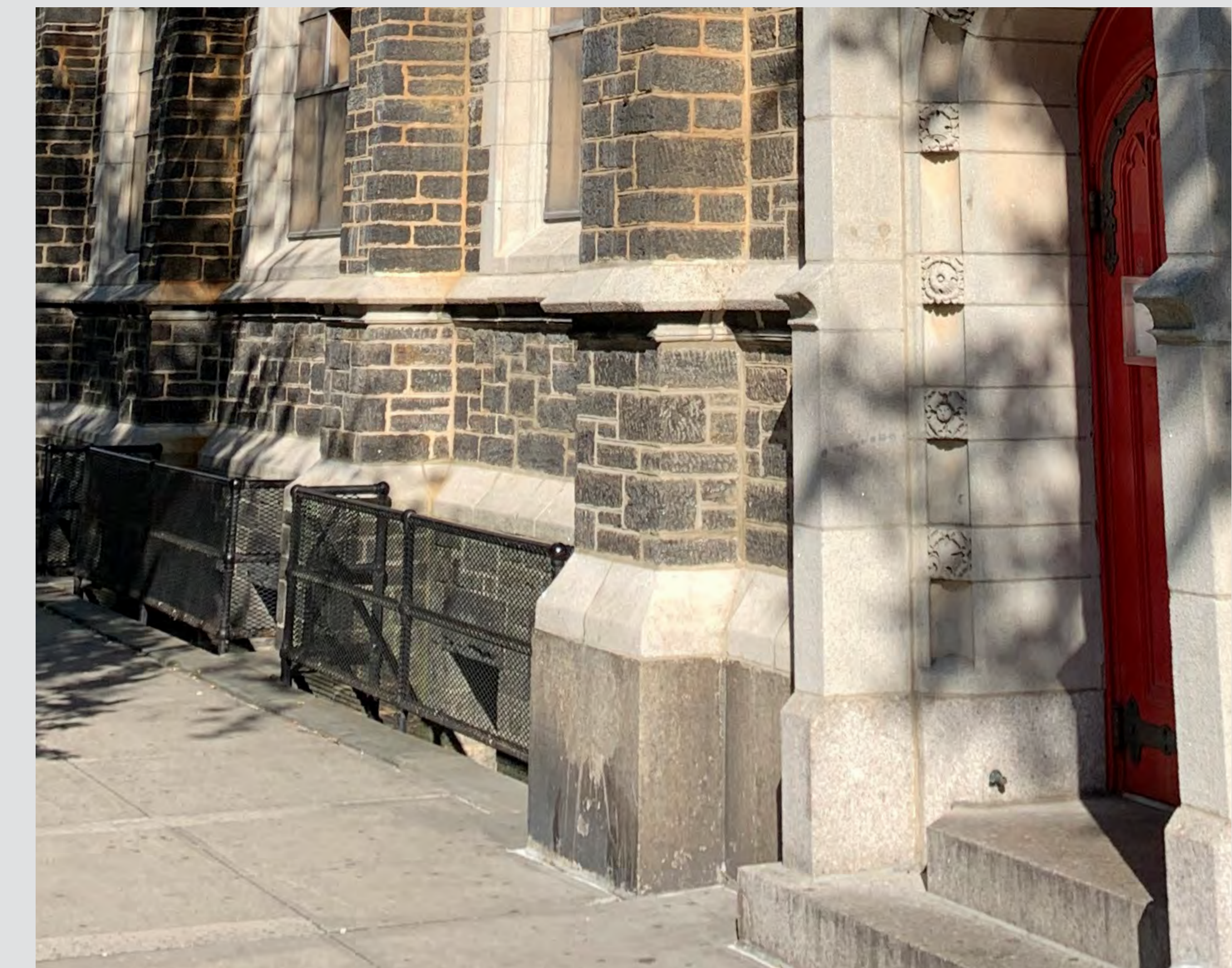
⑥ GRANITE BASE SYSTEM IS PRESENT AT THE CHURCH TOWER AND BROADWAY FRONTAGE. BASES ALONG WEST 114TH STREET ARE SCHIST MEETING THE SIDEWALK.
