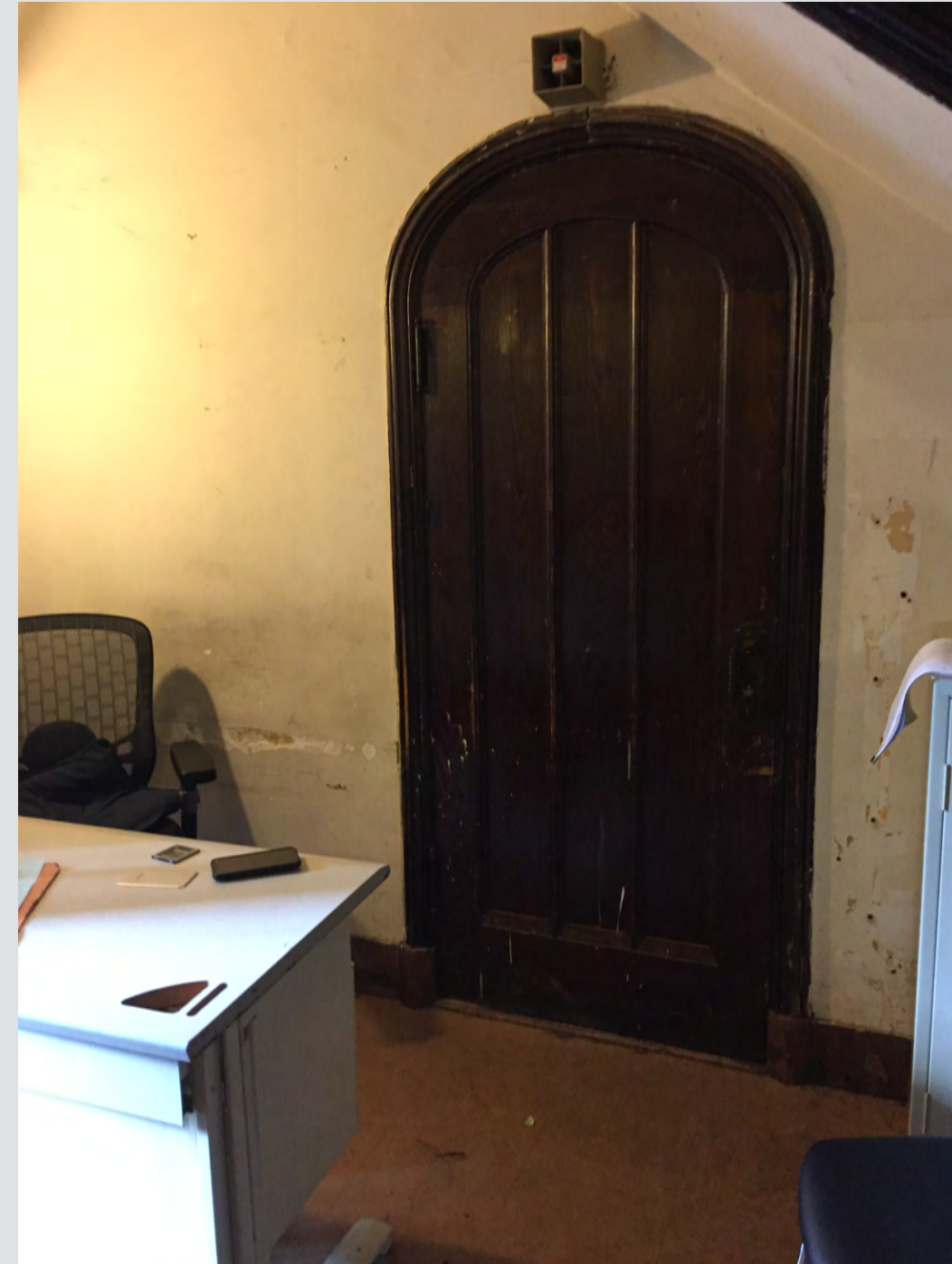
③ DOOR FROM THE TOWER TO SOUTH NAVE OF THE CHURCH. THERE ARE TWO STEPS AT THE INTERIOR DOOR. MODIFICATIONS TO THE TOWER FLOOR, STEPS AND DOOR ARE REQUIRED.
