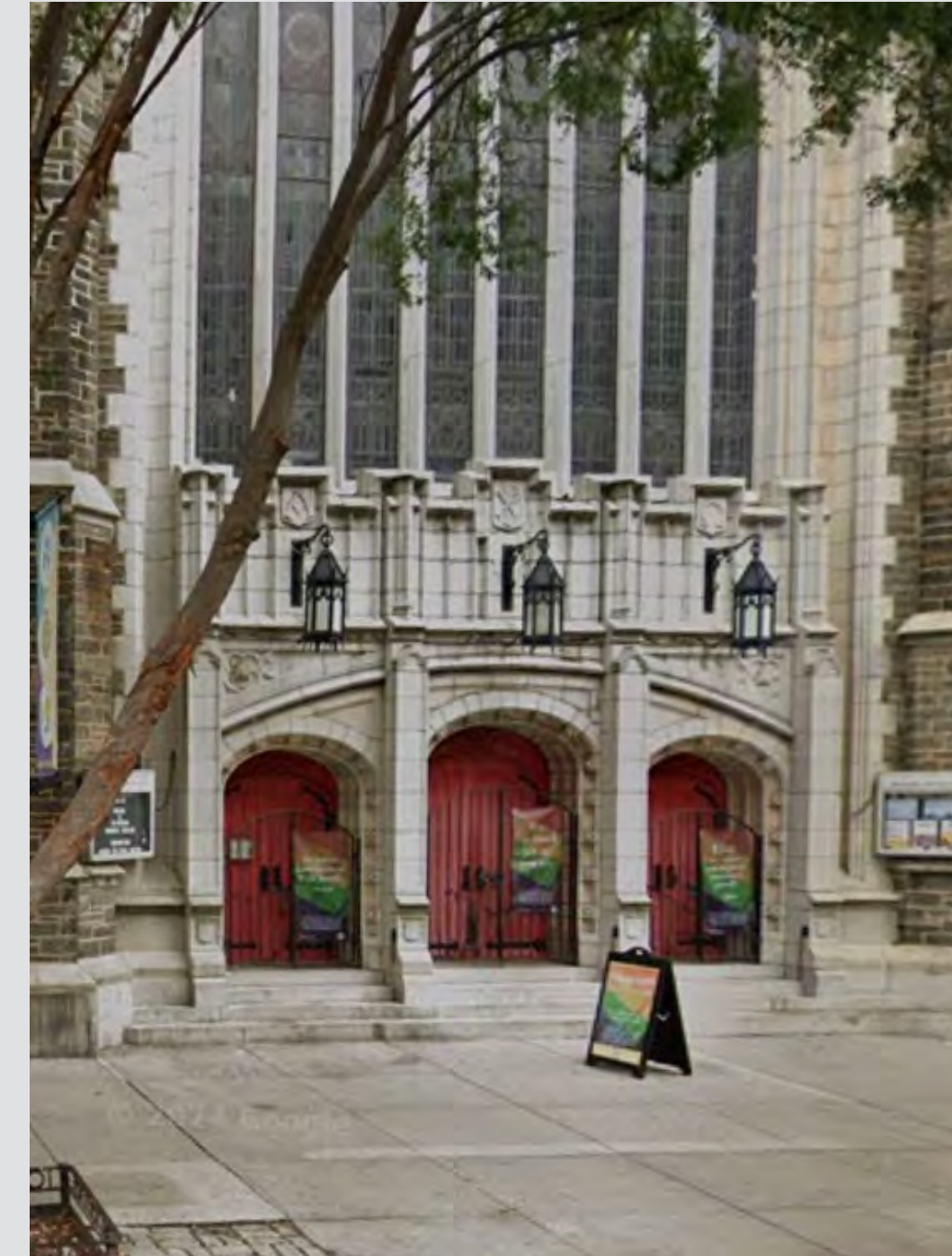
⑤ MAIN ENTRY TO THE CHURCH AND DOOR TO THE TOWER. THERE ARE FOUR STEPS UP FROM THE SIDEWALK AND TWO STEPS DOWN TO THE TOWER. MODIFICATIONS TO THE TOWER FLOOR, STEPS AND DOORS ARE REQUIRED.
