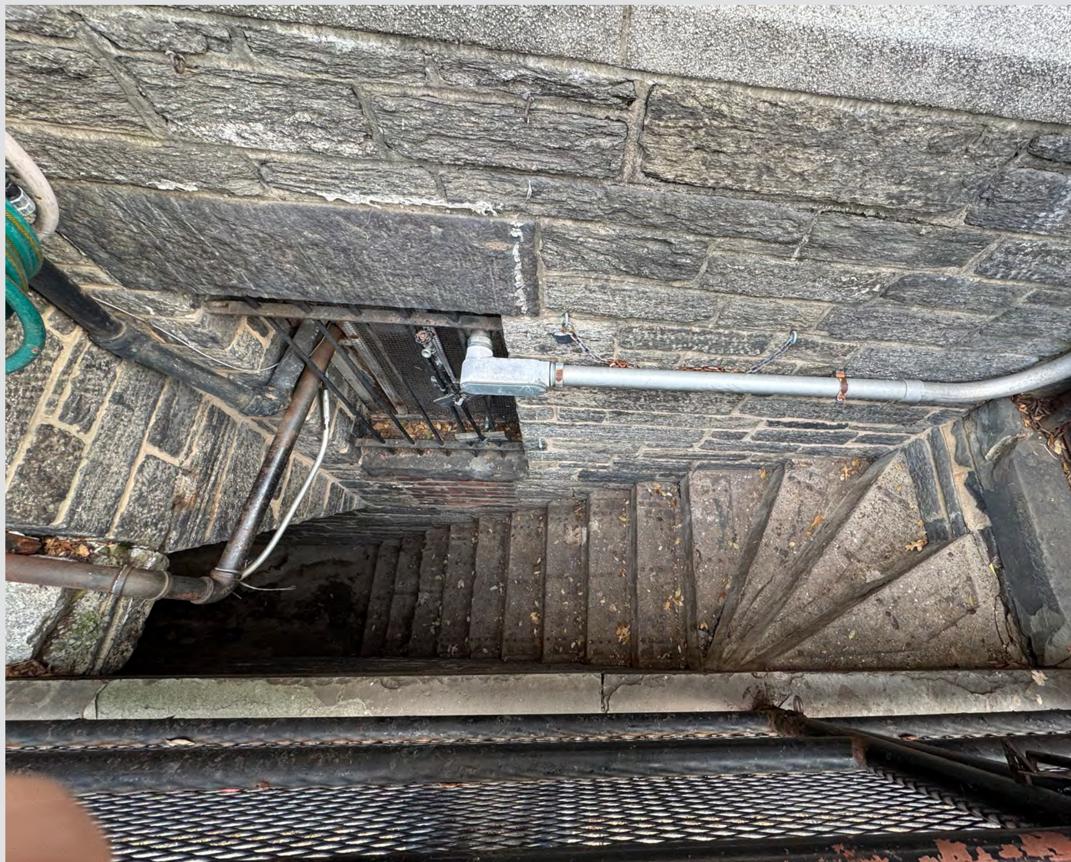
④ THE BASEMENT STAIRS ARE LOCATED AT 2ND WEST WINDOW BAY. THEY LEAD TO THE KITCHEN SERVICE AREA AND ARE ALSO SERVING AS AN EXIT. THE PROPOSED RAMP HAS TO CLEAR THESE STAIRS.
