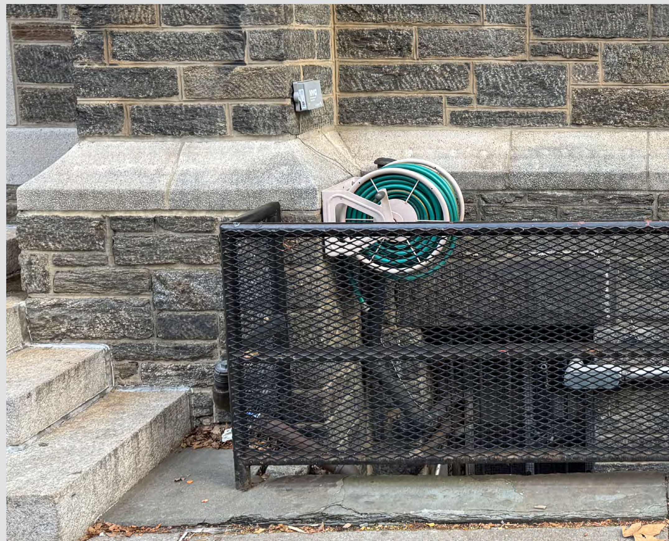
④ DETAIL OF BUILDING BASE AT AT WEST 114TH STREET: GRANITE STEPS, SCHIST WALLS MEETING THE SIDEWALK LEVEL, CAST STONE TRIMS. RAILINGS ARE NON-HISTORIC.
