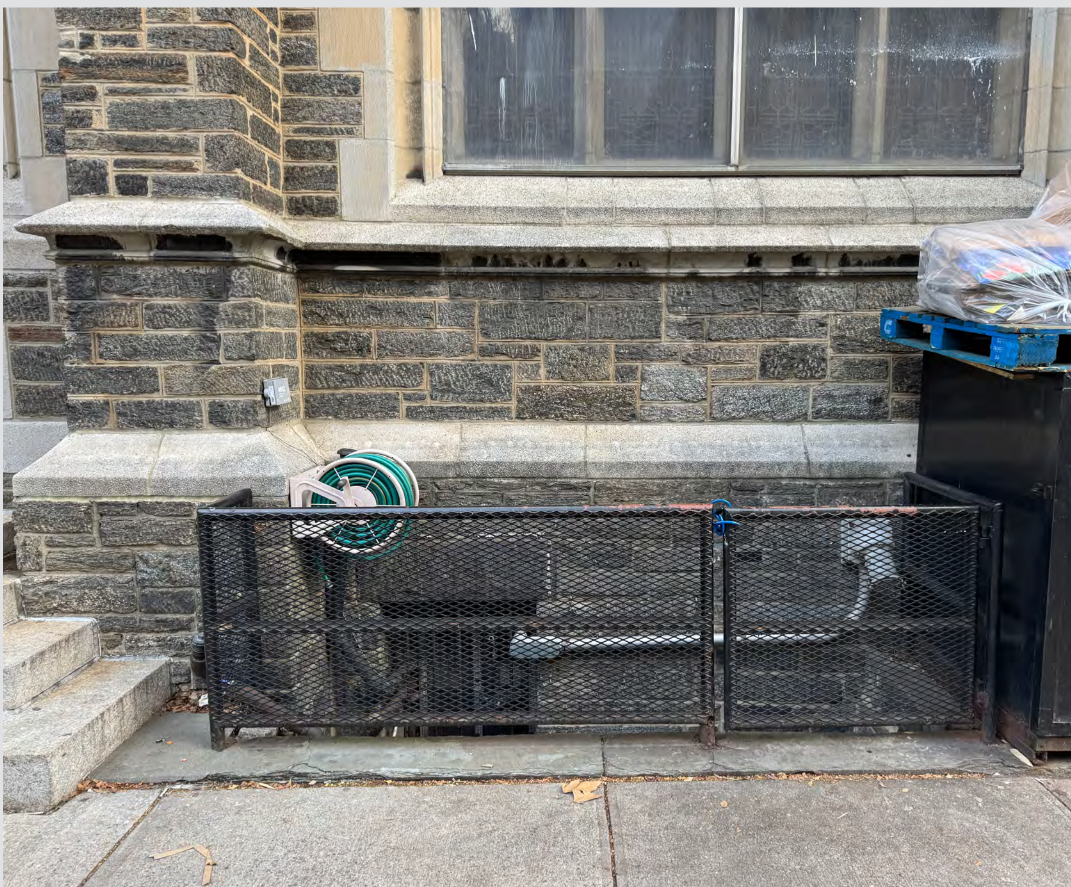
④ THE BASEMENT STAIRS ARE LOCATED AT 2ND WEST WINDOW BAY. THEY LEAD TO THE KITCHEN SERVICE AREA AND ARE ALSO SERVING AS AN EXIT. THE PROPOSED RAMP HAS TO CLEAR THESE STAIRS.
