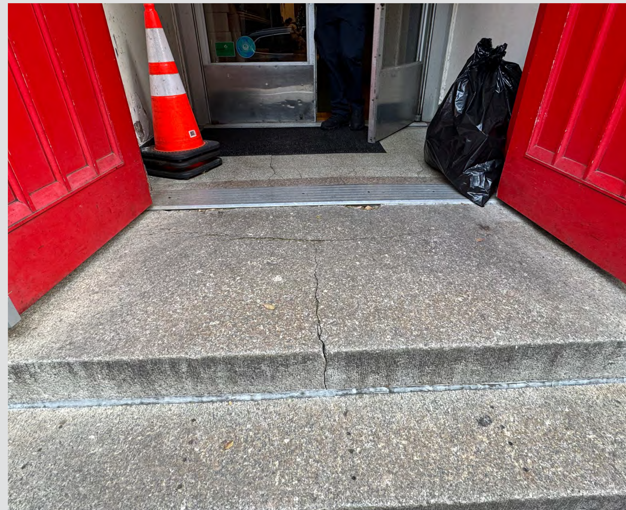
② DETAIL OF GRANITE LANDING AND TERAZZO FLOOR INSIDE.
