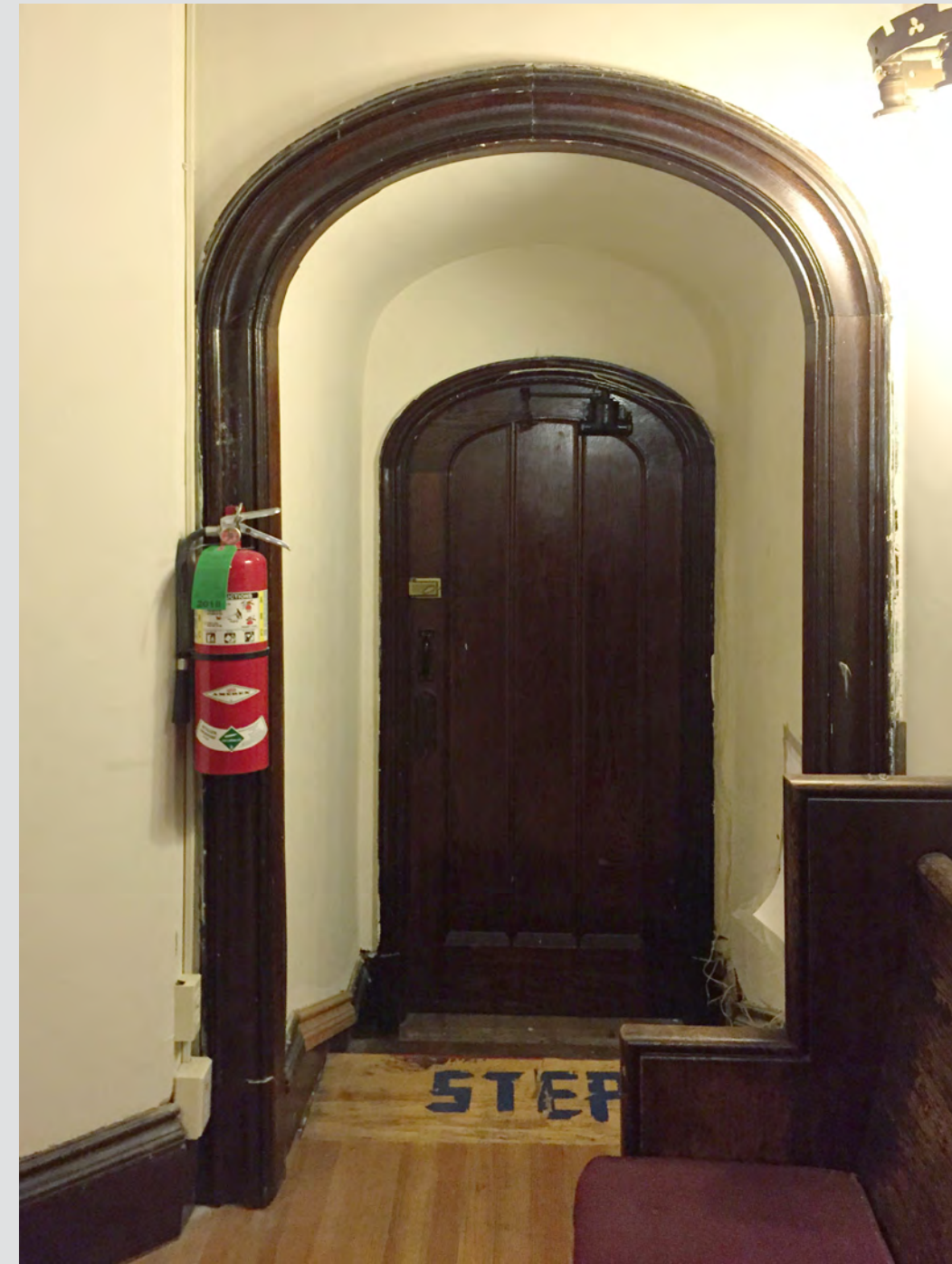
③ DOOR FROM THE TOWER TO SOUTH NAVE OF THE CHURCH. THERE ARE TWO STEPS AT THE INTERIOR DOOR. MODIFICATIONS TO THE TOWER FLOOR, STEPS AND DOOR ARE REQUIRED.
