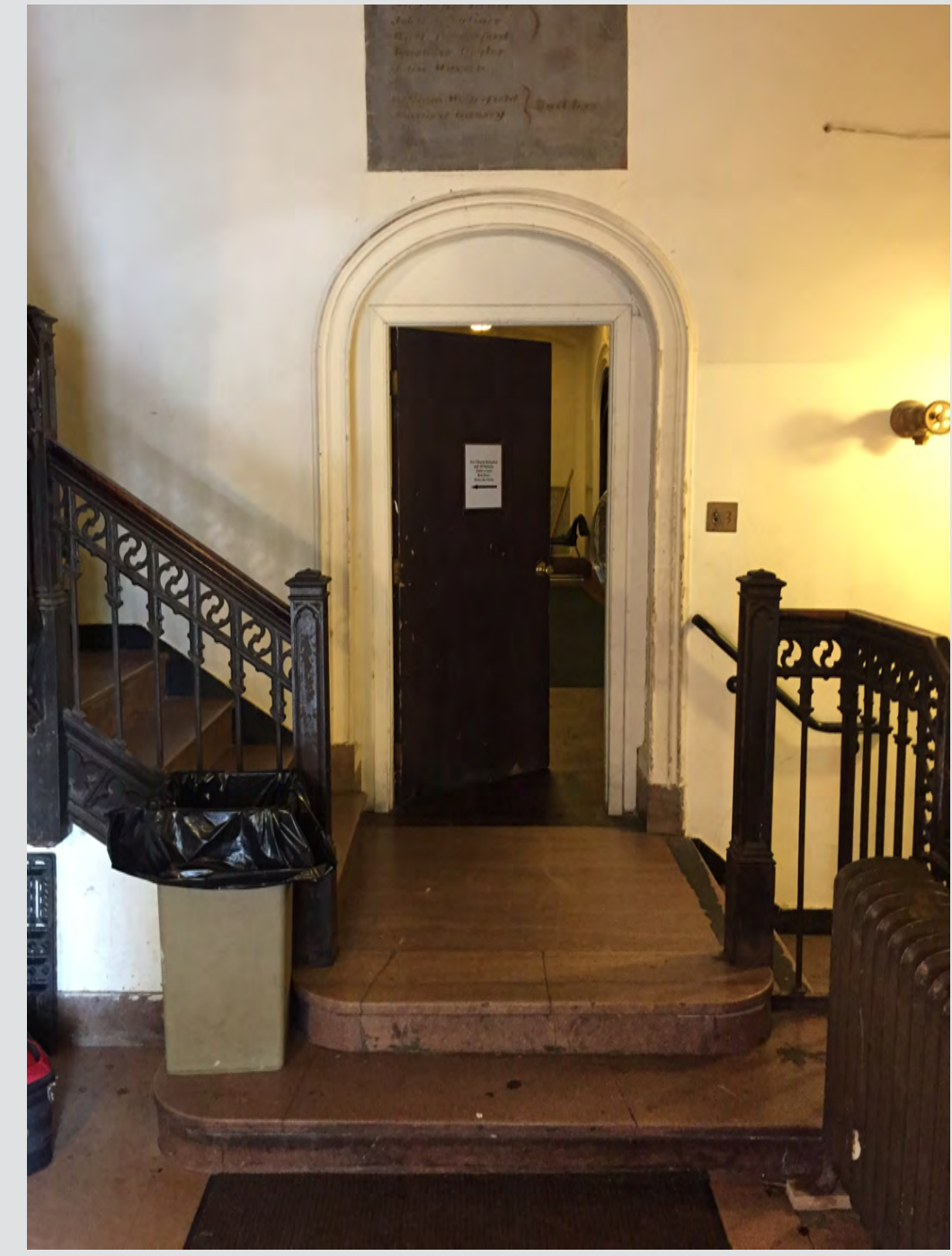
⑤ MAIN ENTRY TO THE CHURCH AND DOOR TO THE TOWER. THERE ARE FOUR STEPS UP FROM THE SIDEWALK AND TWO STEPS DOWN TO THE TOWER. MODIFICATIONS TO THE TOWER FLOOR, STEPS AND DOORS ARE REQUIRED.
