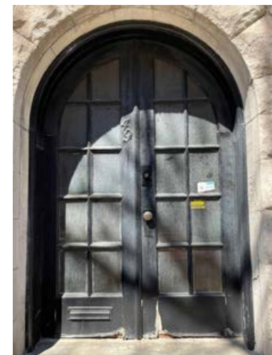
Precedant B 49 St Nicholas Place Replacement wood door with glazing
