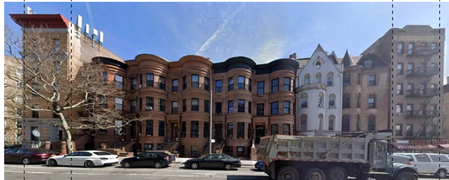
840-856 Saint Nicholas Avenue, Frontal view
