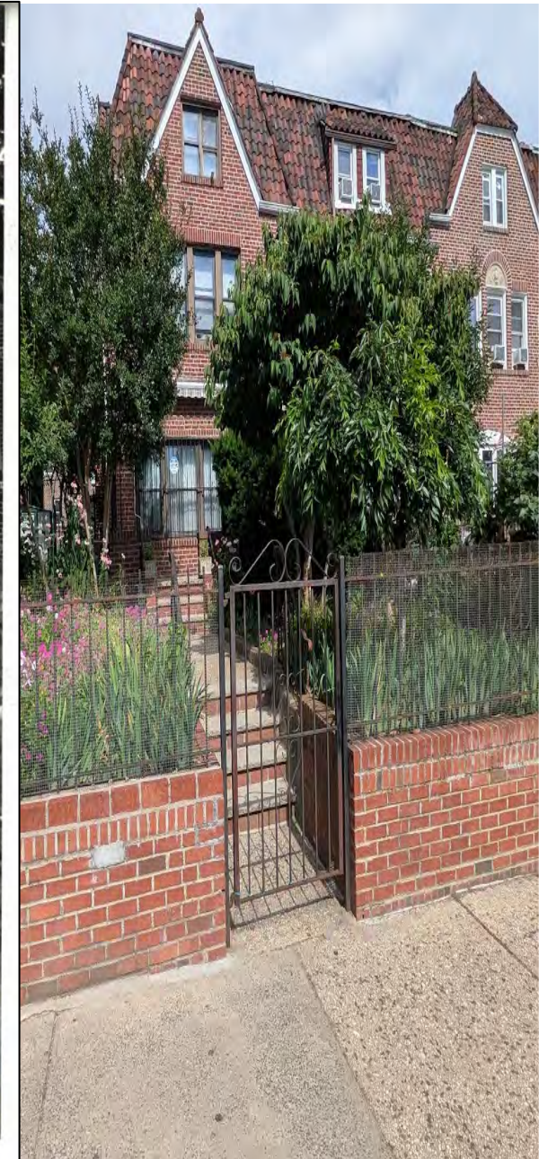
2026 – after alterations made in 2000s
