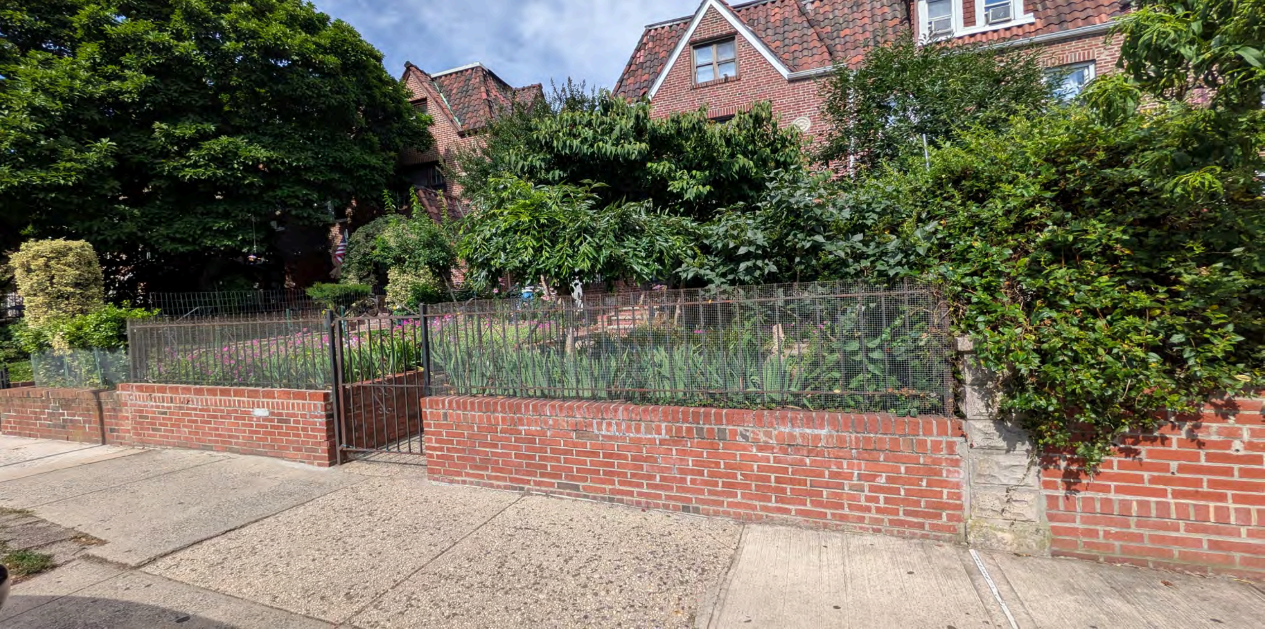
Area Wall next to both neighbors' area walls
