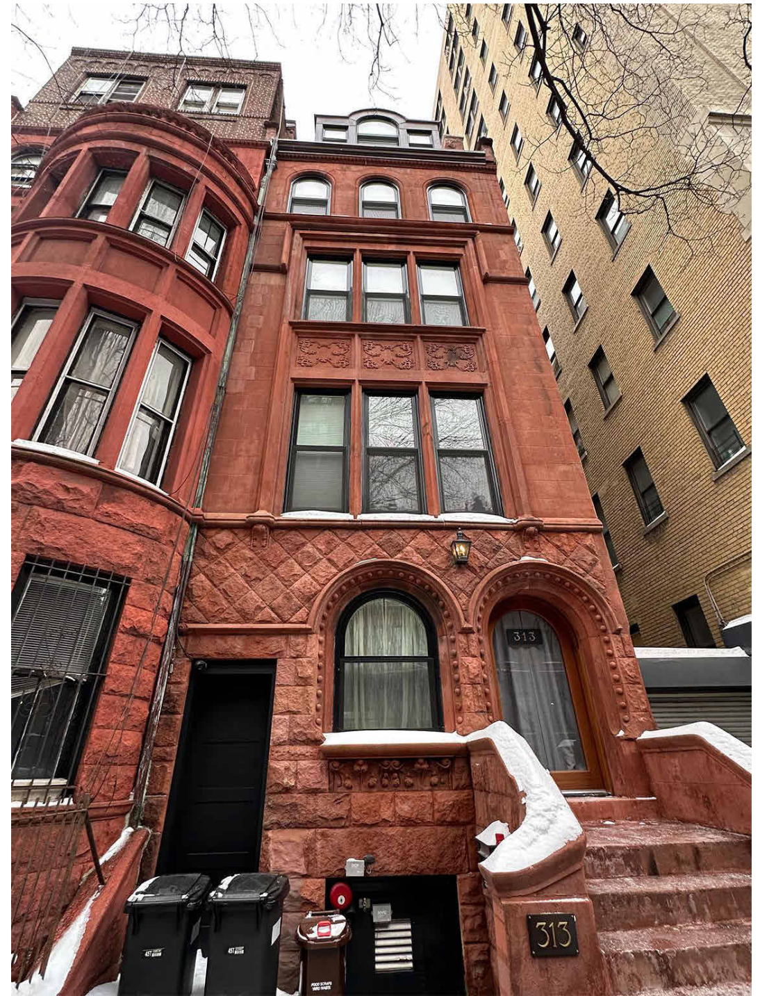
3. ROWHOUSE BLOCK NORTH VIEW -313
