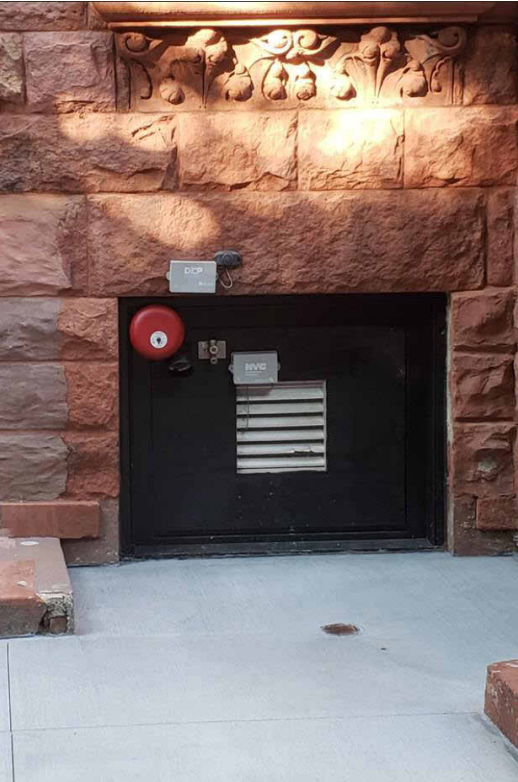
5. VIEW OF EXISTING BASEMENT CLERESTORY OPENING
