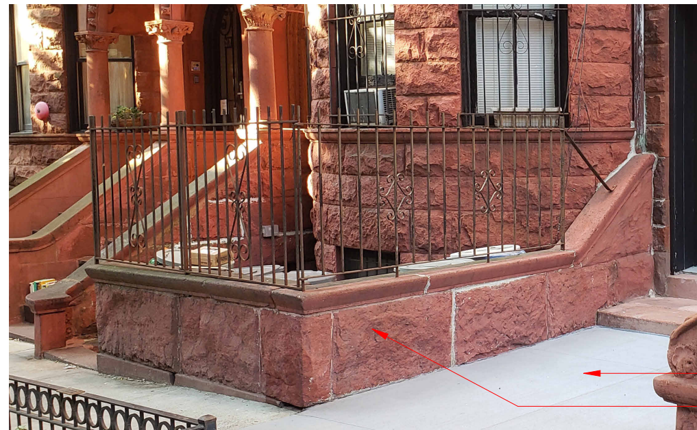
315 W 77TH - SIDEWALK RAILING
