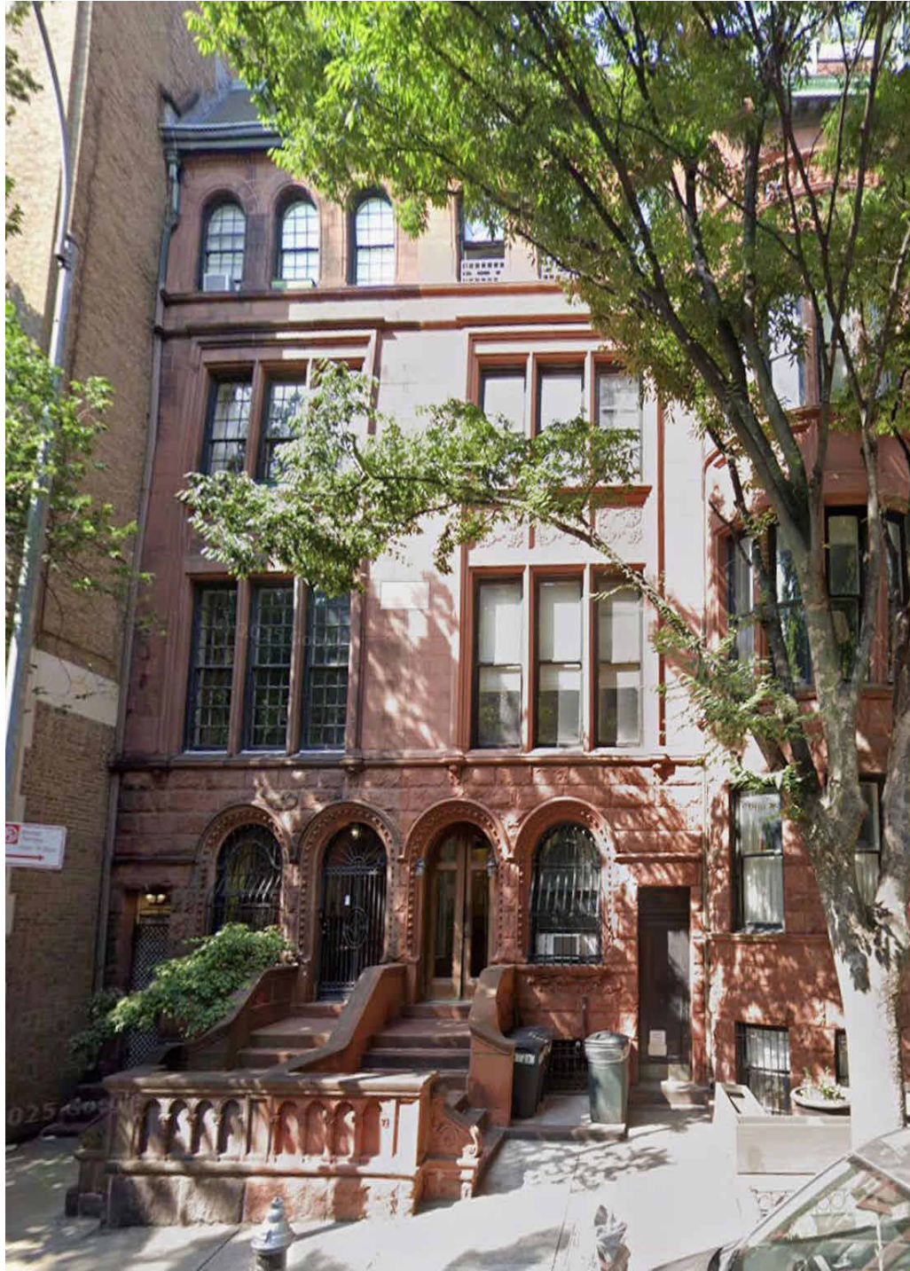
1. ROWHOUSE BLOCK NORTH VIEW -321 & 319
