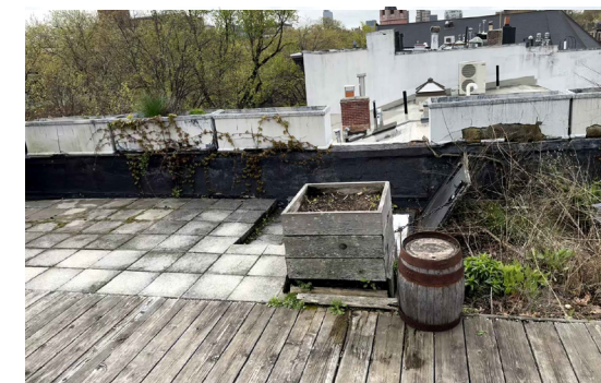
04 EXISTING ROOF HATCH
