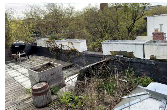
05 EXISTING ROOF HATCH
