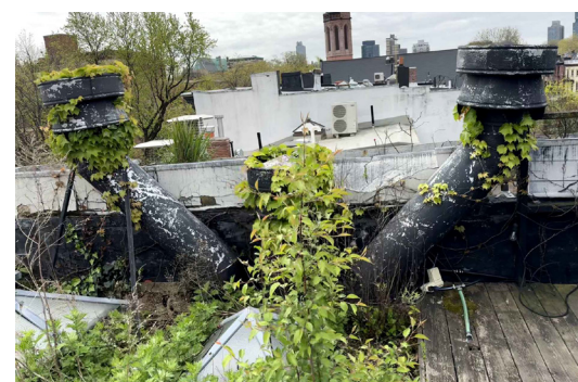
03 EXISTING VENTILATION DUCTS
