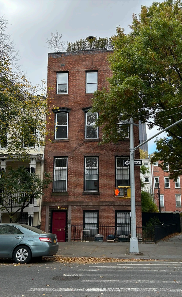
Existing Condition: Adelphi St. Facade
