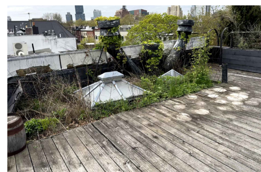
02 EXISTING SKYLIGHTS AND PLANTED AREA
