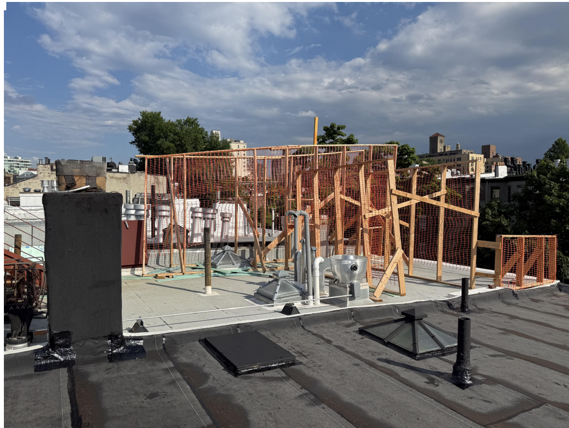
STAGED STRUCTURE MOCK UP
