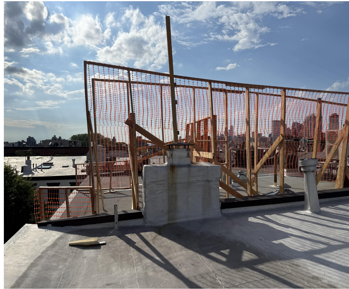
STAGED FLUE MOCK UP
