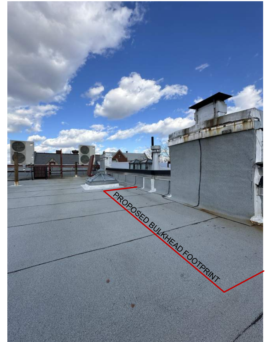
VIEW NORTH (TOWARDS LINCOLN PLACE)
