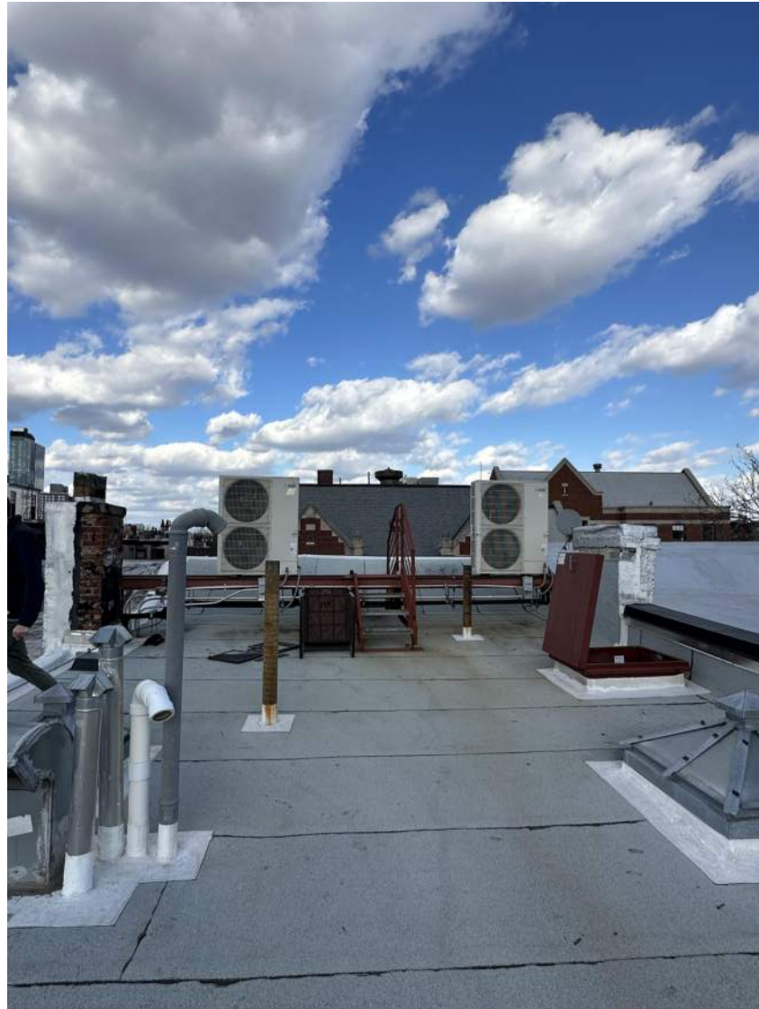
VIEW NORTH (TOWARDS LINCOLN PLACE)
