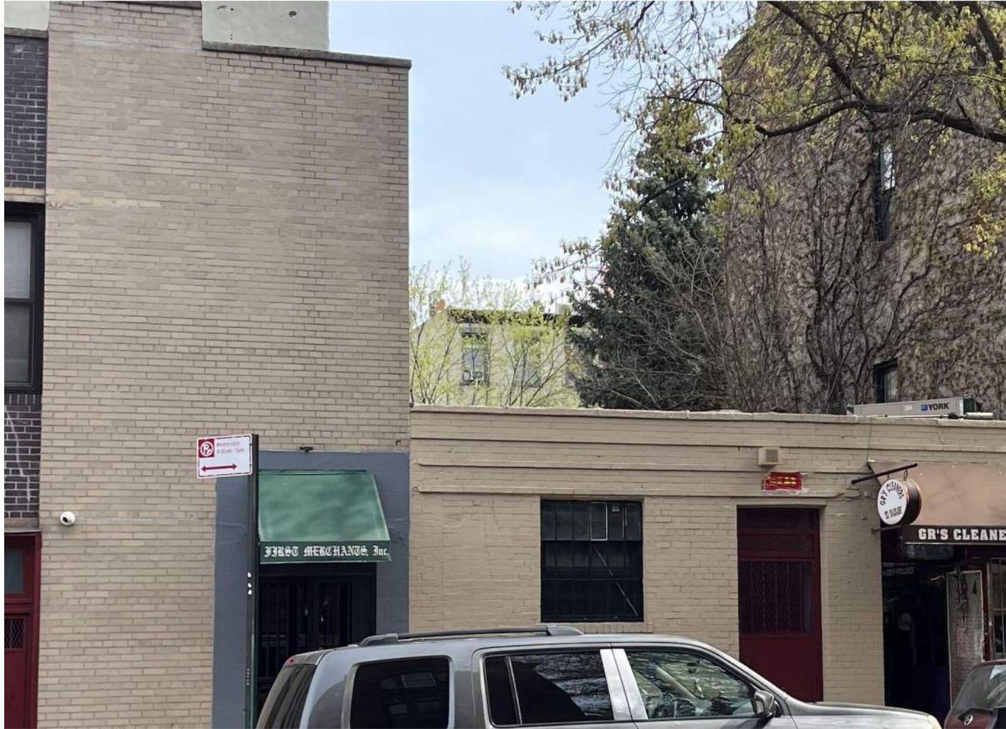
VIEW FROM THE CORNER OF 7TH AVE & BERKELEY PLACE PRIOR TO MOCK-UP
