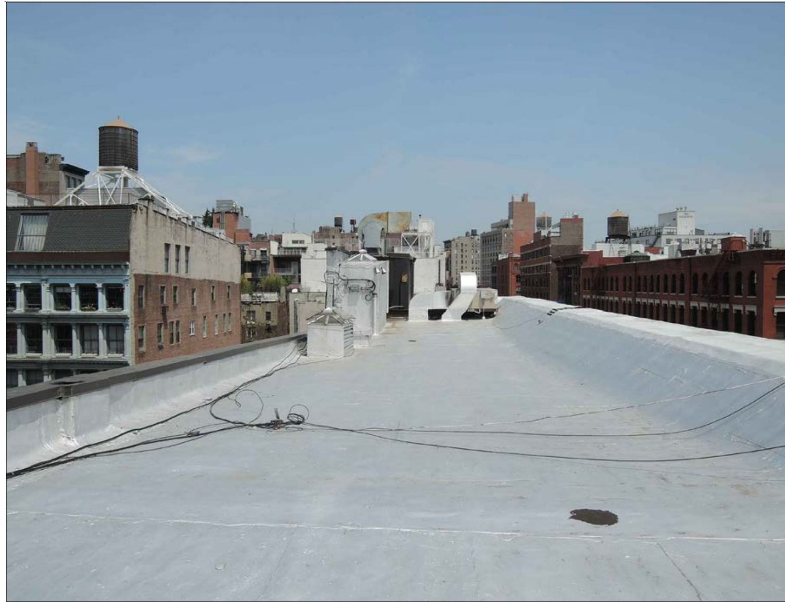
3 - ROOF-EXISTING CONDITIONS LOOKING NORTH
