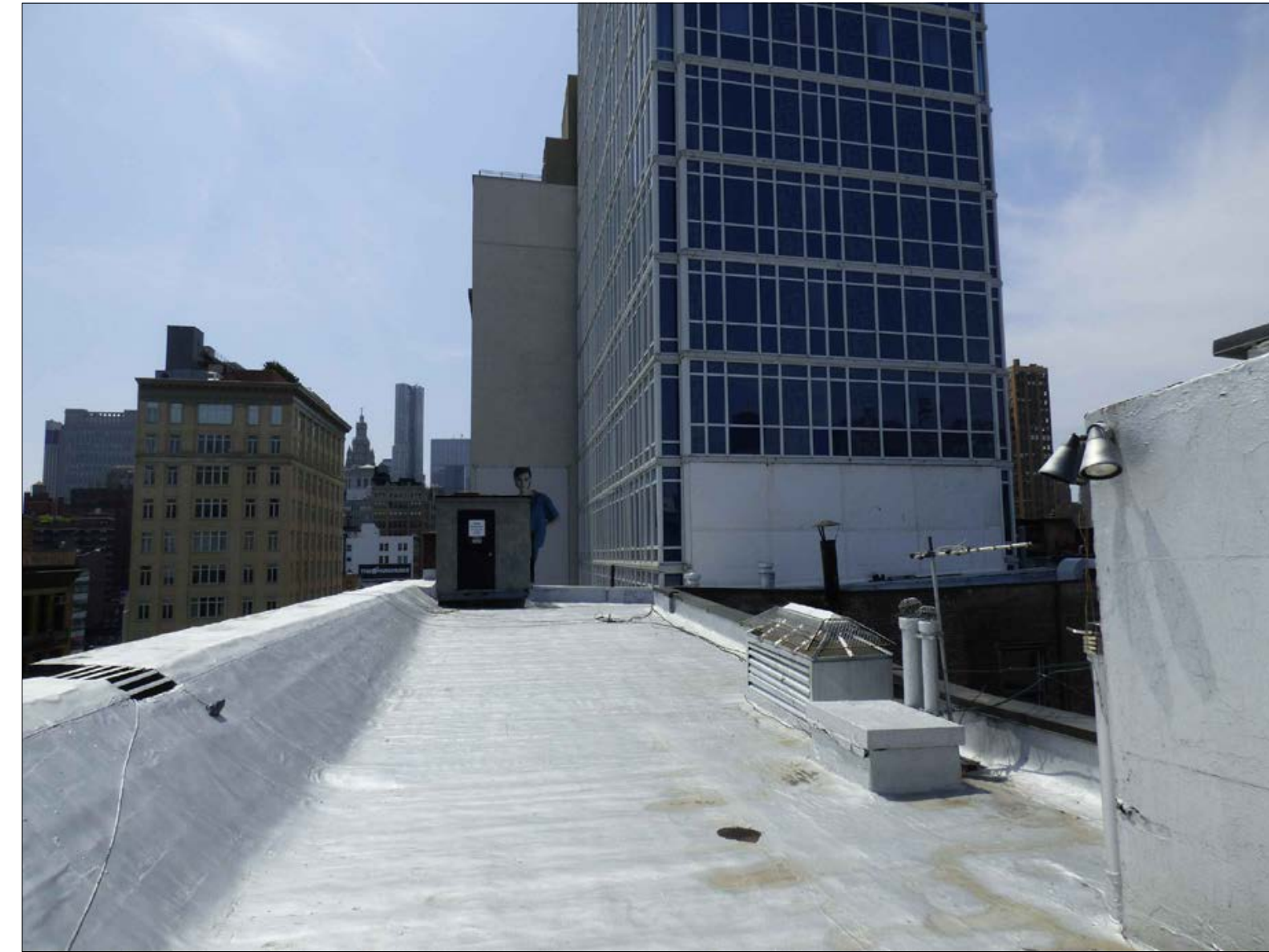
2 - ROOF-EXISTING CONDITIONS LOOKING SOUTH
