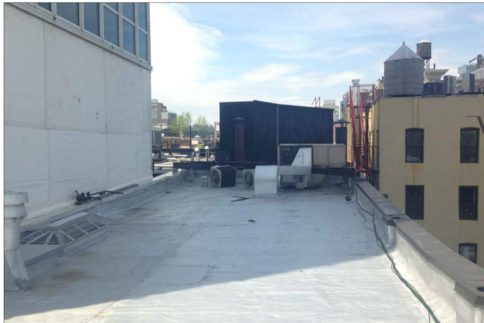
1 - ROOF - EXISTING CONDITIONS LOOKING WEST
