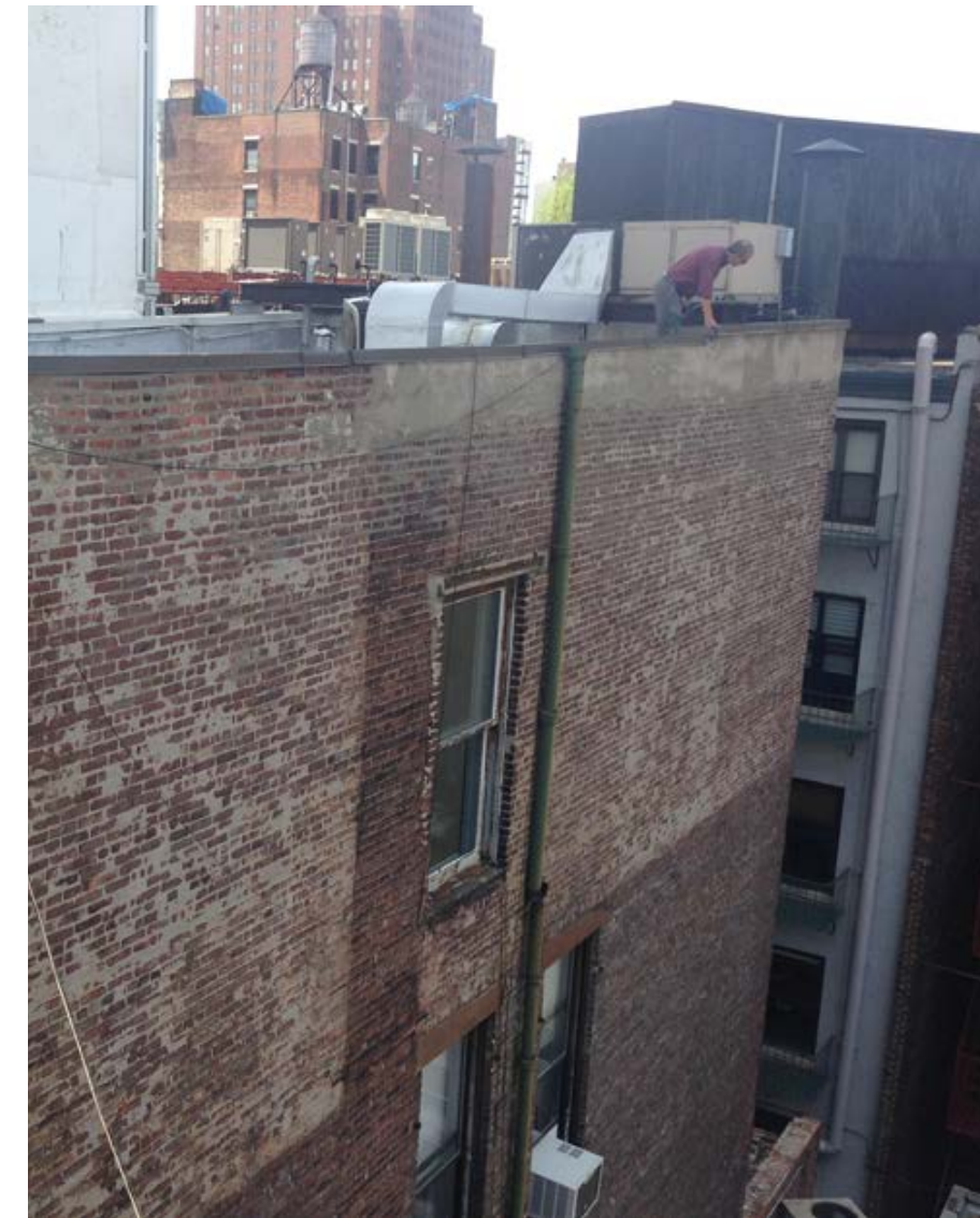
South inner wall
