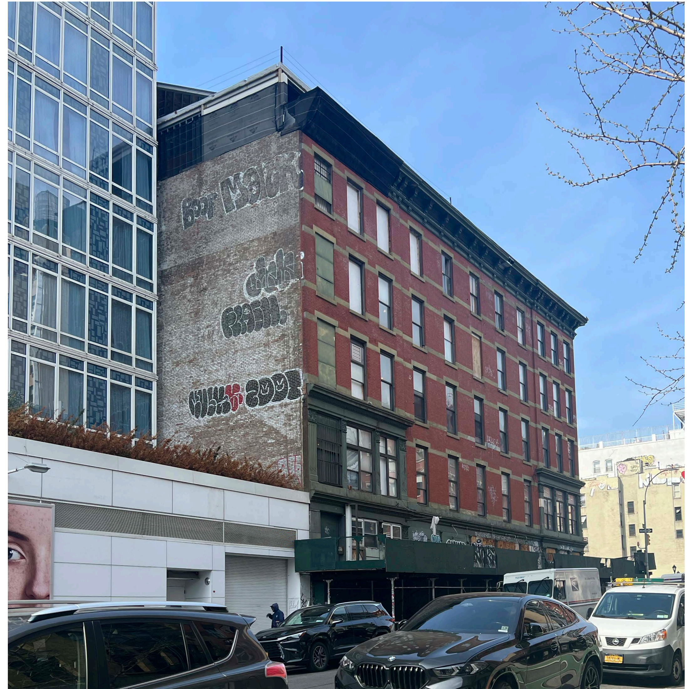
VIEW LOOKING NORTH ON LAFAYETTE STREET
