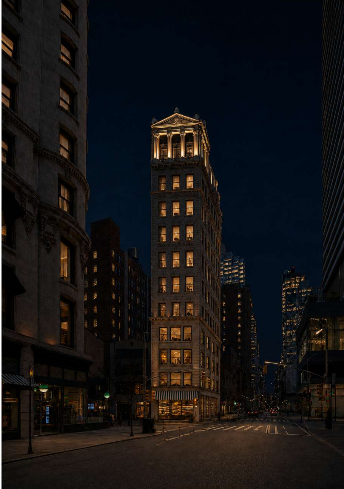
Nighttime View - From E 28 St Looking Towards Broadway
