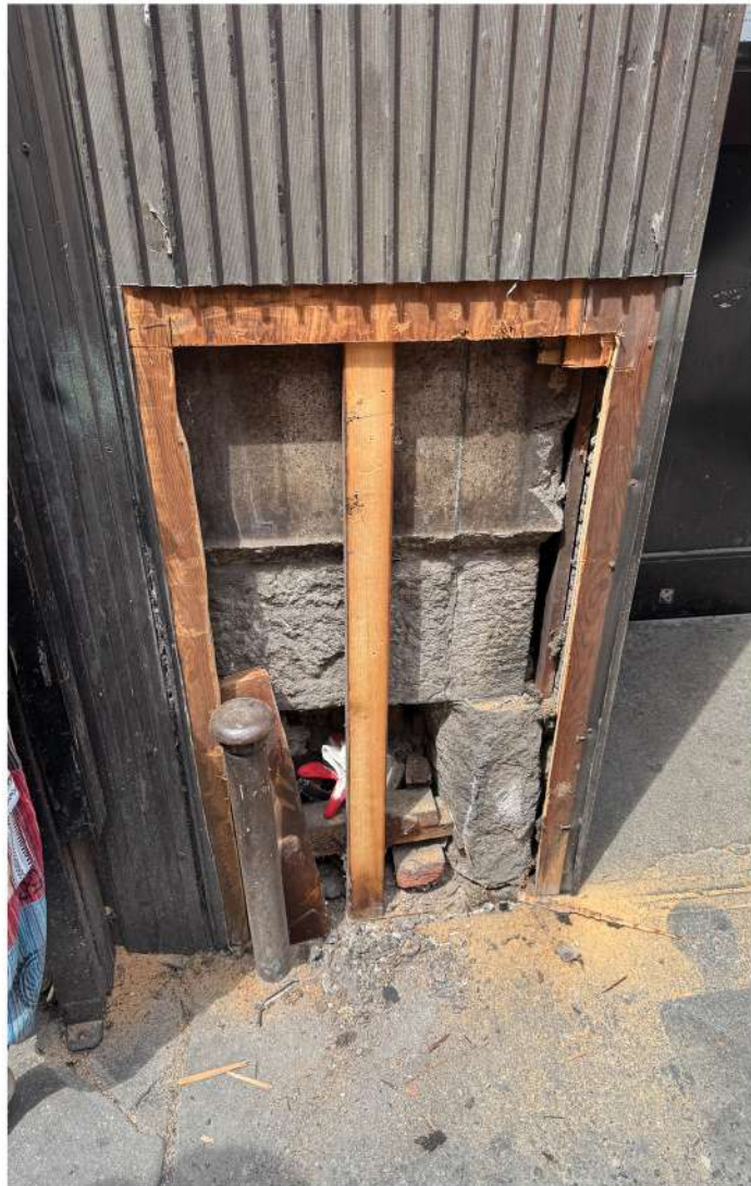
2026, Storefront - Base pier at Broadway
