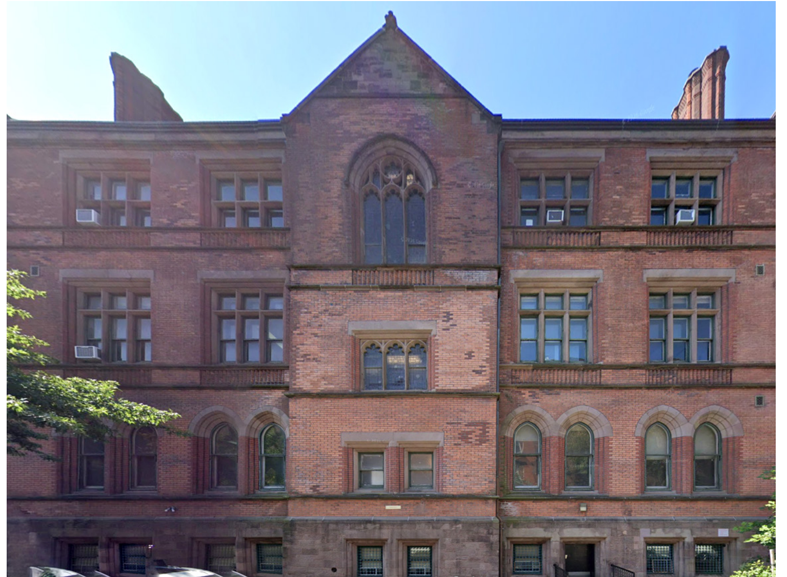
SHERRED NORTH FACADE FROM 21ST STREET
