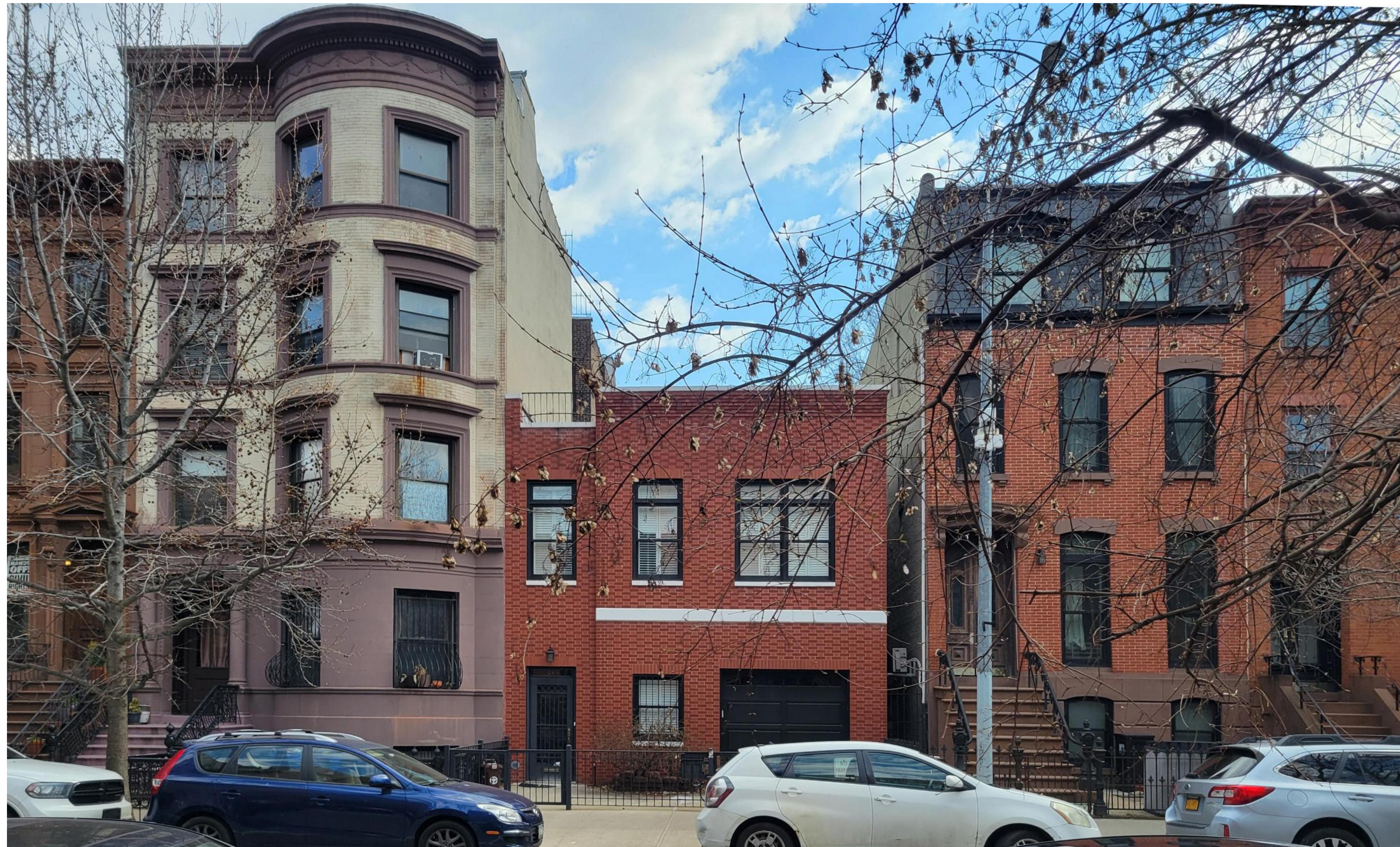
1 EXISTING view from across Cumberland St.
