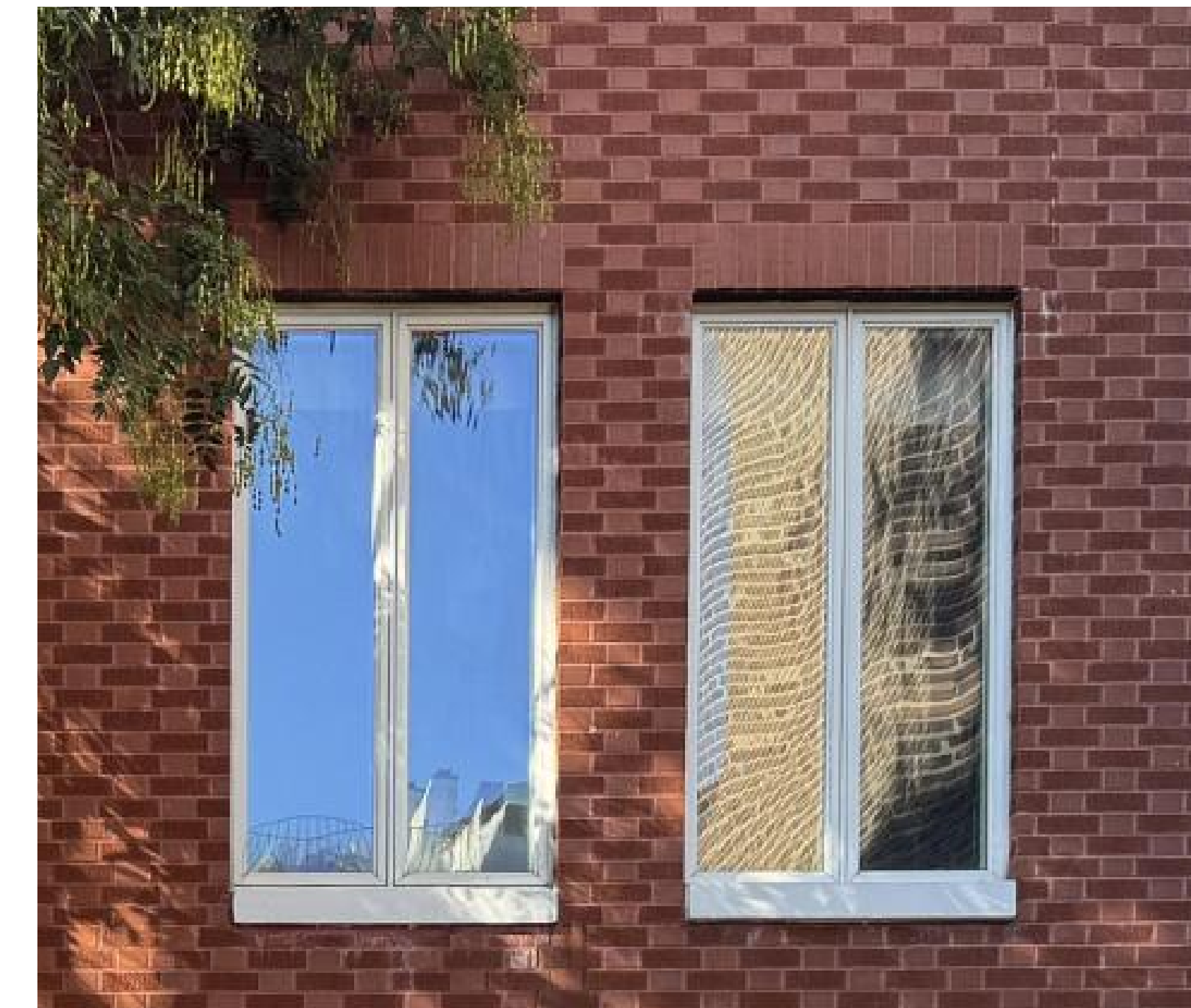
⑤ EXISTING Rear Casement Window
