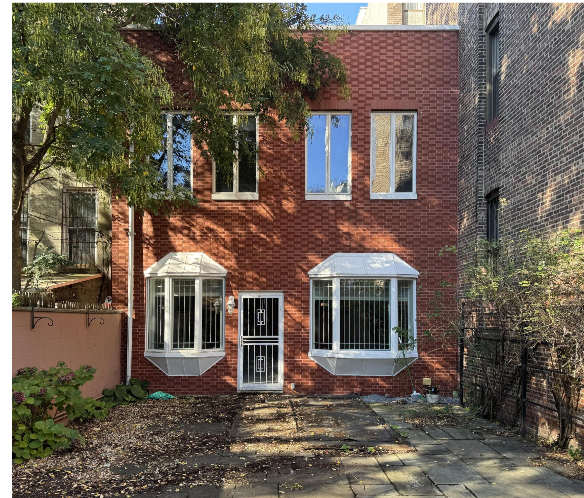
2 EXISTING Rear Facade (West)
