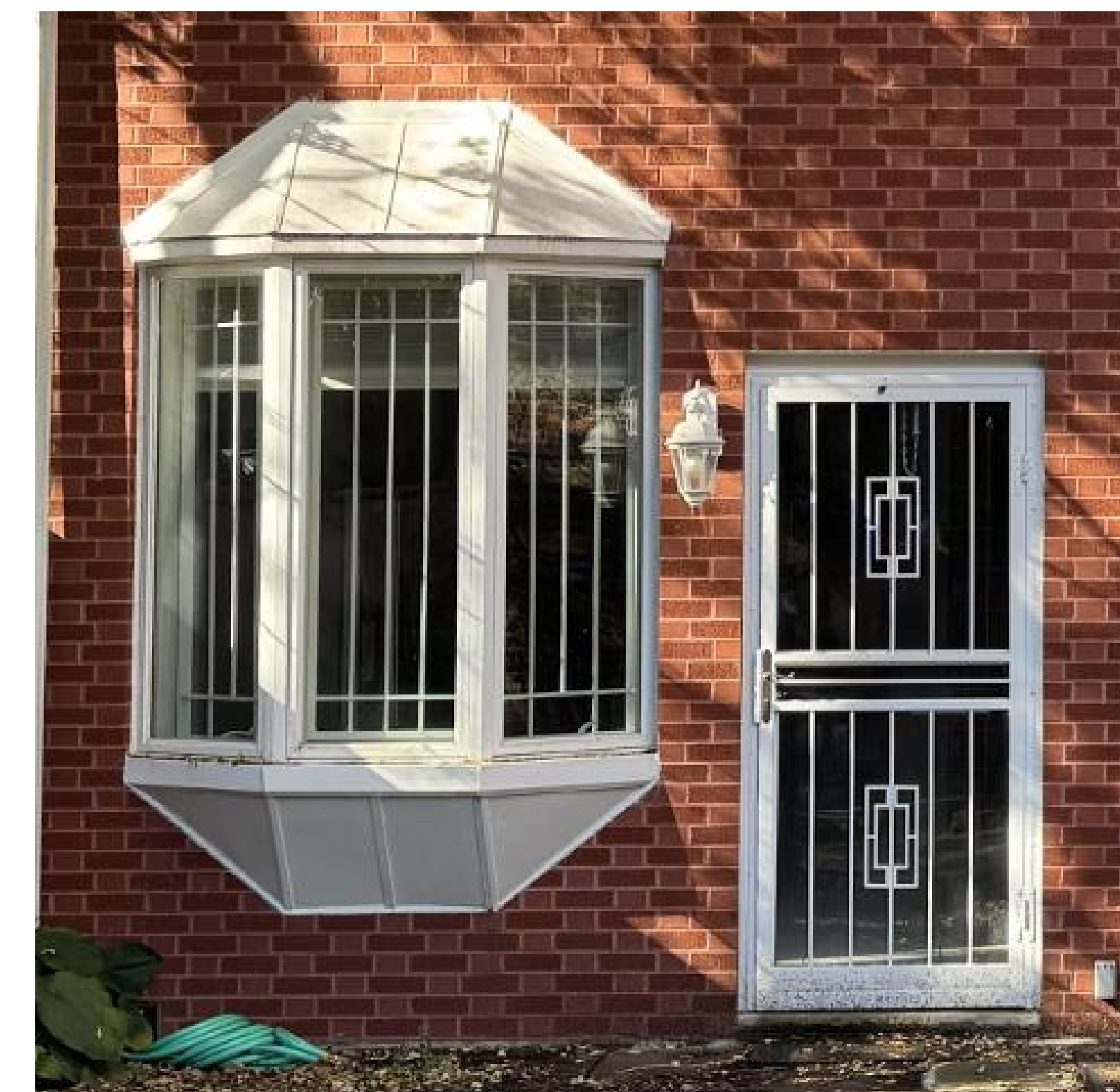
⑥ EXISTING Rear Bay Window and Door
