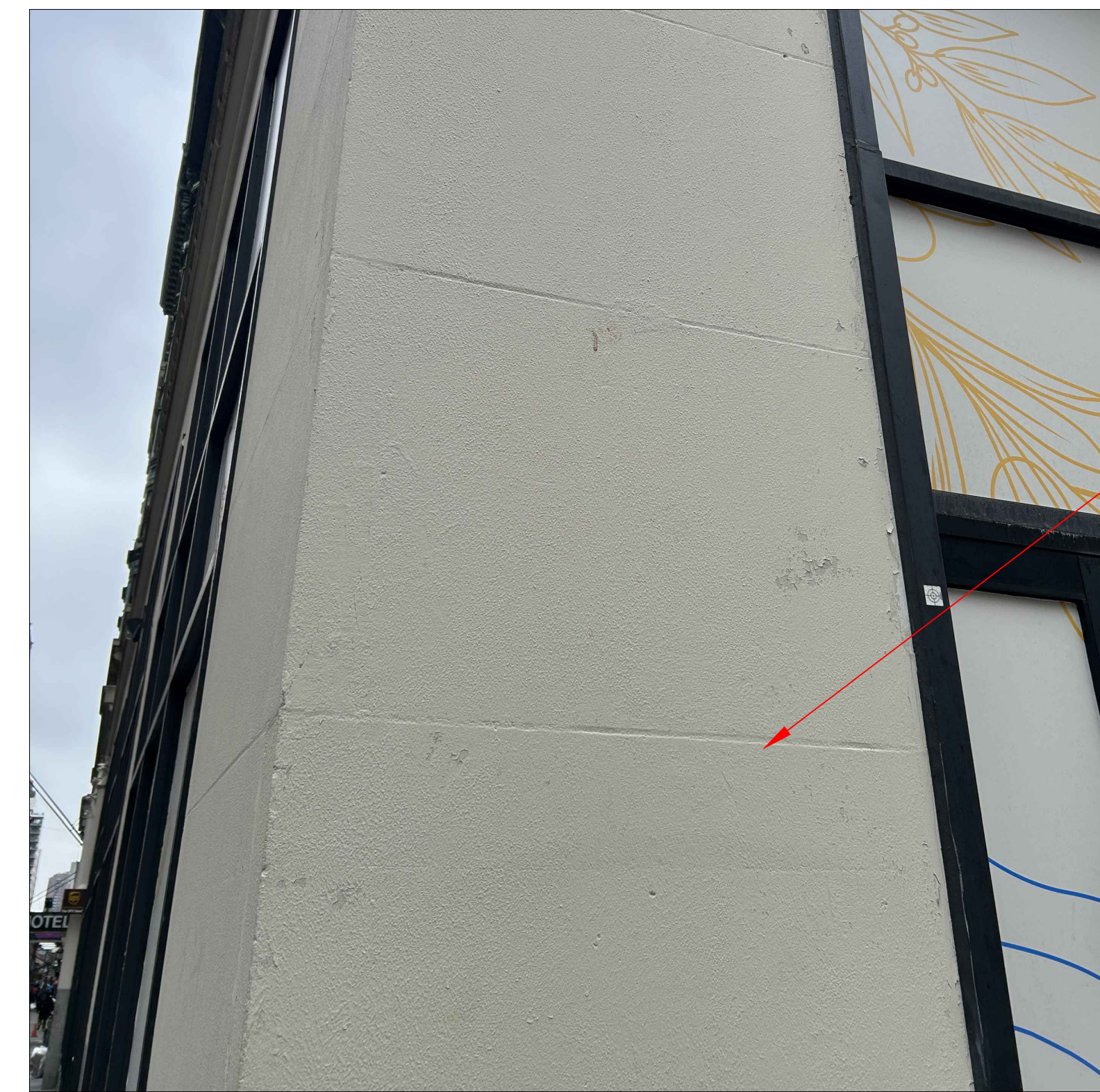
3 CLOSE-UP PHOTO OF BUILDING ELEVATION SCALE: NTS
