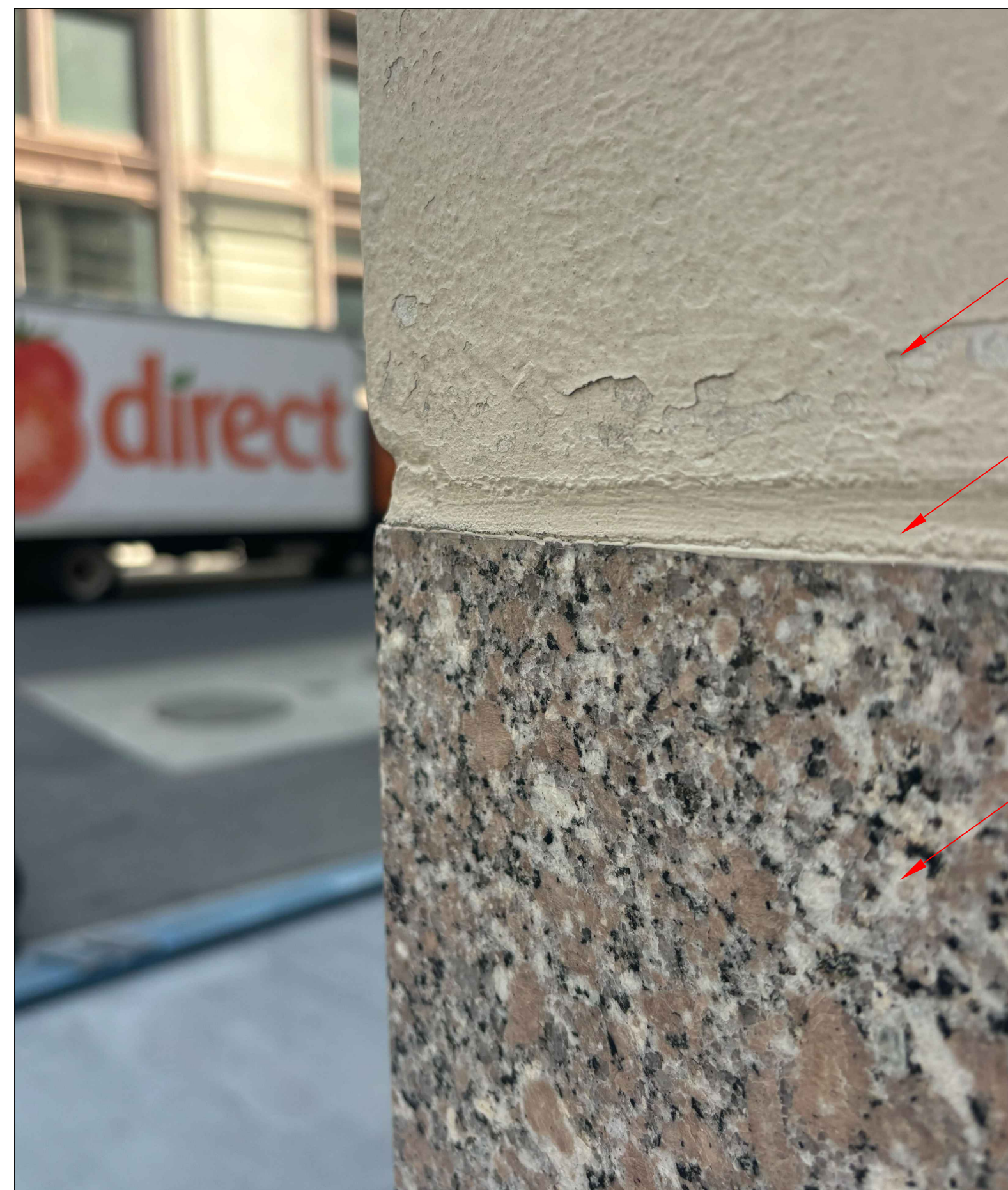
2 CLOSE-UP PHOTO OF MORTAR SCALE: NTS
