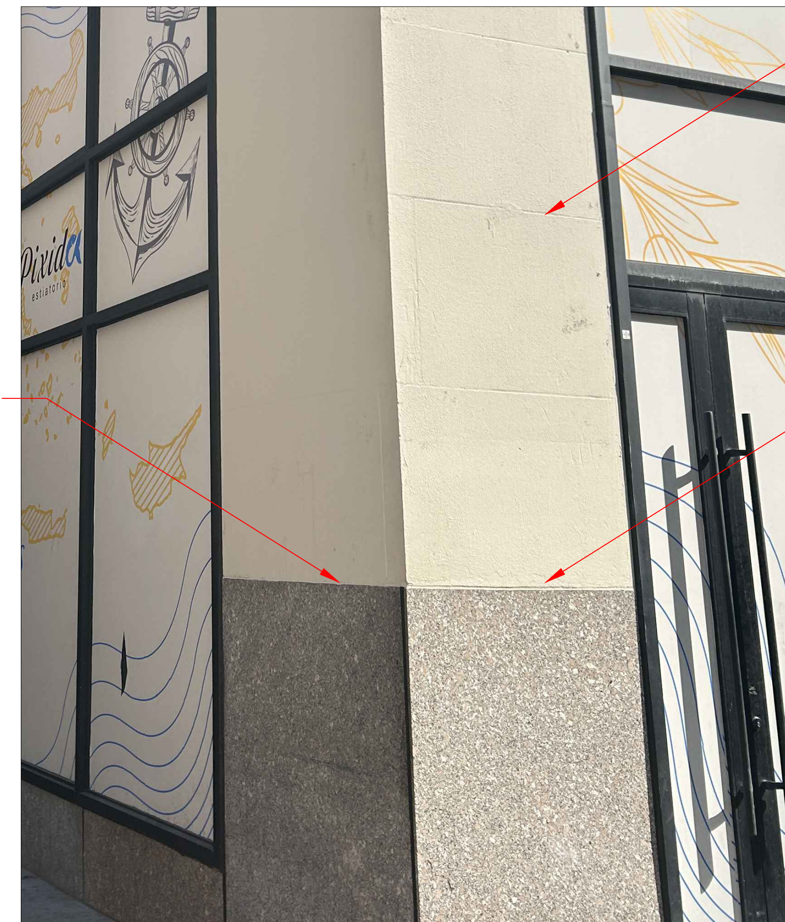
4 CLOSE-UP PHOTO OF BUILDING ELEVATION SCALE: NTS
