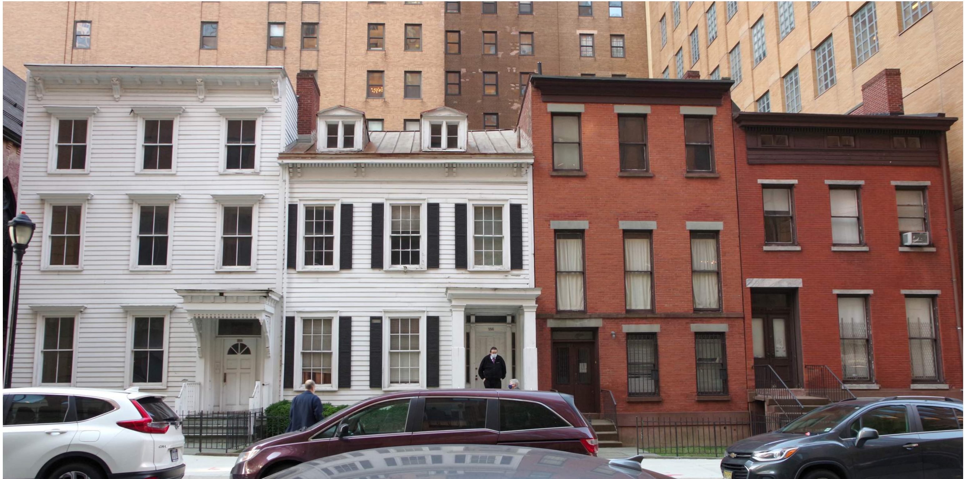
188 Duffield St. Built c. 1835-38 Remodeled in 1880s Queen Anne Second Empire details
