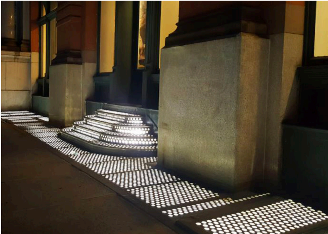
Restored cast iron vault lights at 295 Lafayette Street
