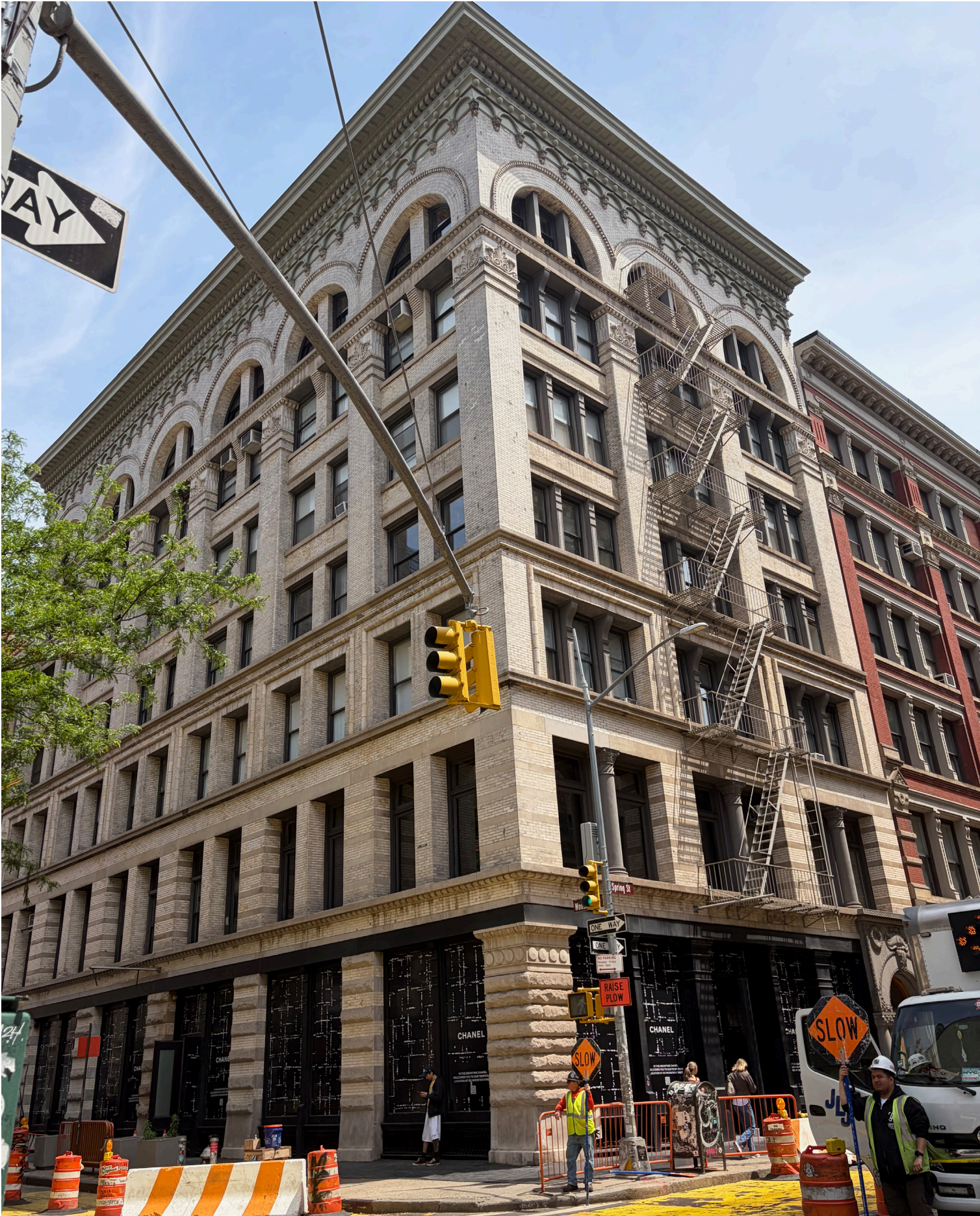
Northeast corner of Spring Street and Wooster
