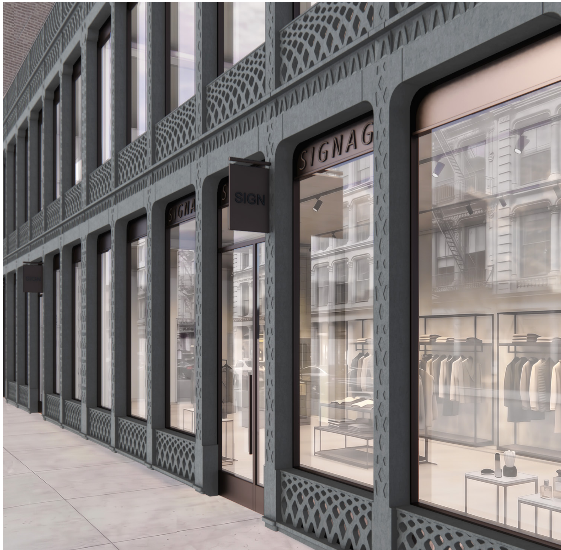
Wooster Street facade
