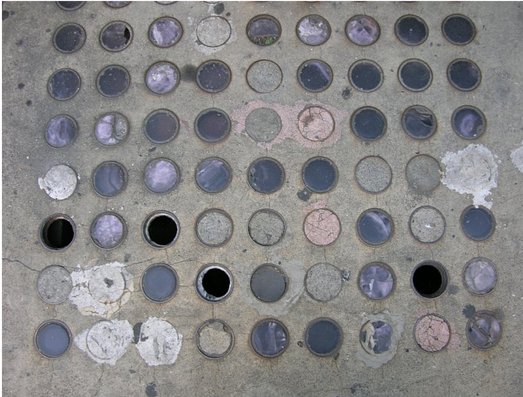
Typical concrete vault lights
