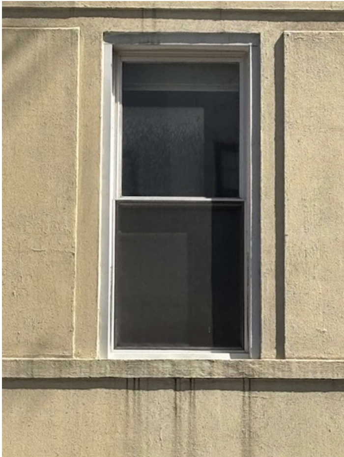
CLOSE UP OF UPPER WINDOWS, EXISTING
