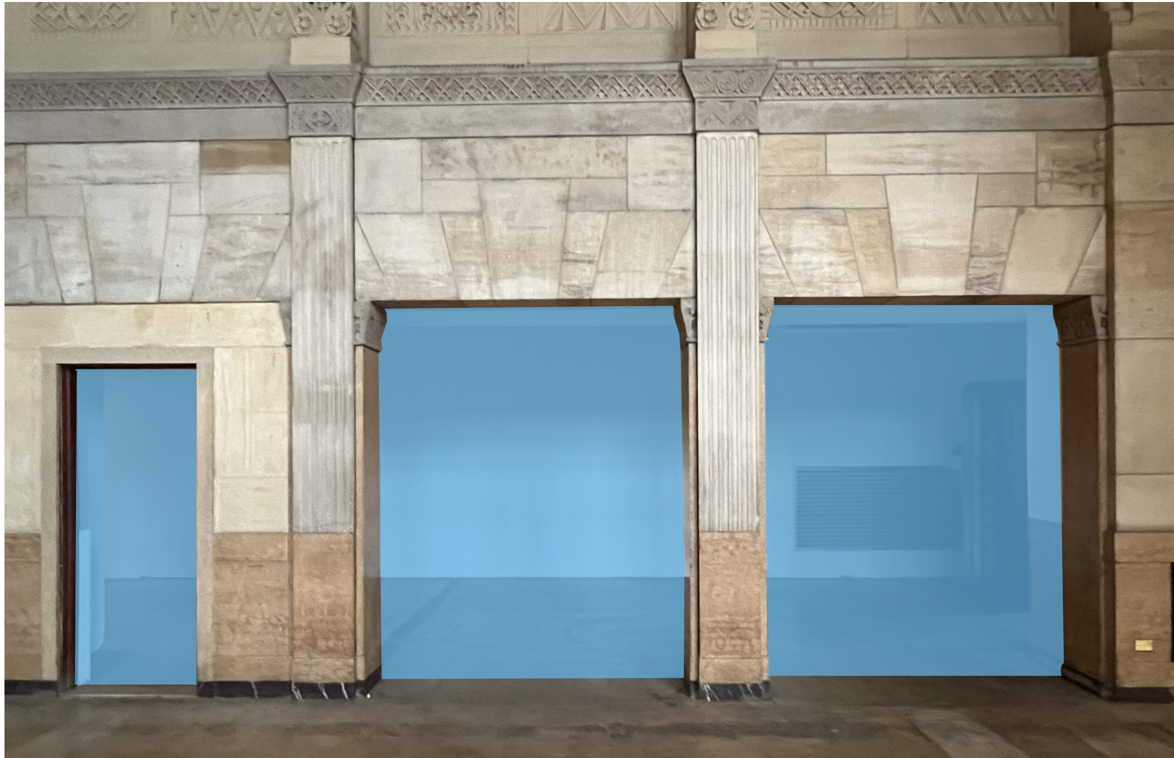
REMOVE DOOR, INFILL OPENING
