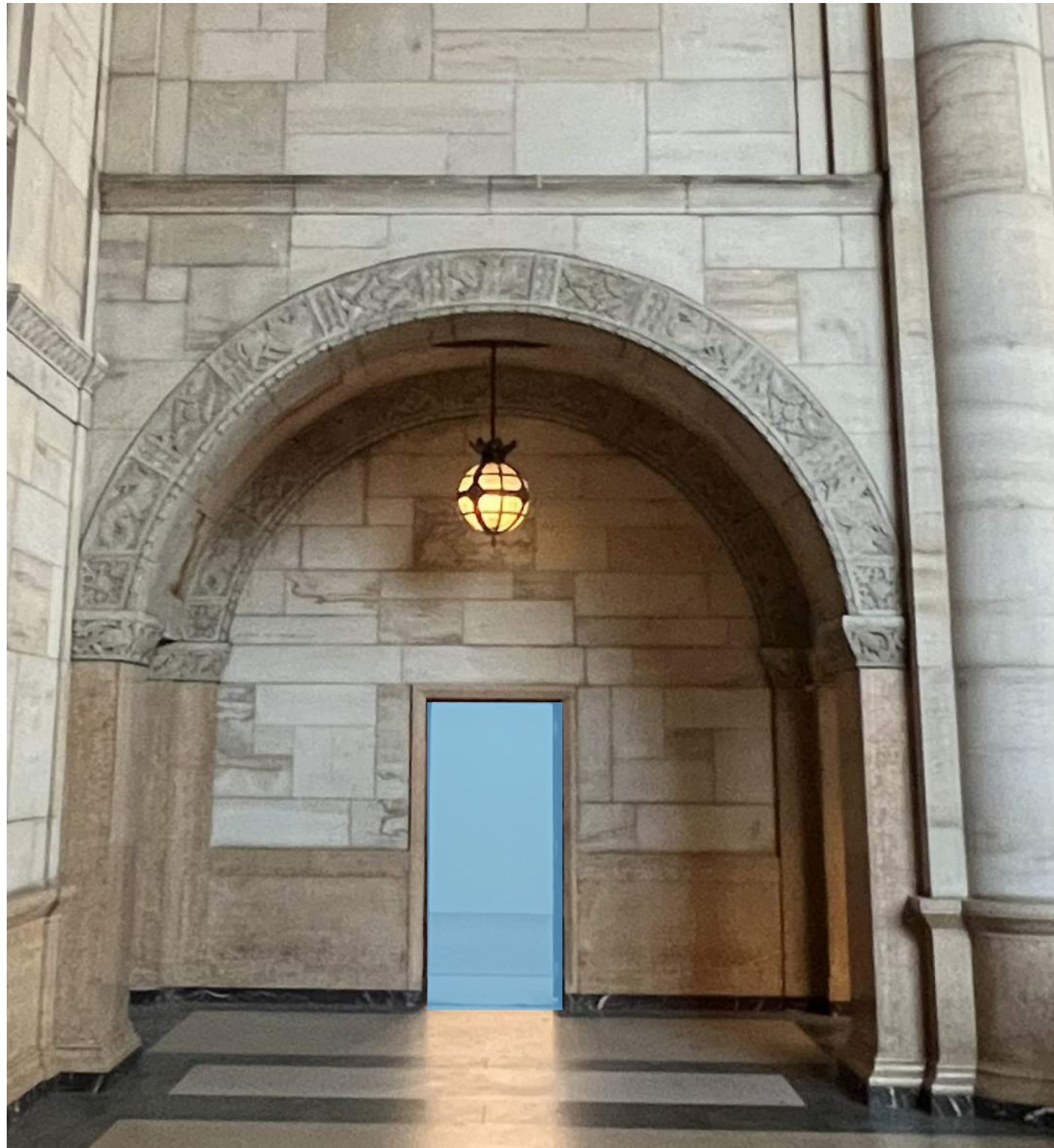
REMOVE DOOR, FRAME TO REMAIN
