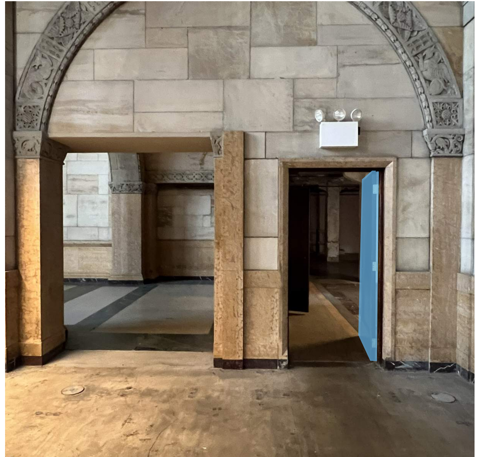
REMOVE DOOR, INFILL OPENING
