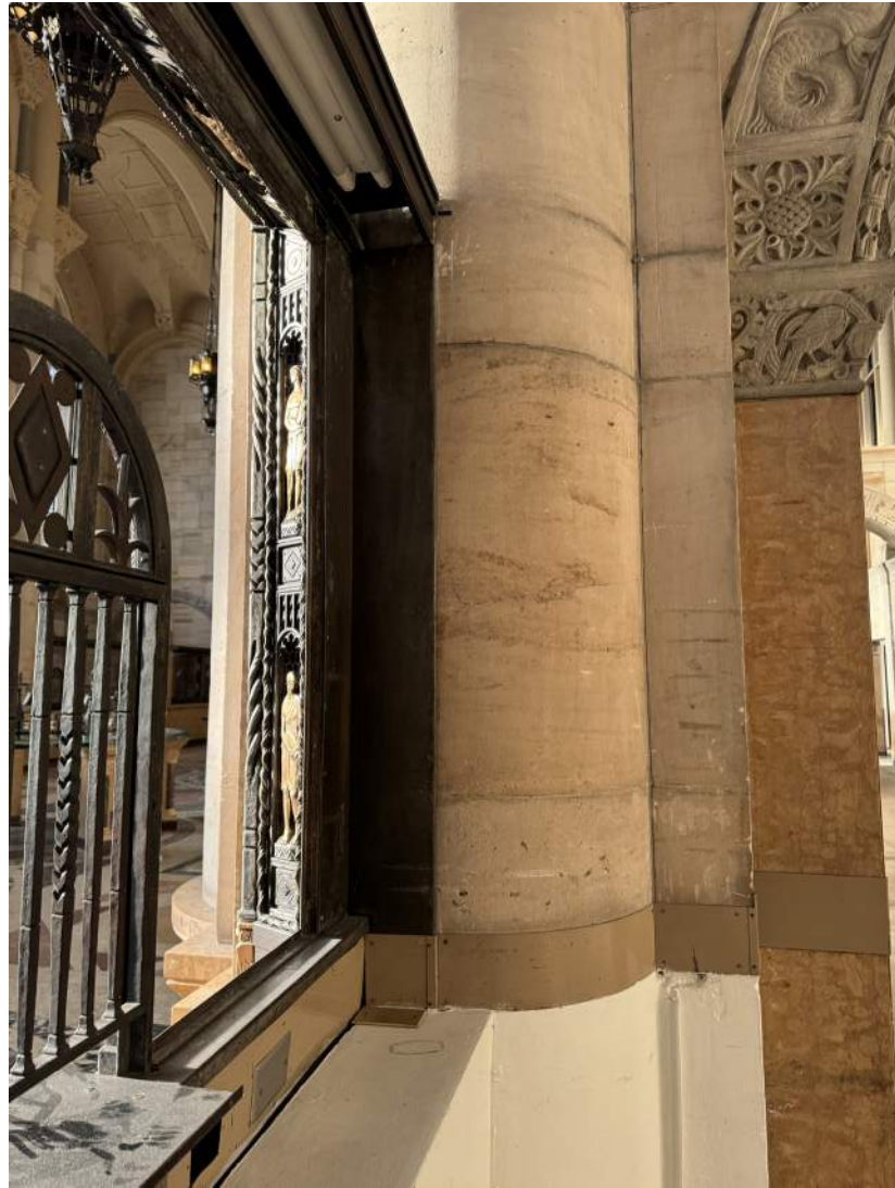
Teller Window Lighting
