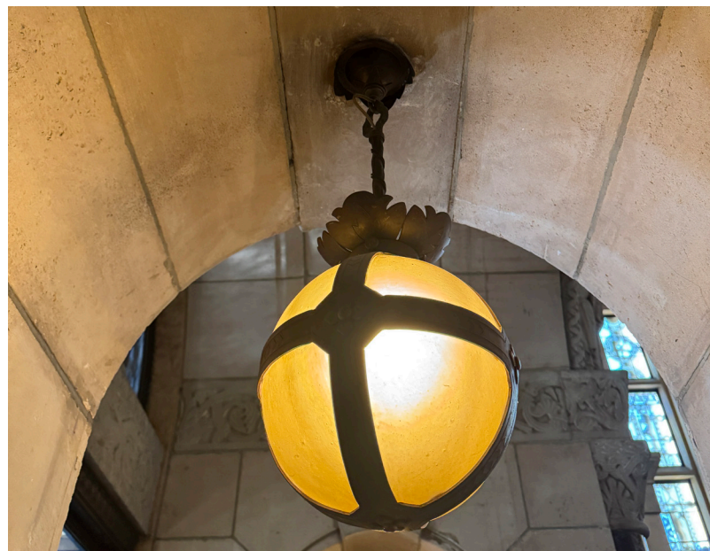
Existing lighting to be relamped with LEDs Hidden indirect lights to be added
