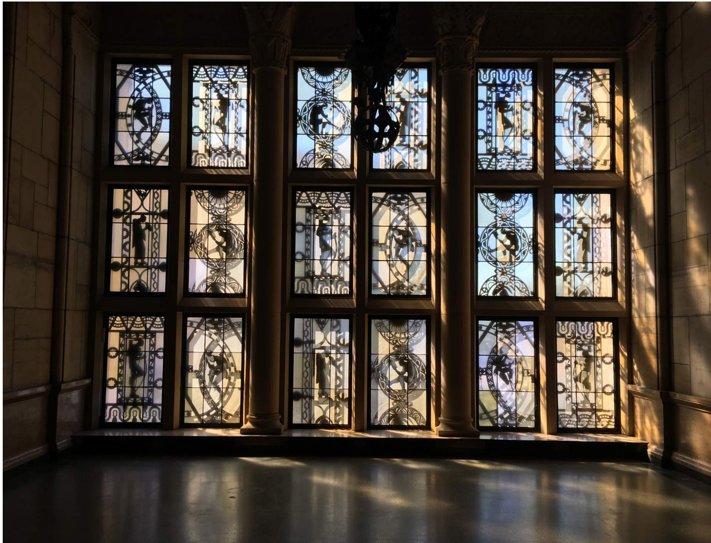
Mezzanine Windows Existing
