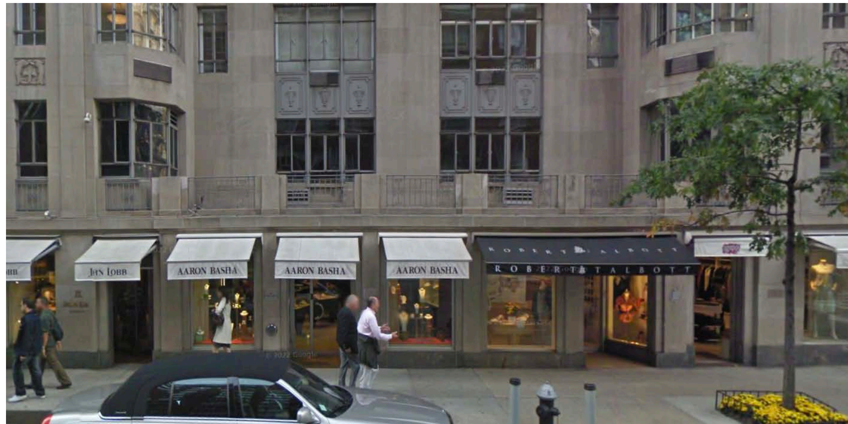
ORIGINAL BALUSTRADE AND RAILING IN 2009
