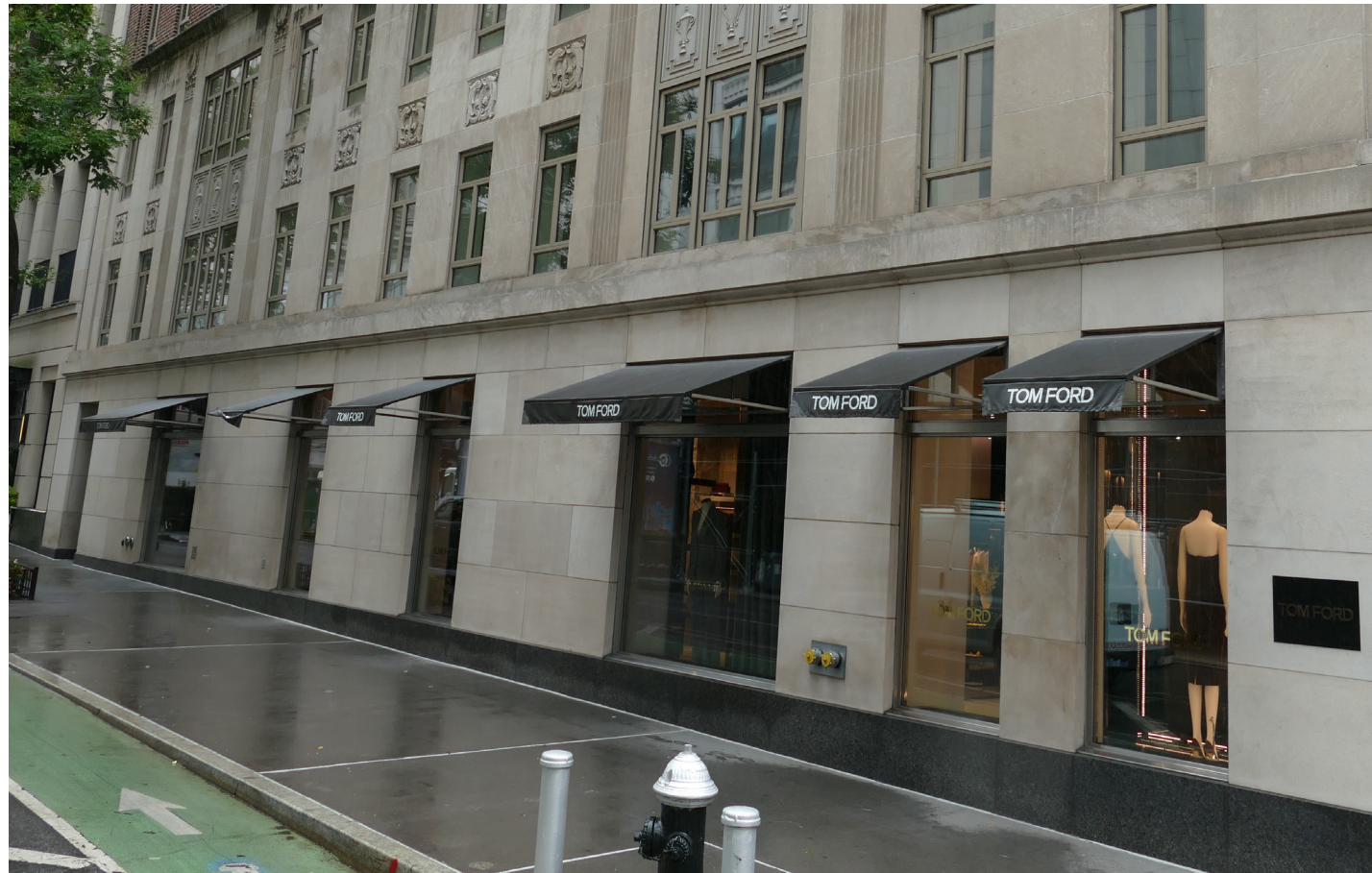
EXISTING STOREFRONT AT BUILDING BASE AT EAST 61ST STREET
