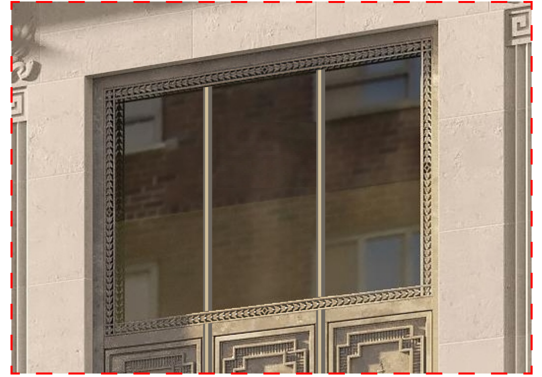
NEW DIVIDED WINDOW SYSTEM WITH REPLICATED DECORATIVE METAL FILIGREE BORDER (NICKEL FINISH)
