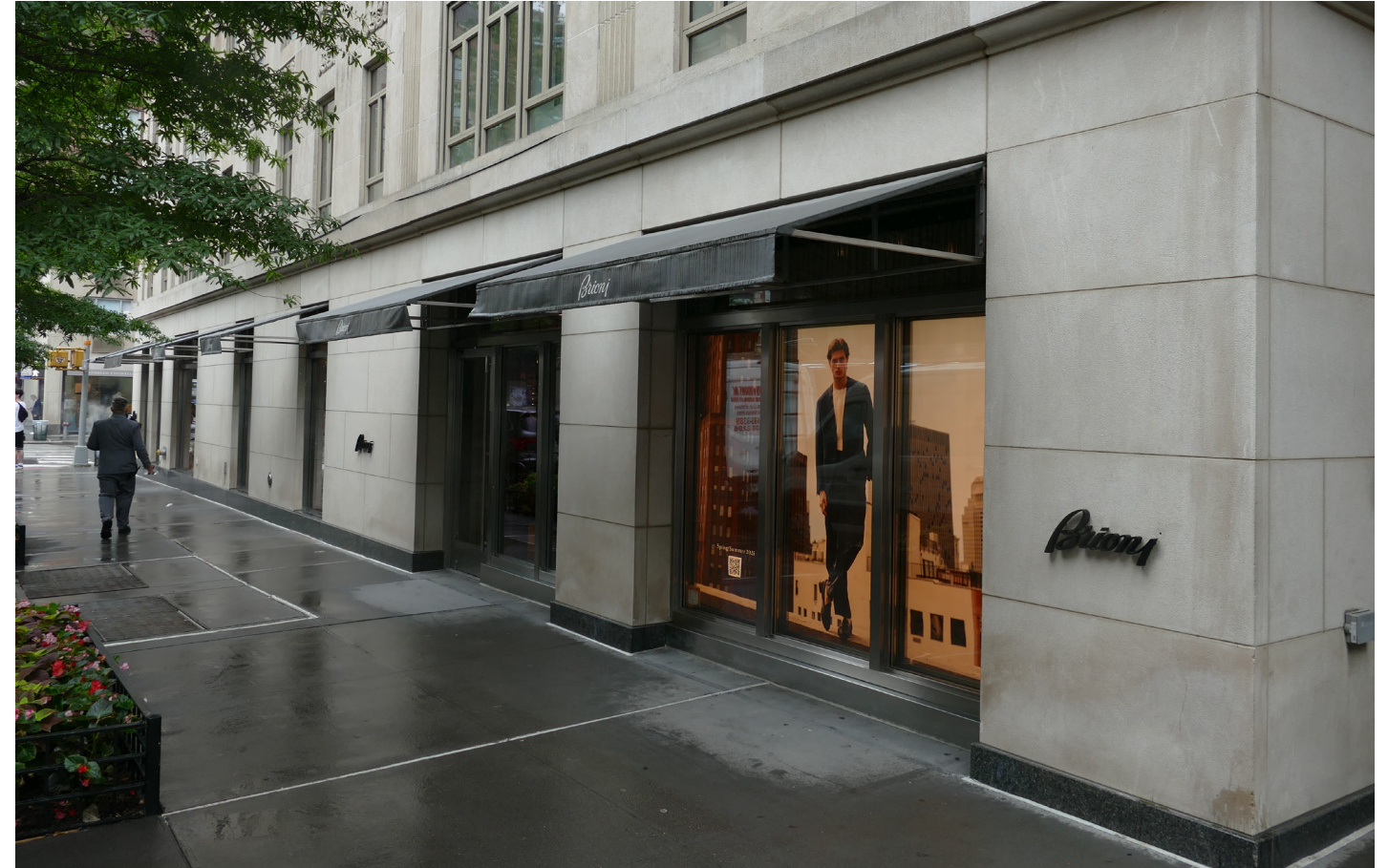
EXISTING STOREFRONT AT BUILDING BASE AT EAST 62ND STREET
