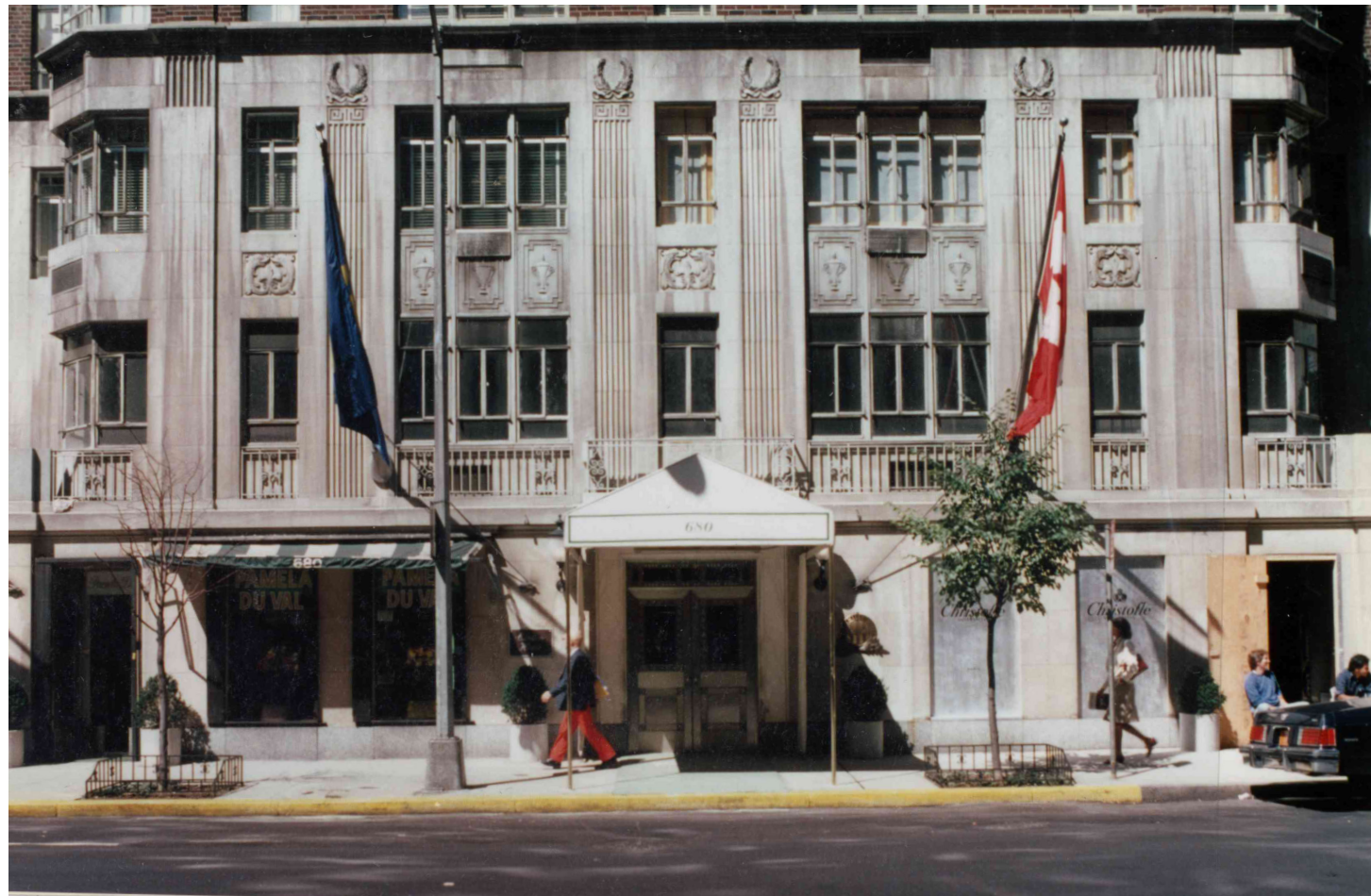
1981 (LPC DESIGNATION PHOTO)
