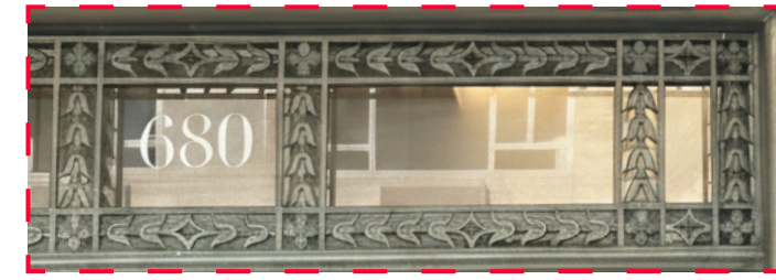
DETAIL OF EXISTING DECORATIVE METAL FILIGREE (NICKEL FINISH)
