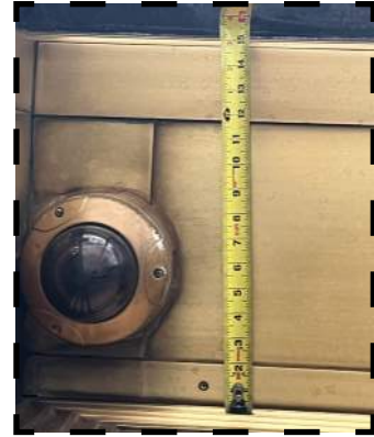
HEADER DEPTH & CAMERA LOCATION
