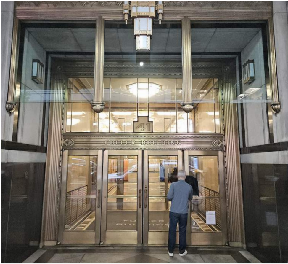
MAIN ENTRANCE EXTERIOR DOOR
