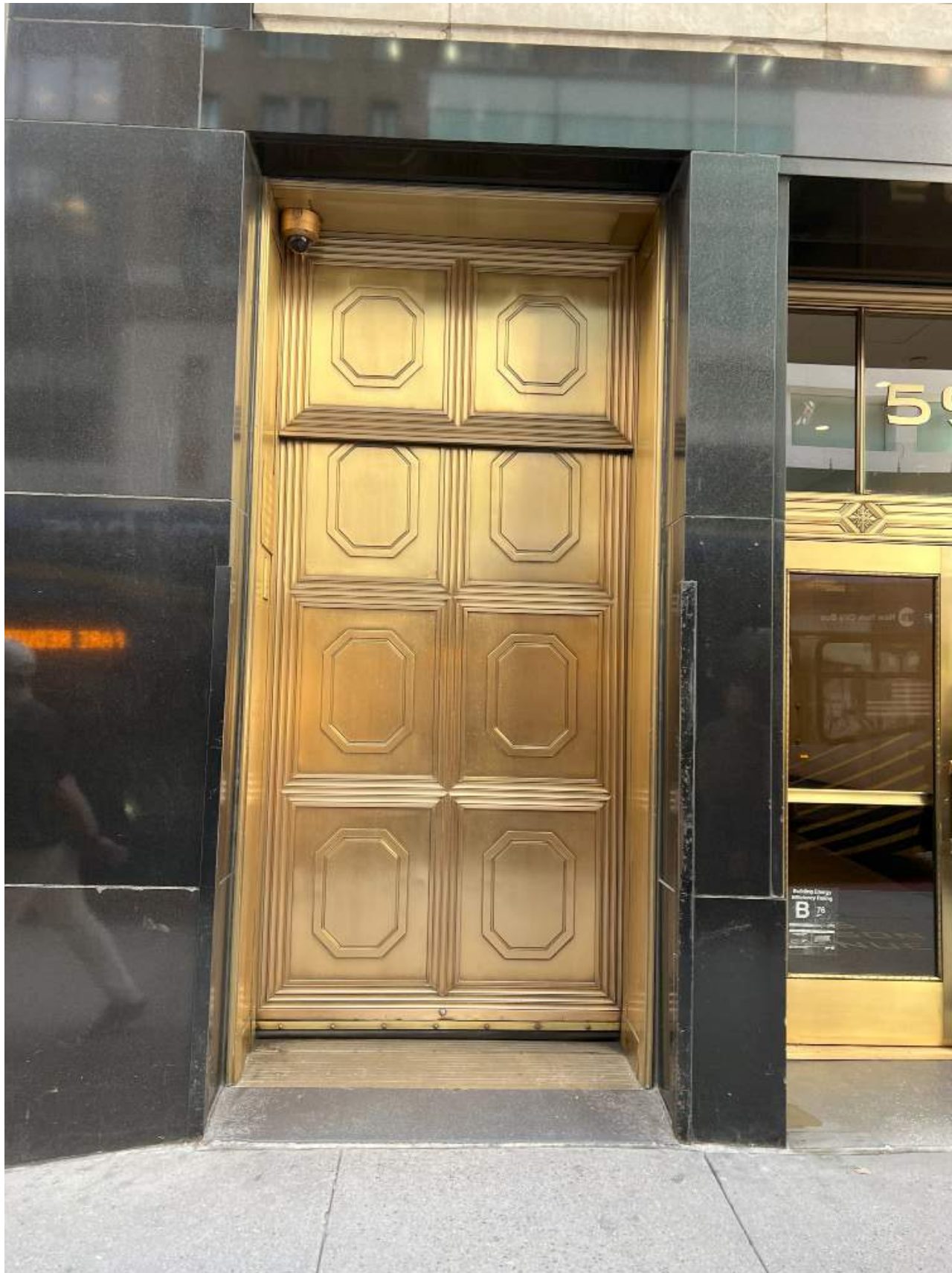
PH-1 EXISTING LOADING DOCK DOOR
