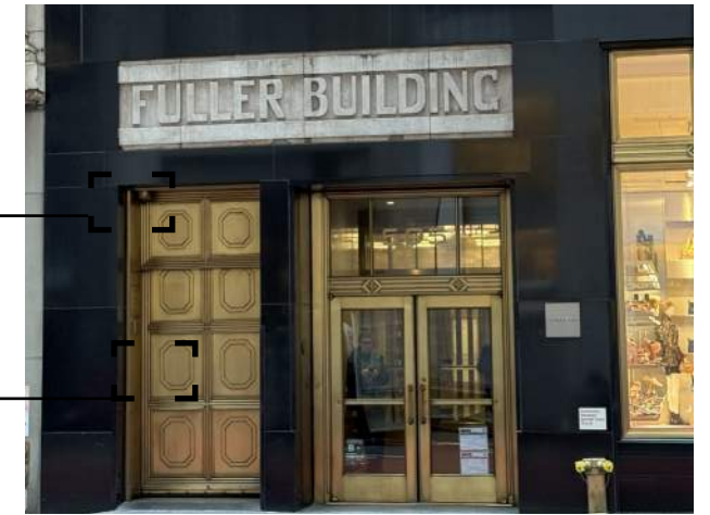
PHOTO @ MADISON AVENUE FREIGHT ELEVATOR DOOR
