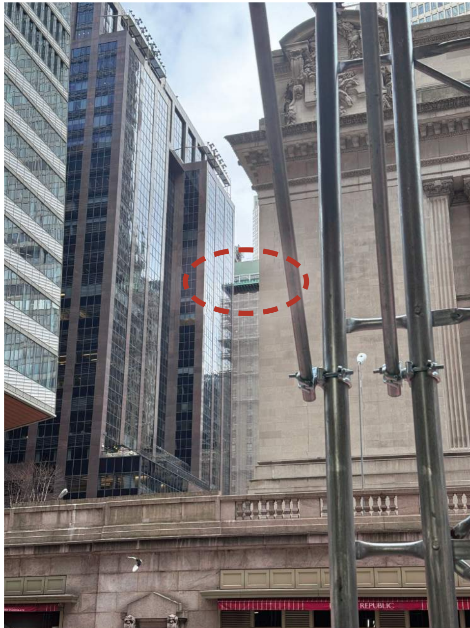
③ Existing Structure is Partially Visible
