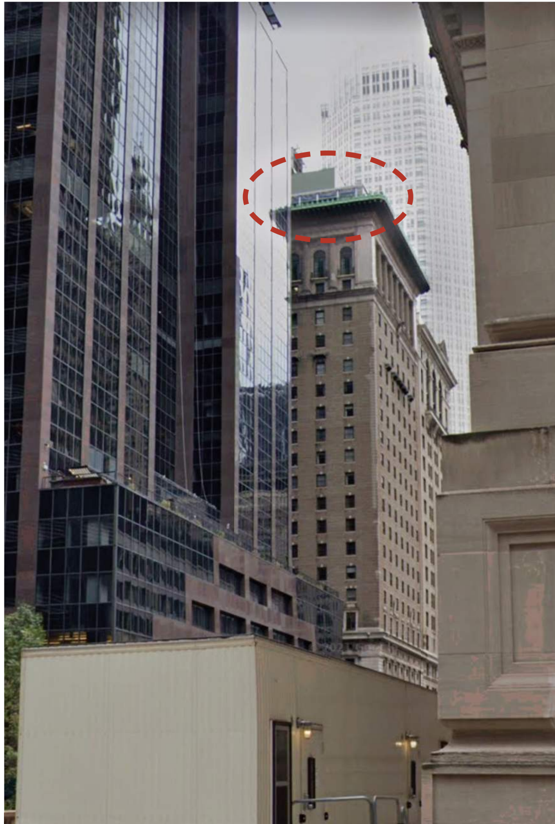
4 Existing Structure is Visible
