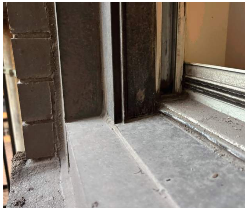
Typical Existing Type B1 Sill
