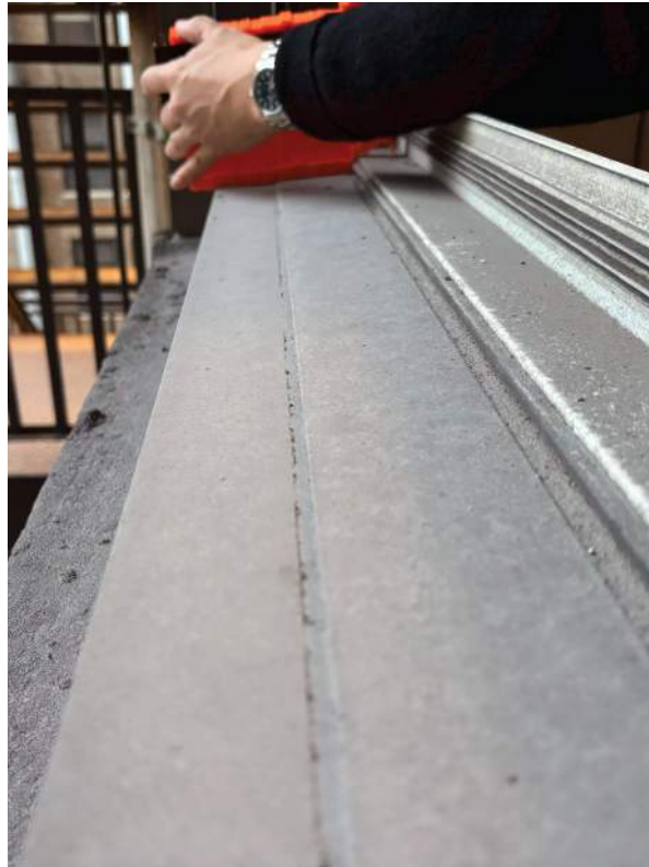
Typical Existing Type A Exterior Sill
