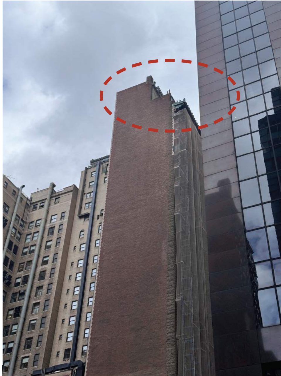
① Existing Structure is Not Visible
