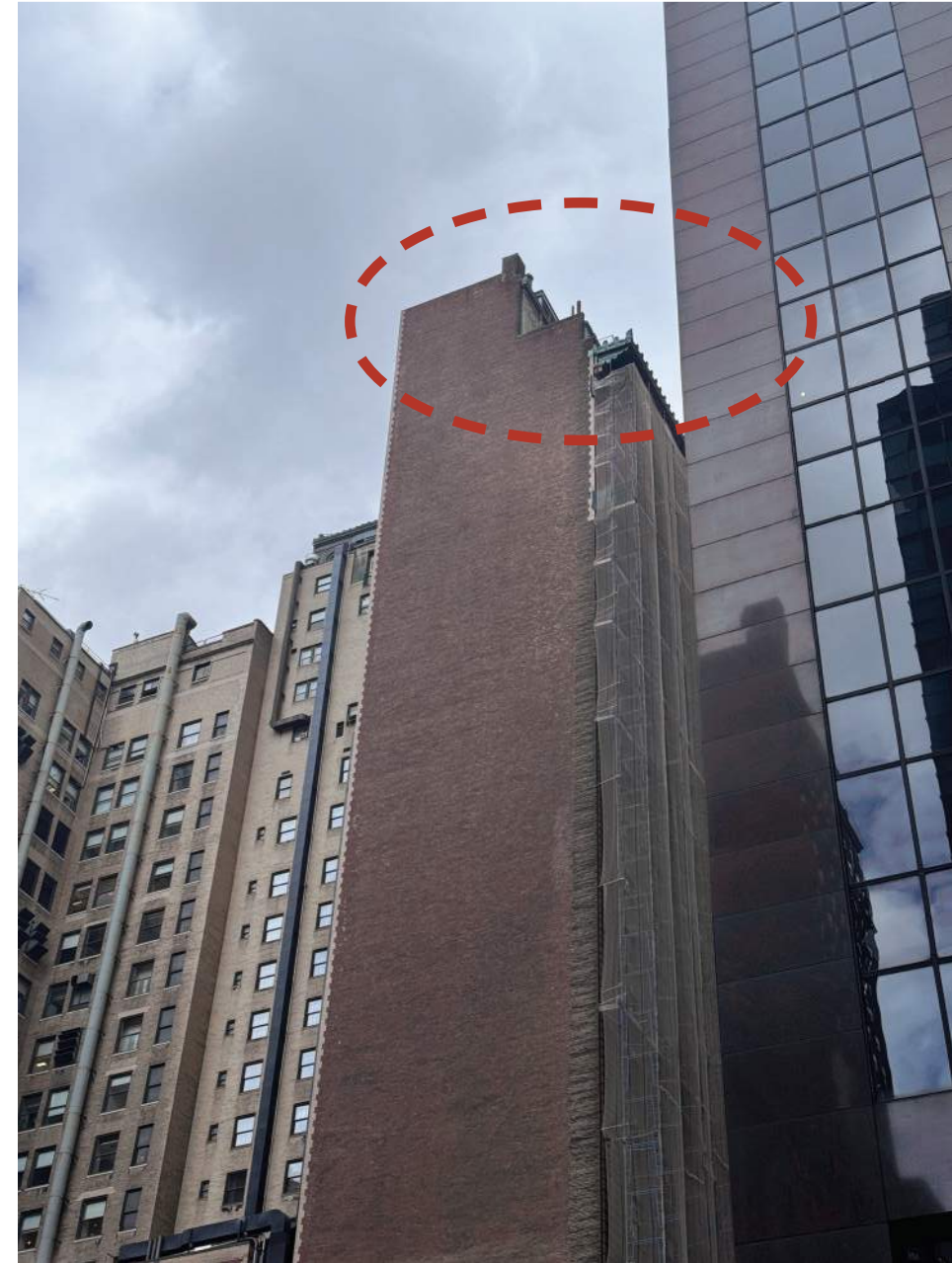
① Proposed Structure is Not Visible
