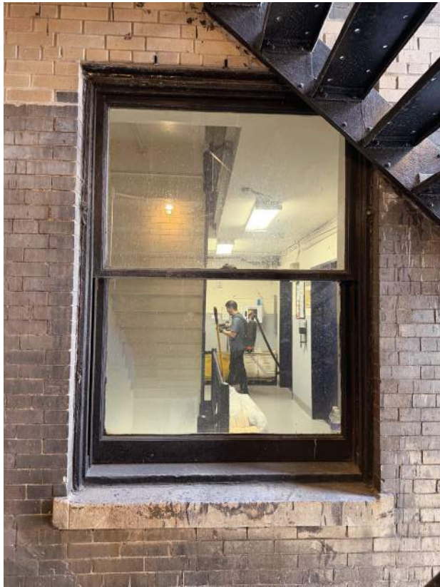
Typical Existing Type C2
