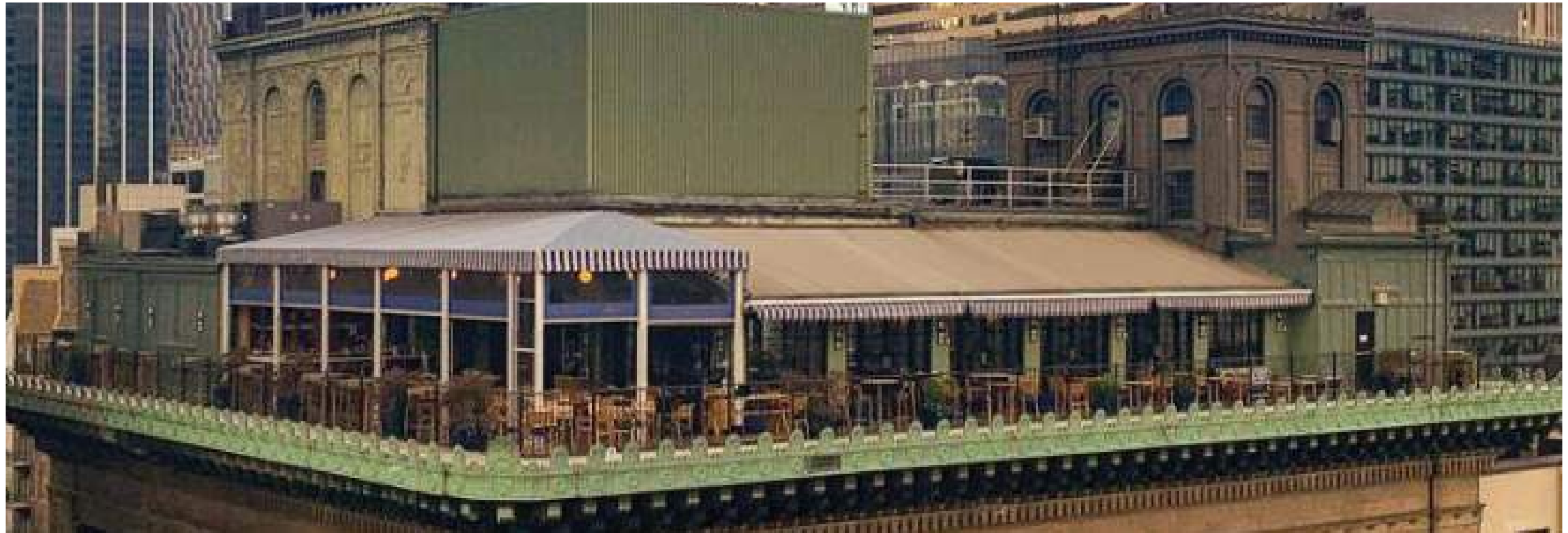
Existing Roof, Photo
