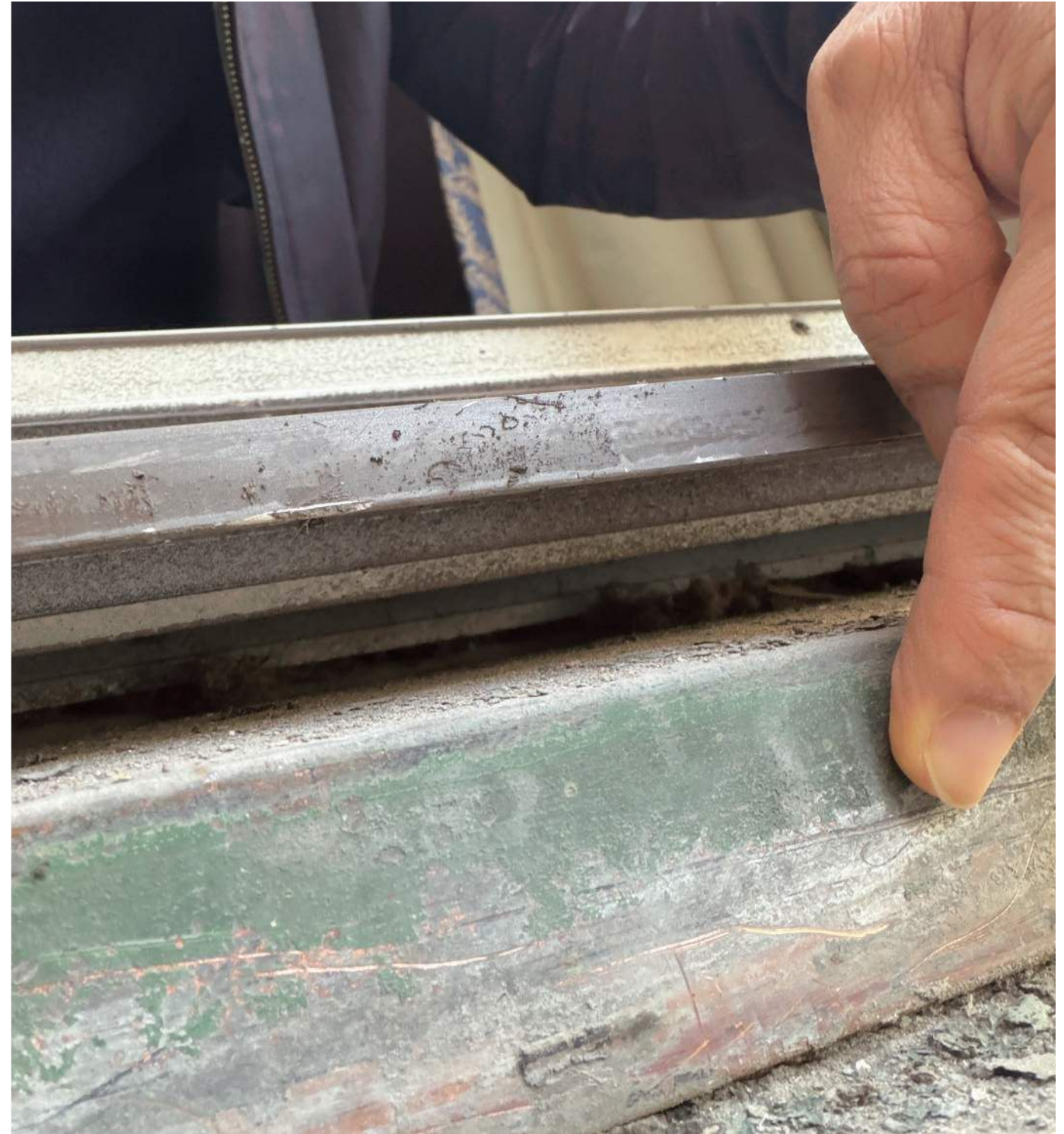
Typ. Exist. Copper Clad Window Sill
