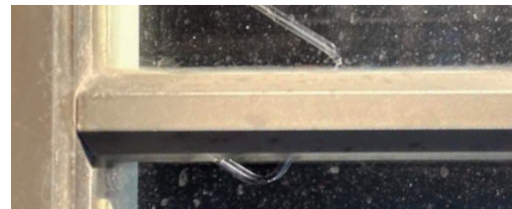
Typical Existing Type A Exterior Muntin
