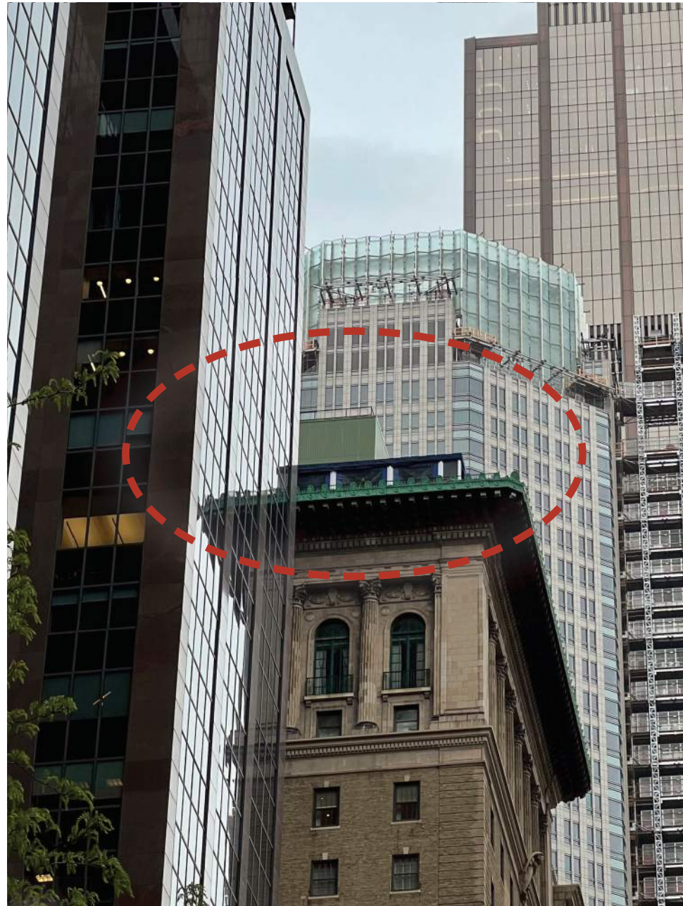
2 Existing Structure is Visible
