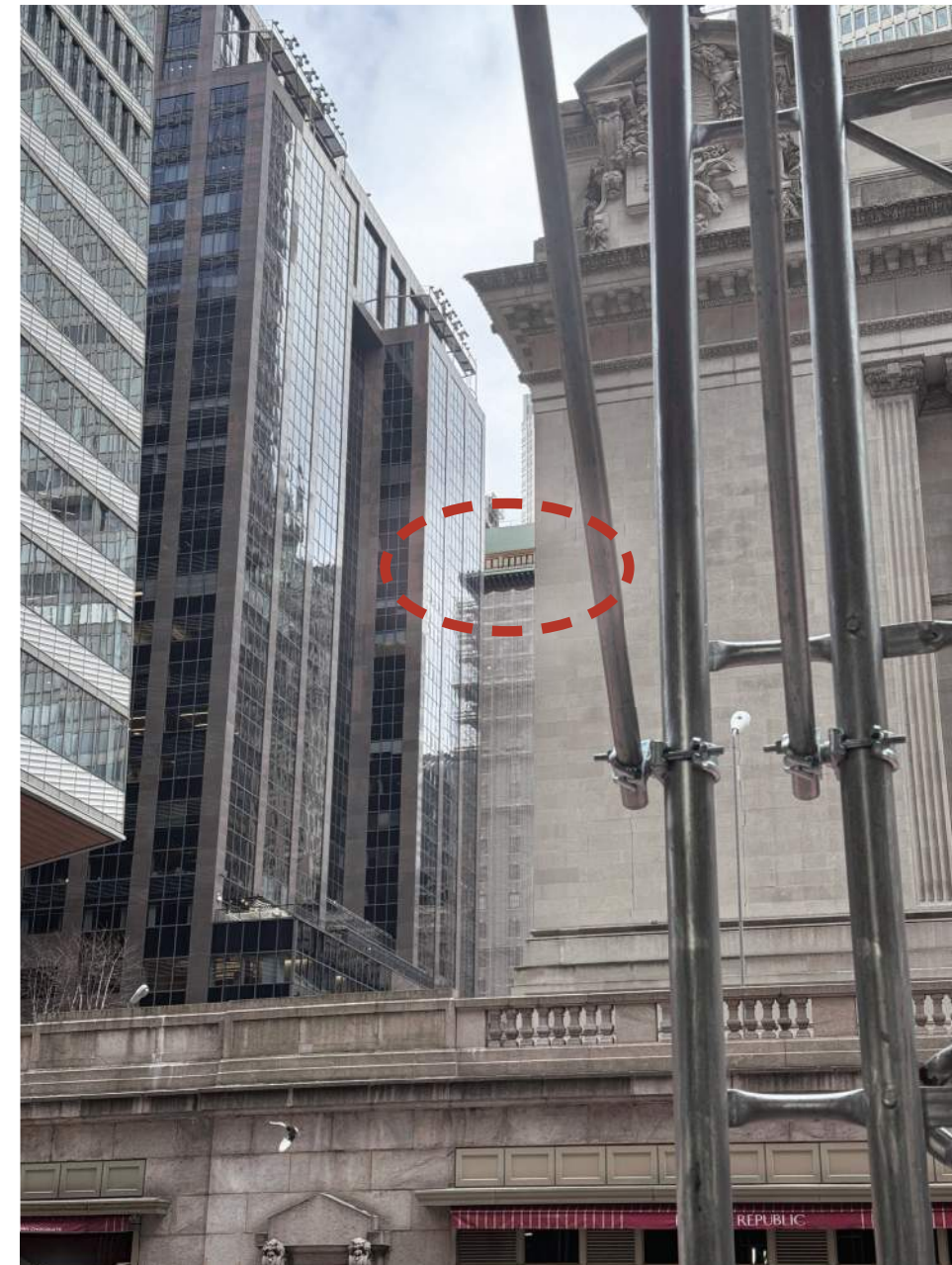
③ Existing Structure is Partially Visible
