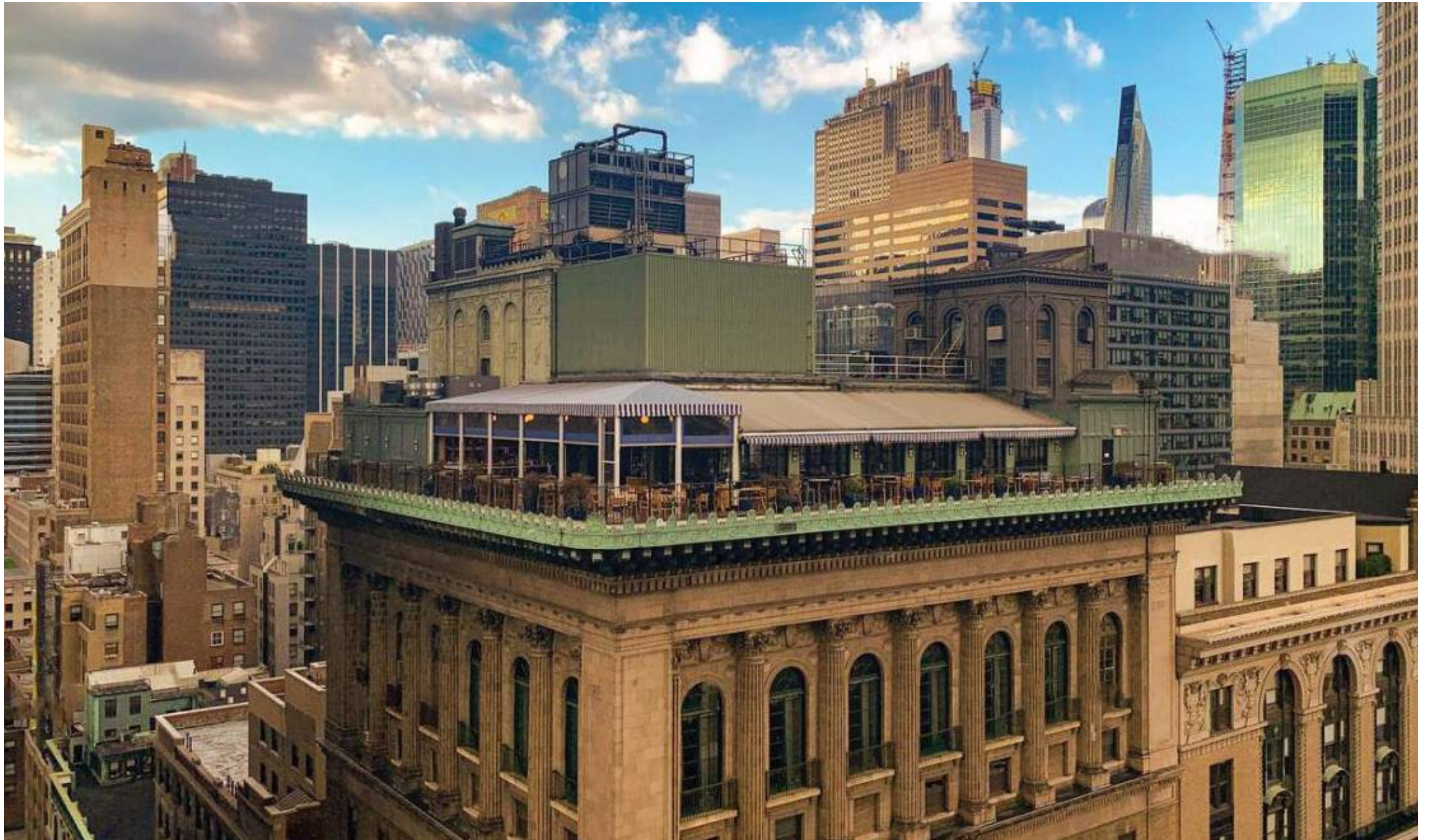
Existing Conditions 22nd Floor – 2019 Photo
