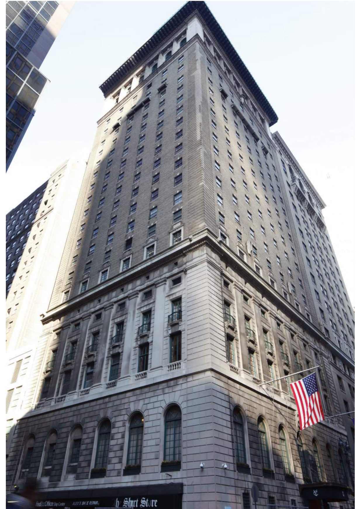
2016 Landmarks Designation Photos
