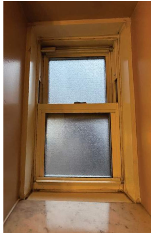
Typical Existing Type B2 Interior
