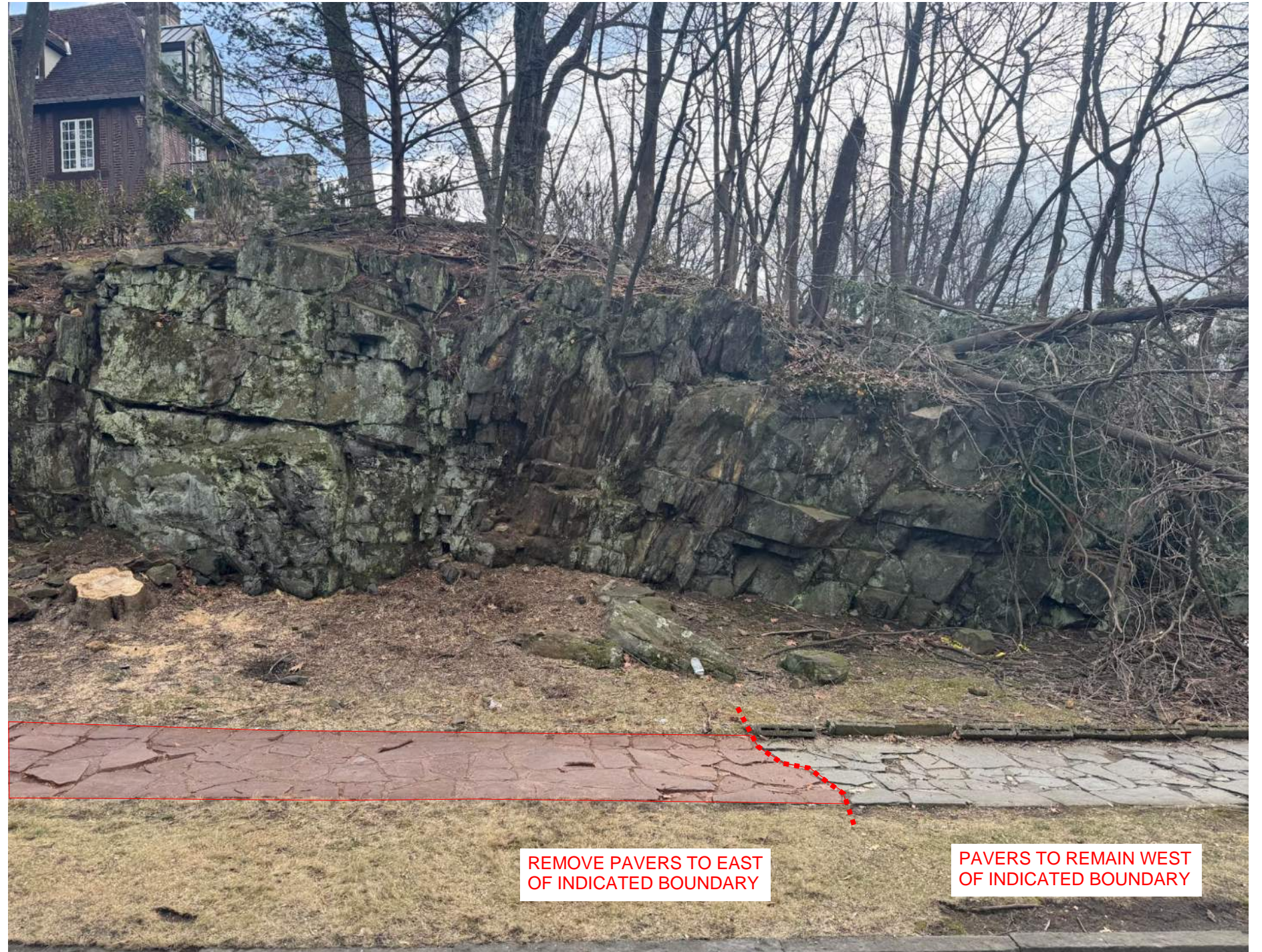
PHOTO 2 – Photo taken on sidewalk of W 246th Street looking south. Red dotted line denoting boundary of sidewalk paver removal. In line with extent of neighboring property's (412 W 246th St) precast curb.
