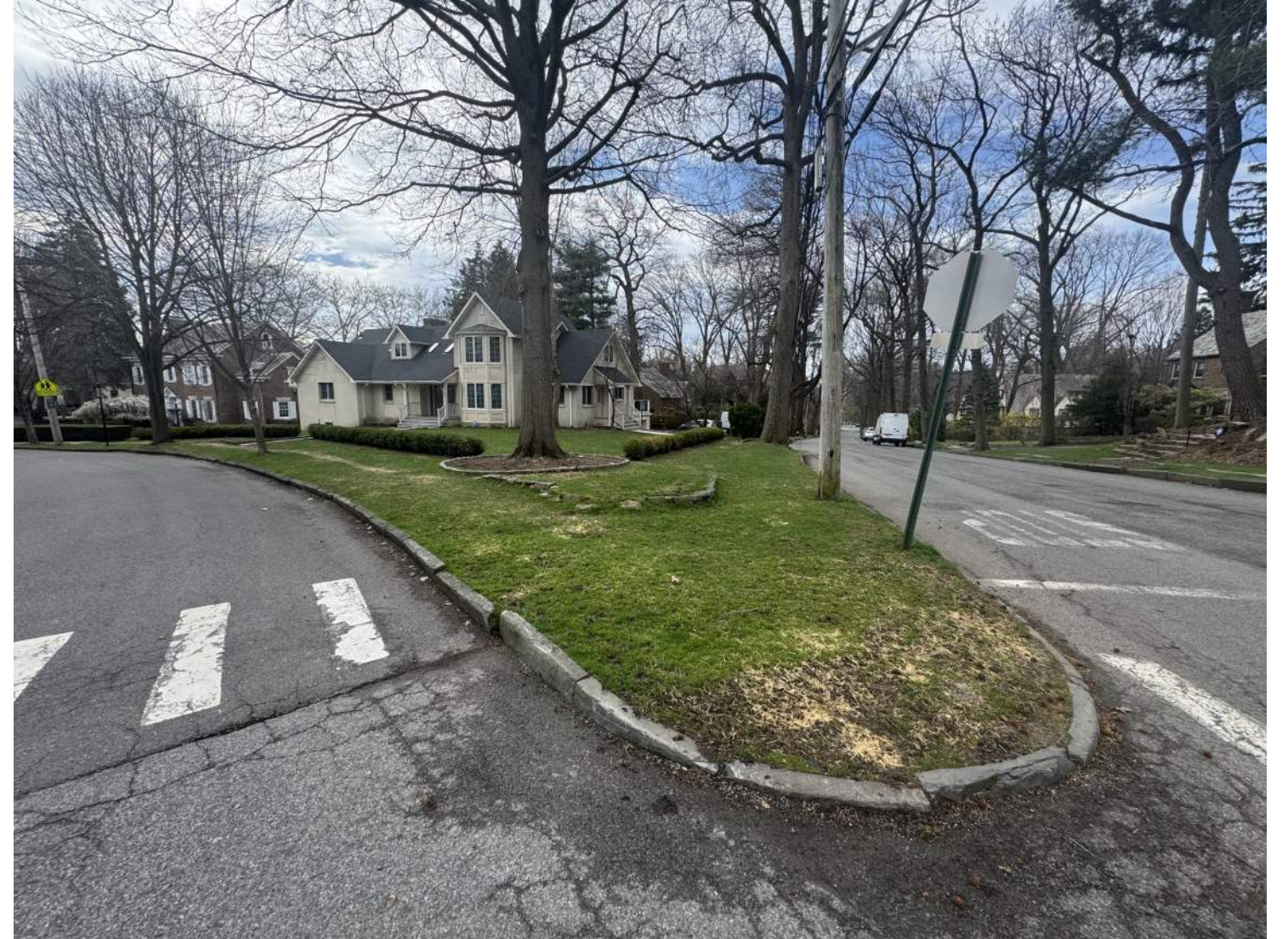
PHOTO 8 – Photo taken on the southeast corner of Waldo Ave and W 246th St looking southeast. Property along sidewalk is 4530 Waldo Avenue, Bronx, NY 10471 (Bronx Block 5807 Lot 643) *photo location not on photo key
