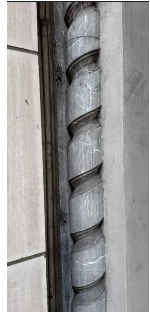
RESTORED ROPING DETAIL ON FIFTH AVENUE S CORNER
