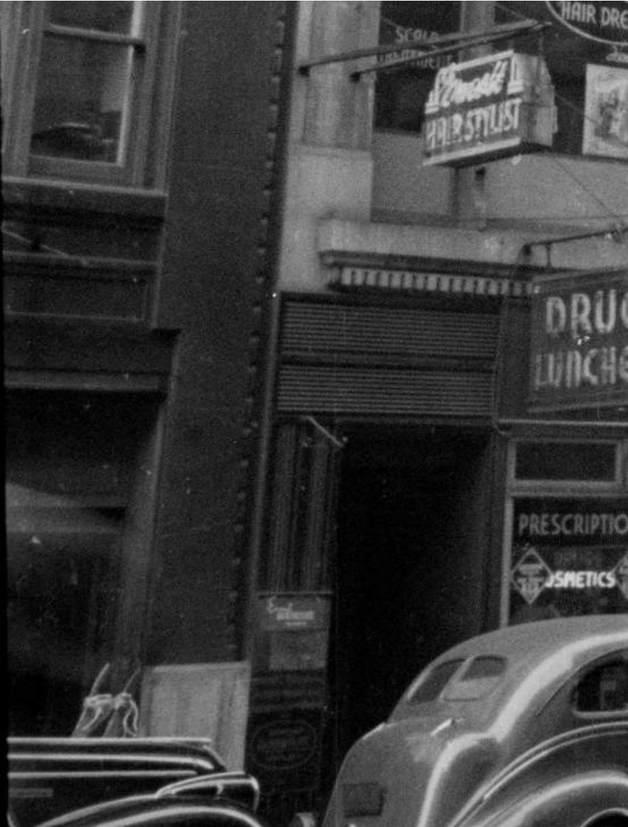
BUILDING CORNER WITH ROPING AT WEST ENTRANCE ON 37TH ST
