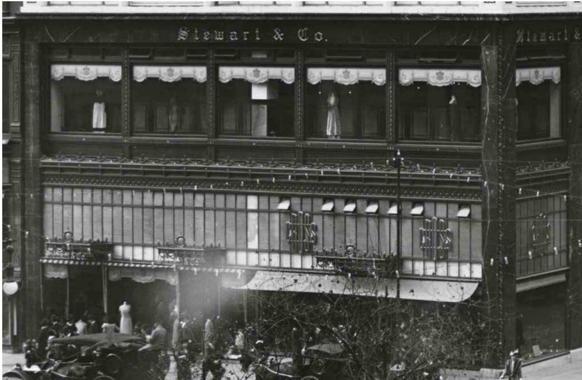
41 CLERESTORY BAYS ACROSS FACADE SQUARE TOP TRANSOM AND BOTTOM APPX 1:3:1 PROPORTION
