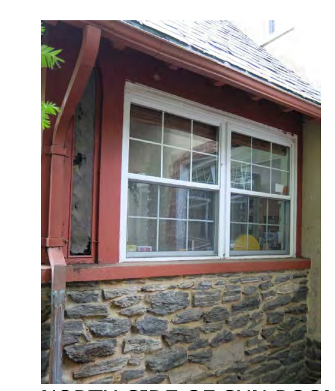
NORTH SIDE OF SUN ROOM
