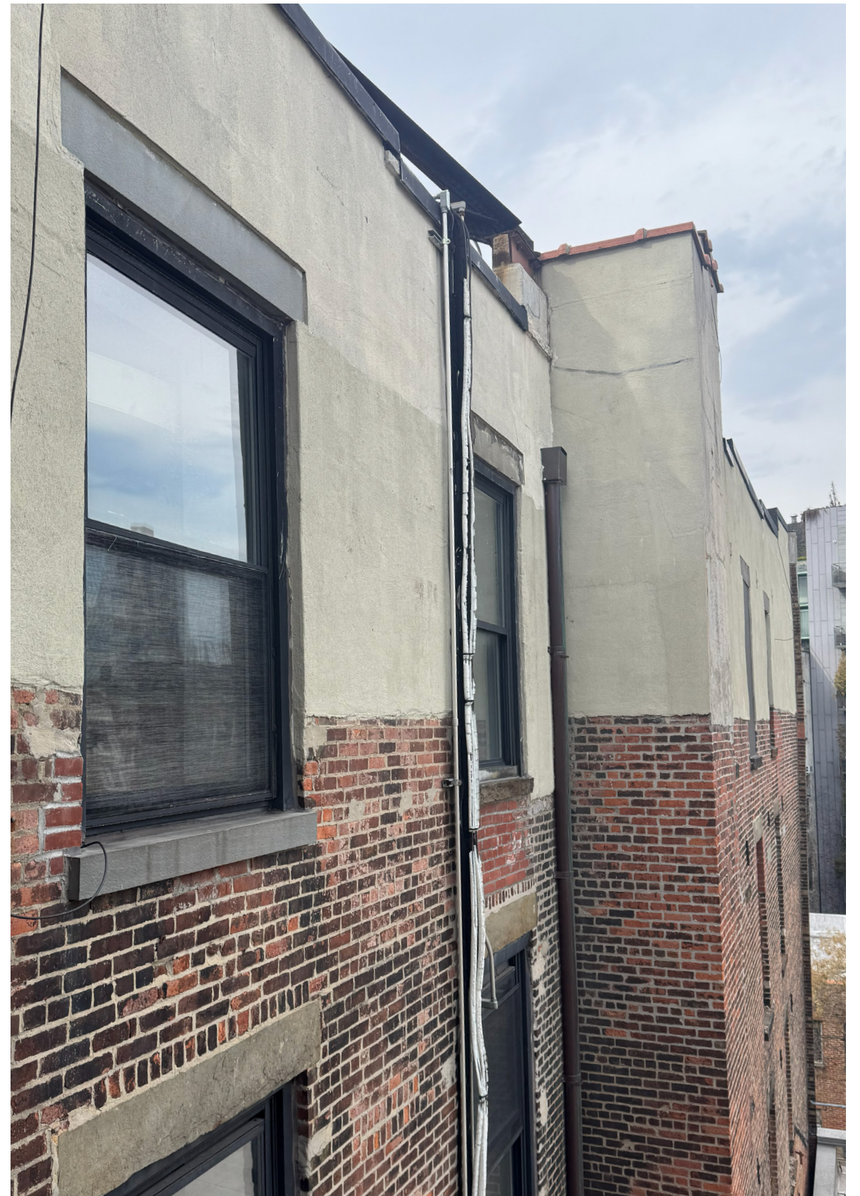
Upper Floor of East Side Elevation
