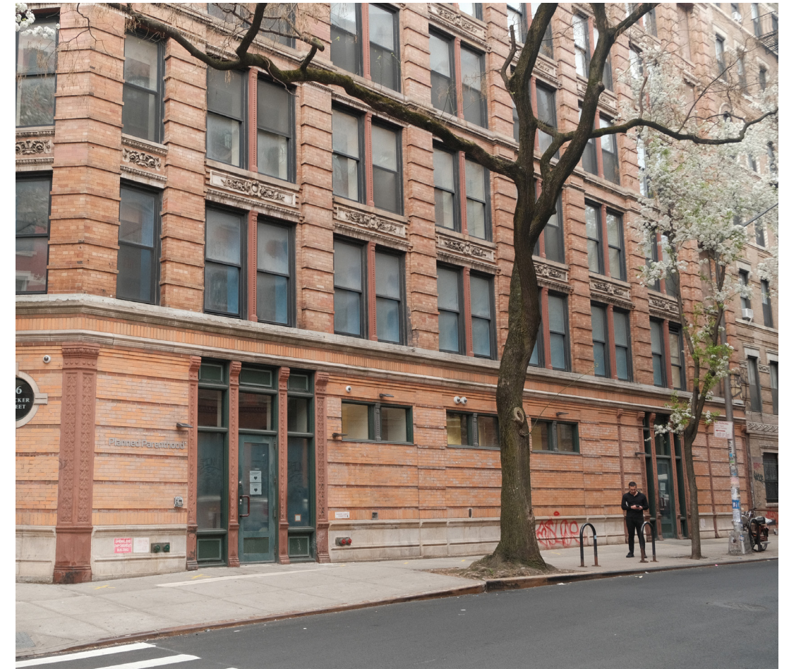
Mott Street Elevation, facing southeast
