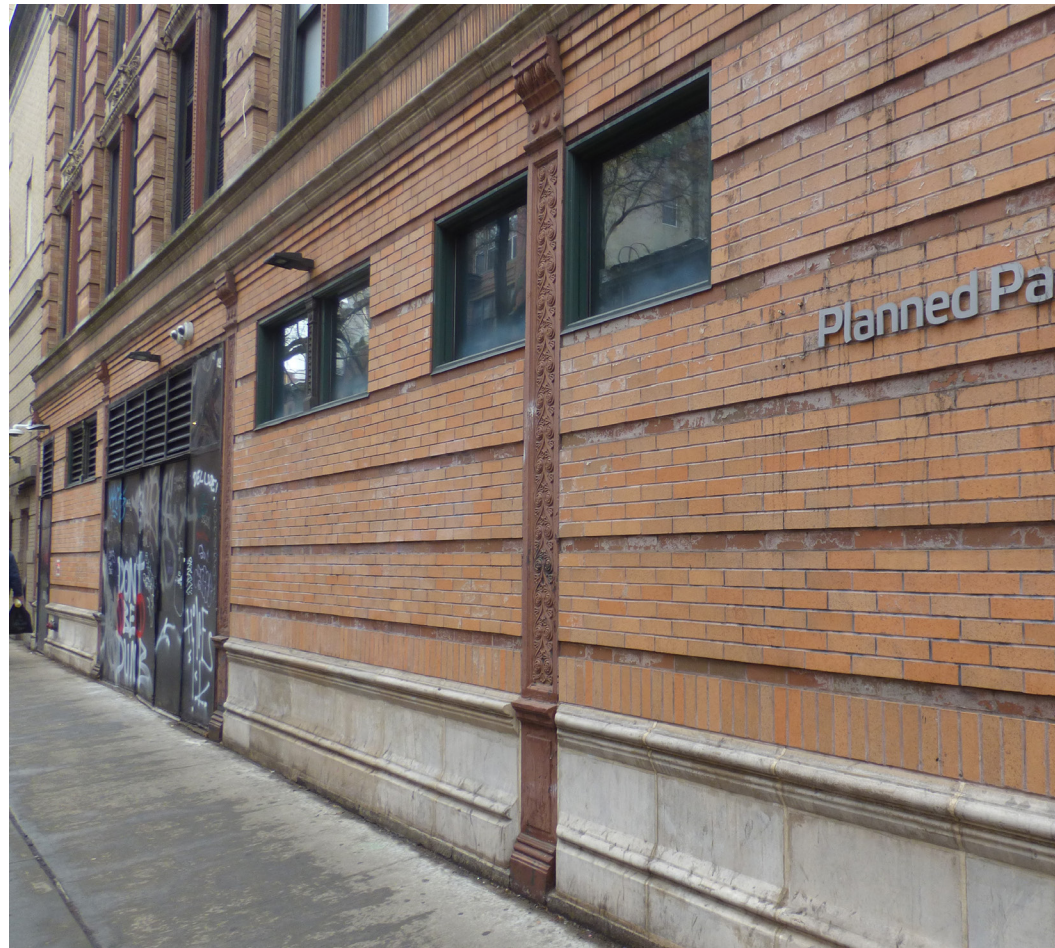
Bleecker Elevation, facing east
