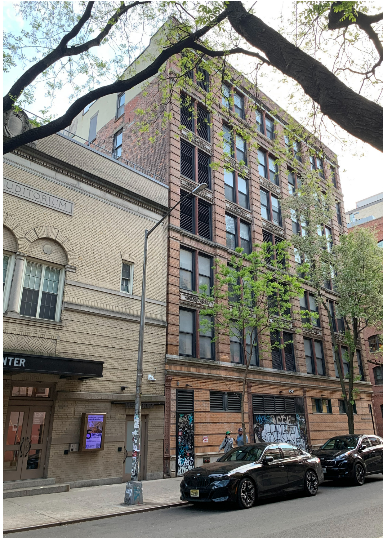
Blecker Street Facade, Facing South, 2026
