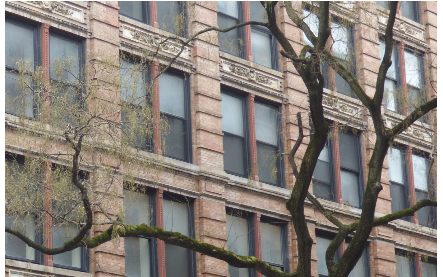
Window Details, Mott Street facade
