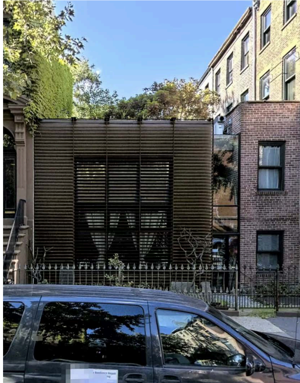
228 Washington Ave: Backyard extension visible from the street
